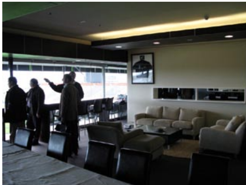
AMI corporate box: Ply bulkhead at doors bulkheads, suspended ply bulkhead with recessed down lighting and uplighting and plaster board ceiling. Mirror backed joinery unit semi recessed. Plaster board walls paint finished with 40mm anodised aluminium skirting
