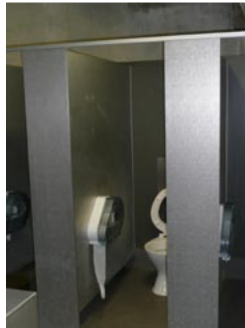
AMI GA Toilets: Toilet partitioning rigidised (textured) stainless steel in aluminium frame. Floor mounted pans with flush valves. No ceilings.
