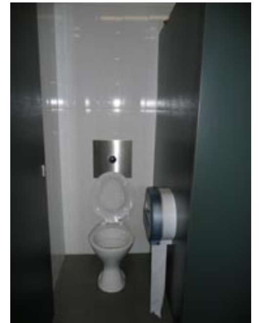
AMI Corporate Toilets: Compact laminate partitions, tiled walls to door height, SS flush plate with sensor.
