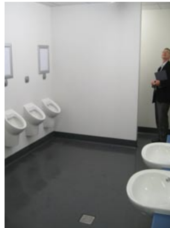
Westpac Corporate Toilets: Wall hung urinals with electronic flush valves. Vinyl floor and skirting. Plaster board walls. Suspended gib ceiling. Semi-re- cessed basins with single lever mixers on HPL top.
