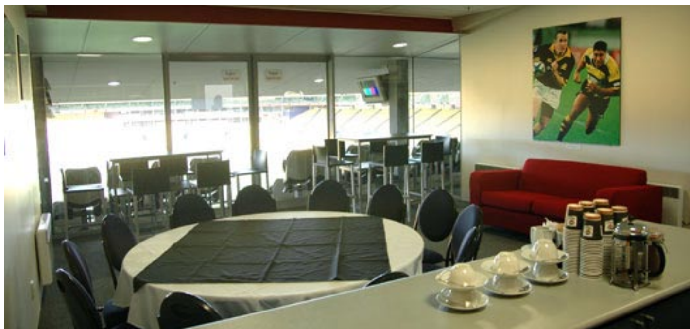
Westpac corporate box: Plaster board bulkhead at doors with recessed down lighting. Wall mounted heaters. Plaster board walls paint finished. Bowl glazing framed bi-parting sliding doors in aluminium frames to side lites, frameless glass returns.
