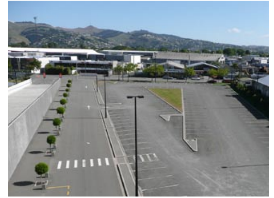
AMI Landscaping: Asphalt car-park, planted grass edges, concrete pavers to foot paths. Lighting via masts
