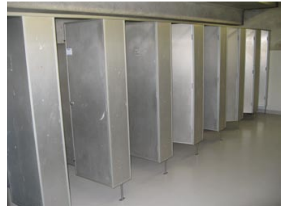
Westpac GA Toilets: Toilet partitioning rigidised (textured) stainless steel in aluminium frame. No ceilings.
