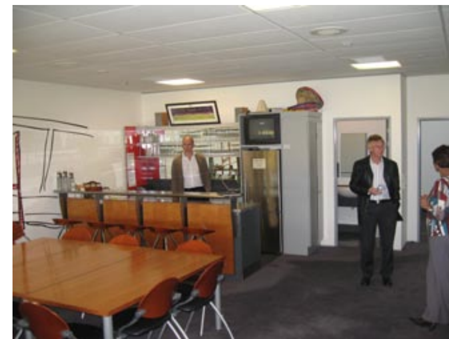
Westpac corporate box: Suspended tile ceiling with recessed fluorescent fittings. Carpeted floor in broadloom. Joinery unit in LPL with cupboard unit and fridge. Back bar with open shelving and mirror back. Larger boxes (pictured) have servery bar with timber veneer fronts and laminate top.
