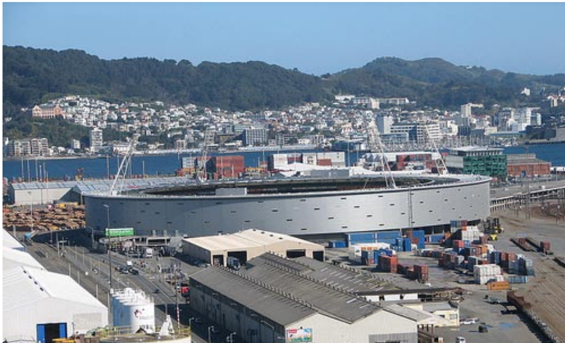
Westpac Exterior: Profiled metal run horizontally with windows set out in spaced pattern. Roof overhang at eaves separated from facade by continuous clerestory glazing detail.
