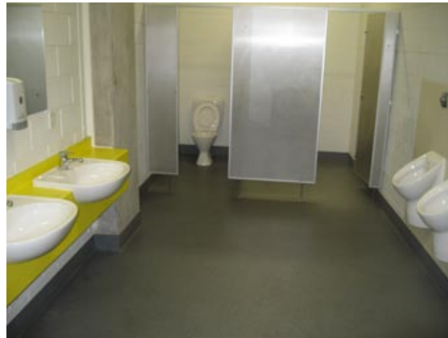
Westpac Players Change: Toilets painted block walls, rigidised SS laminate partitions. Individual urinals, semi recessed basins with single lever mixers on HPL unit. Waterproof flooring
