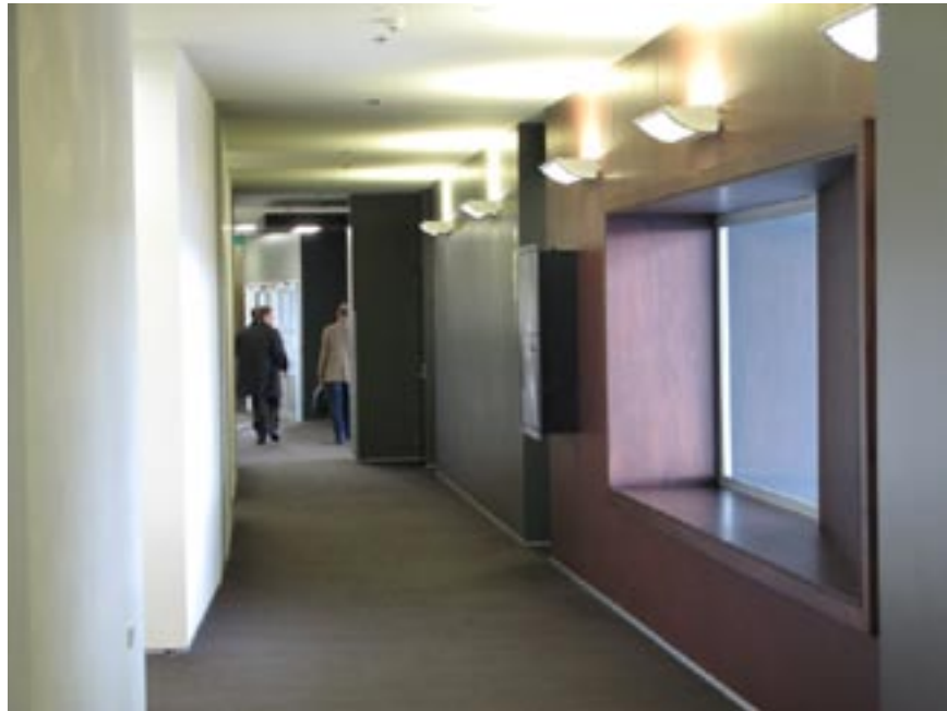
AMI corporate corridor: Ply jamb liners and solid timber architraves to feature window boxes. Broadloom carpet
