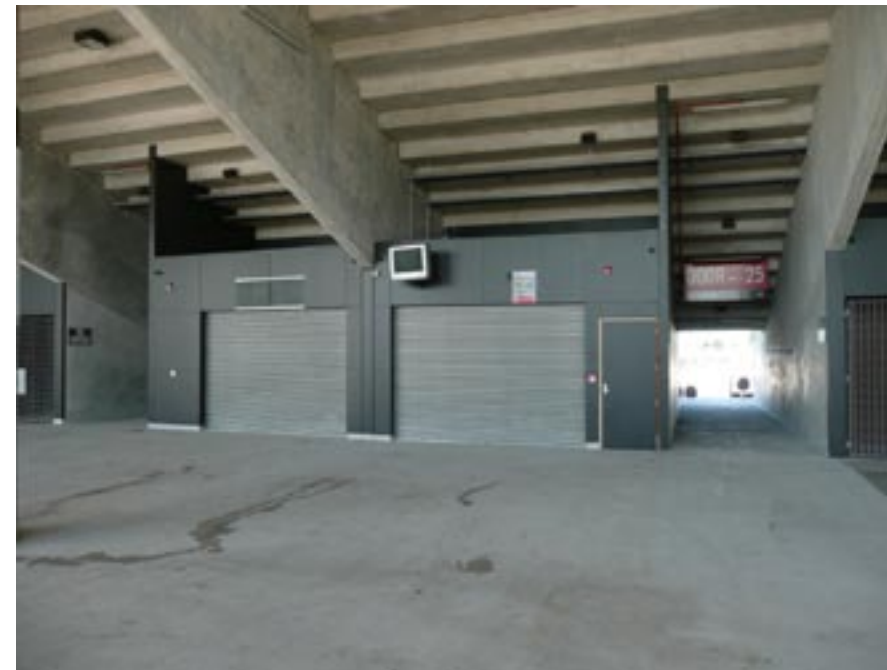
AMI GA Concourse L2: Exposed concrete structure, painted toilet and F&B facilities. Facing walls fibre cement sheet, flanking vomitory walls full height painted pre-cast. Vomitory entrances sprinkler protected.
