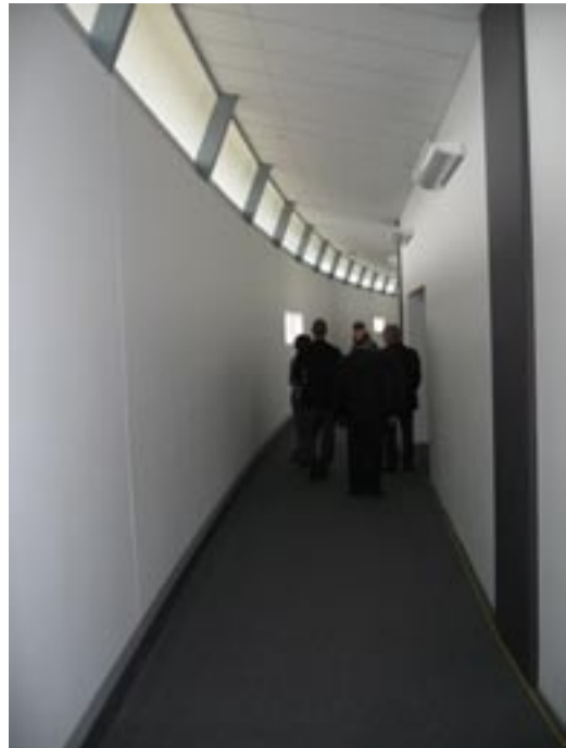
Westpac corporate corridor: Plaster board walls, sloping tiled ceiling. Wall mounted up lighters. Feature clerestory glazing with intermittent punched windows. Broadloom carpet.
