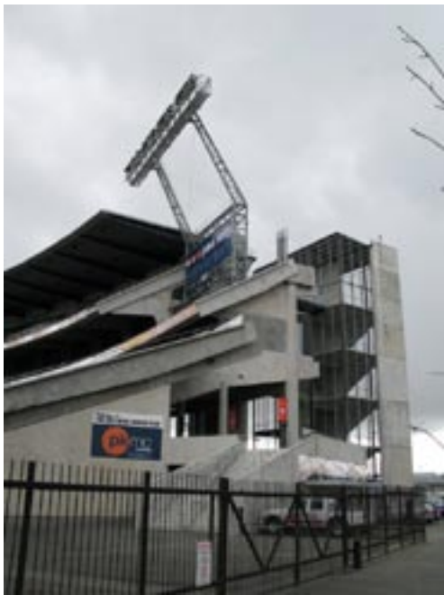
AMI Fences: Metal posts with 3 horizontal railings and verticals with intermediate braced panels.
