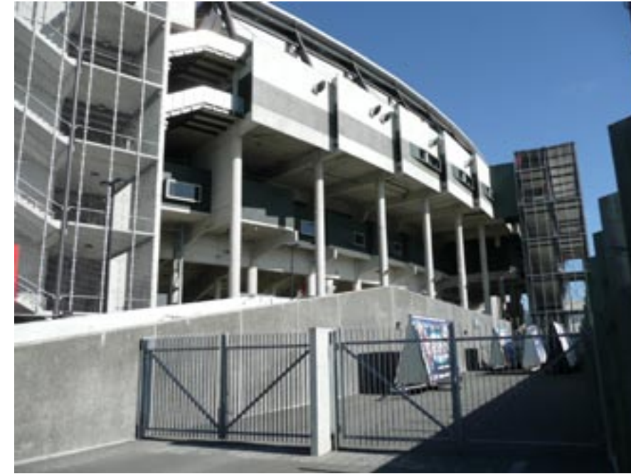
AMI Exterior: Articulated facade, large overhangs, stepped plan. Mixture of fibre cement sheet and pre-cast concrete cladding elements. Galv metal sheet and galv square reinforcing mesh barriers
