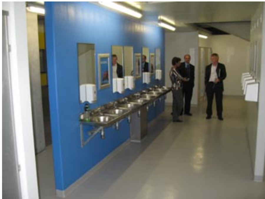
Westpac GA Toilets: Painted pre-cast wall, SS basins in grouping with SS bottle traps and solenoid taps. Central services point, Ceiling over basins and hand driers area, surface mounted fluorescent fittings. Sealed epoxy floor and skirting
