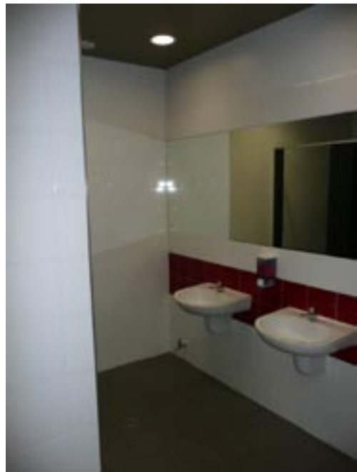
AMI Corporate Toilets: Tiled walls up to door height, painted walls above. Floor tiled. Basins wall mounted with shrouded wastes. Painted plaster board ceilings with recessed down lights
