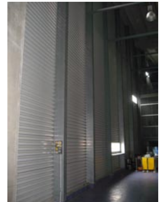
Westpac GA Concourse: Inside face of exterior walls unlined
