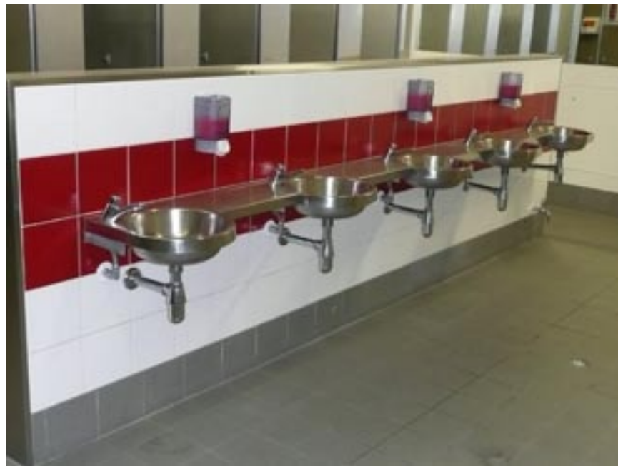
AMI GA Toilets: Half height tiled wall, SS basins in grouping with SS bottle traps and solenoid taps.
