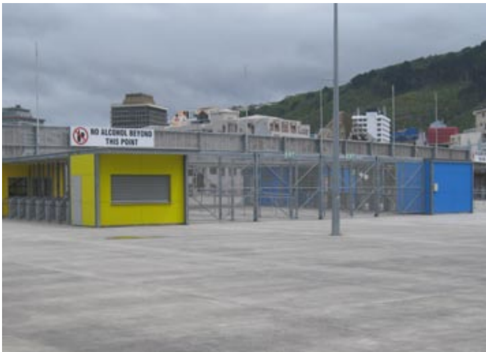
Westpac Fences: Large galv metal gates with intermediate braced panels.
