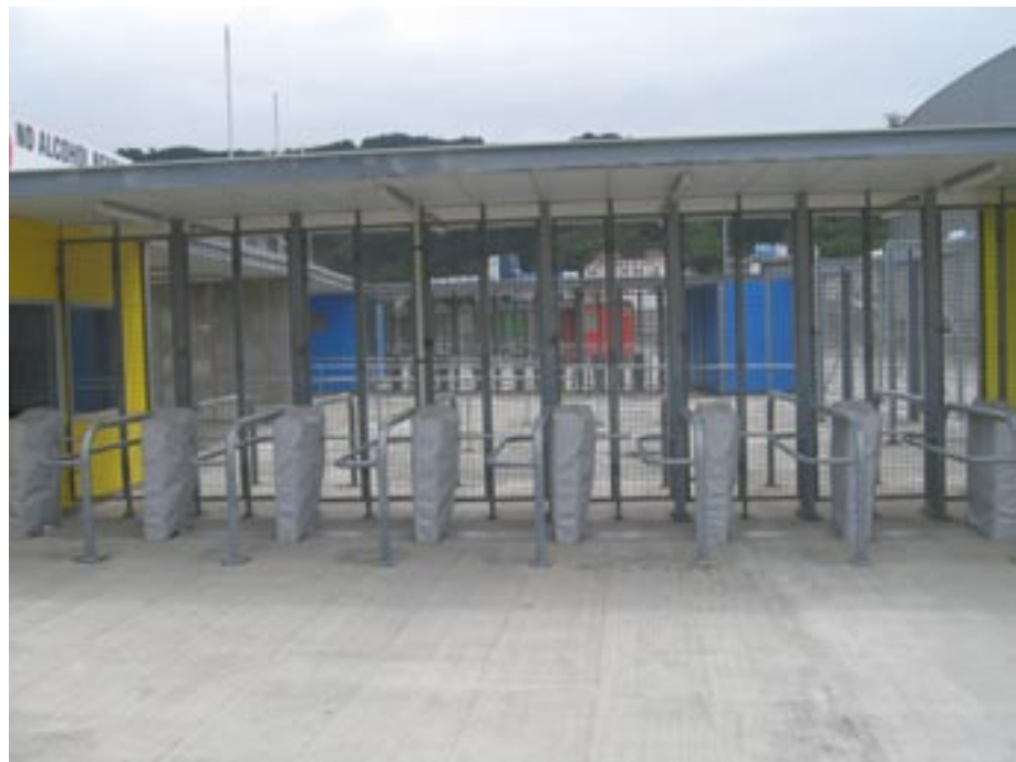
Westpac Gates: Purpose made galv frames with larger RHS intermediate posts, square galv mesh infill.
