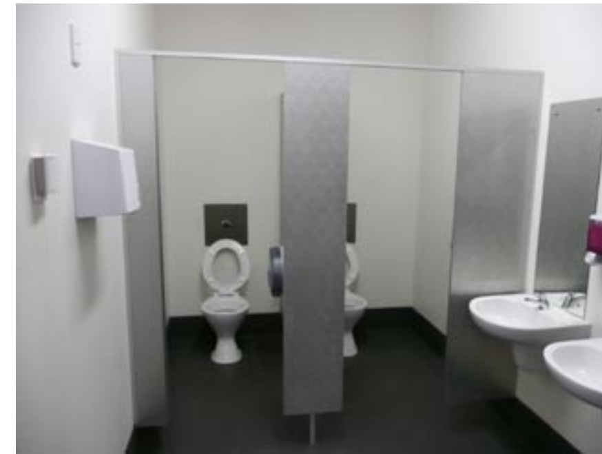
AMI Players Change: Toilets painted plaster board walls, rigidised SS laminate partitions. Shared wet area with partitions and slider. Waterproof vinyl flooring
