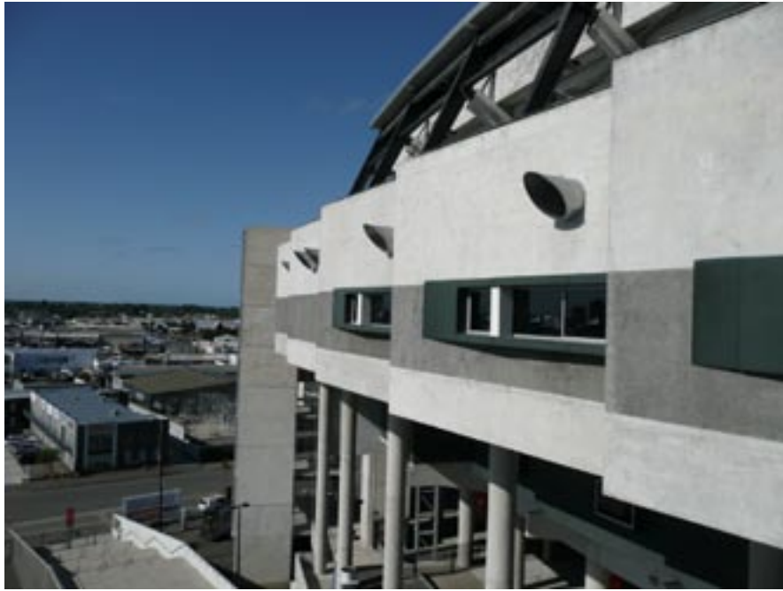
AMI Exterior: Exposed concrete structure, pre-cast concrete panels smooth faced with exposed aggregate feature panels. Exposed stair tower with pre-cast and galv mesh walls and metal roof. Fibre cement facing details to horizontal strip windows
