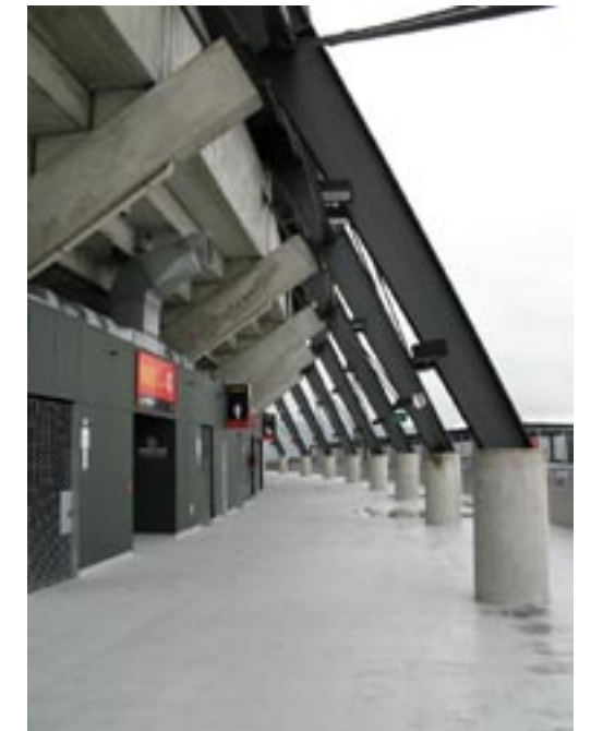
AMI GA Concourse L5: Slab waterproofed with applied membrane
