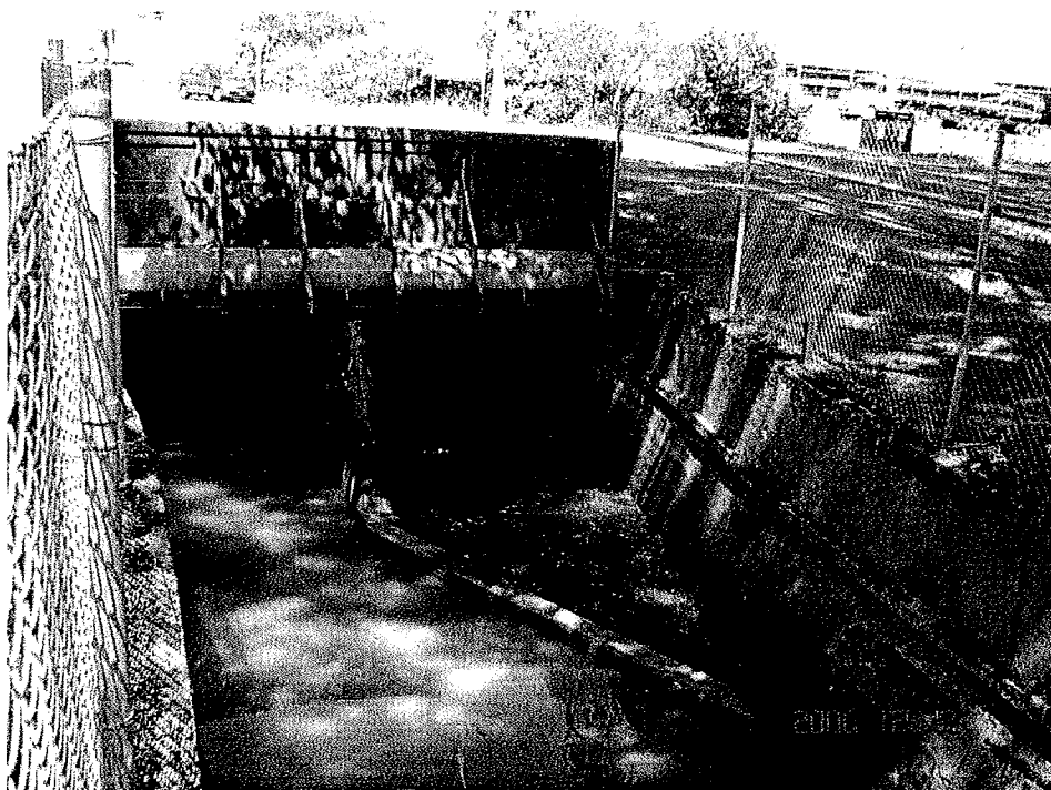
Figure 3.3: Photo of entrance to Opoho Creek culvert upstream of Ravensbourne Rd. Concrete wall level on right at ~RL102.6m
