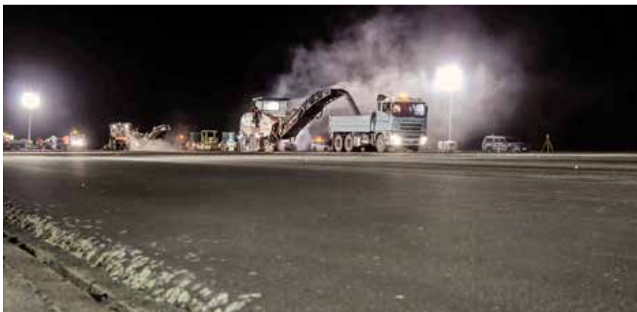
Dunedin International Airport resealed its runway with Echelon paving during non-operational hours. The project took 23 nights with minimal disruption to services.
