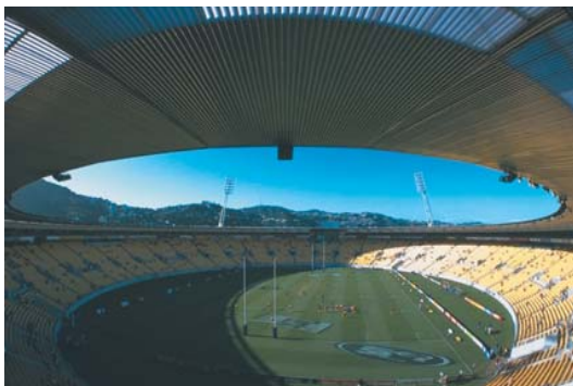
Fig 2.3.8.C Westpac Stadium, NZ Heavy shadow to light zones can cause lens flare in transition.
