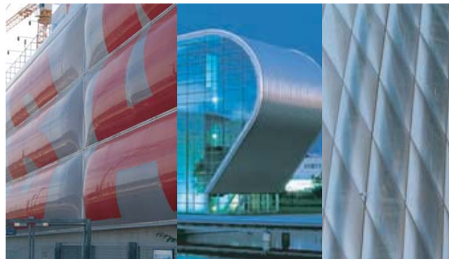
ETFE Cladding Profiled Aluminium ETFE Cladding
