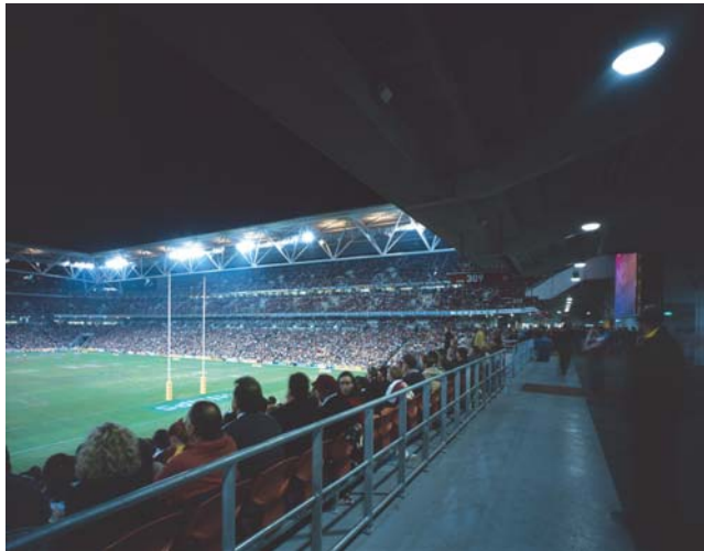
Figure 2.3.4.M Suncorp Stadium GA concourse
