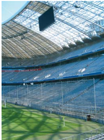
Figure 2.3.4.G Allianz Arena Operable Blinds
