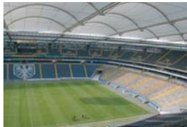
Fig 2.3.8.D Commerzbank Arena, DE light shadows caused by the cables and strong shadows caused by the jumbotrons and PTFE roof canopy. Heavy shadow to light zones can cause lens flare in transition.
