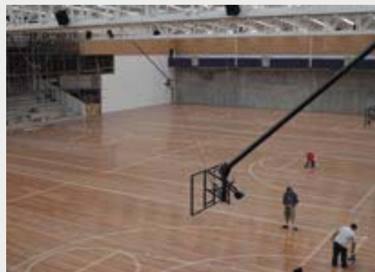
The Edgar Centre Upgrade.
