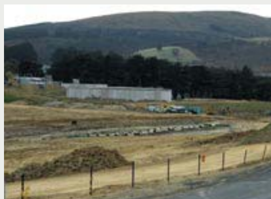
Major work is being undertaken at Mt Grand.
