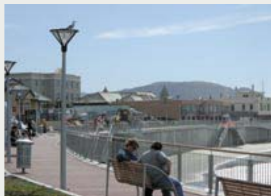
St Clair seawall upgrade is one of many projects progressed during the year.
