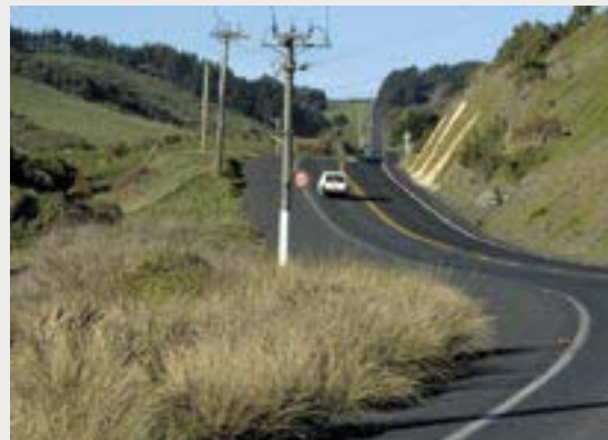
Road resealing and renewing is ongoing.
