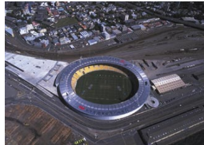
Westpac Stadium, Wellington
