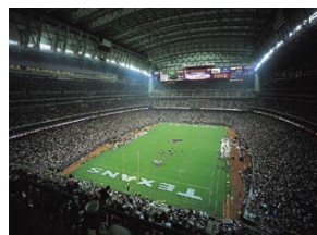
Reliant Stadium, Houston
