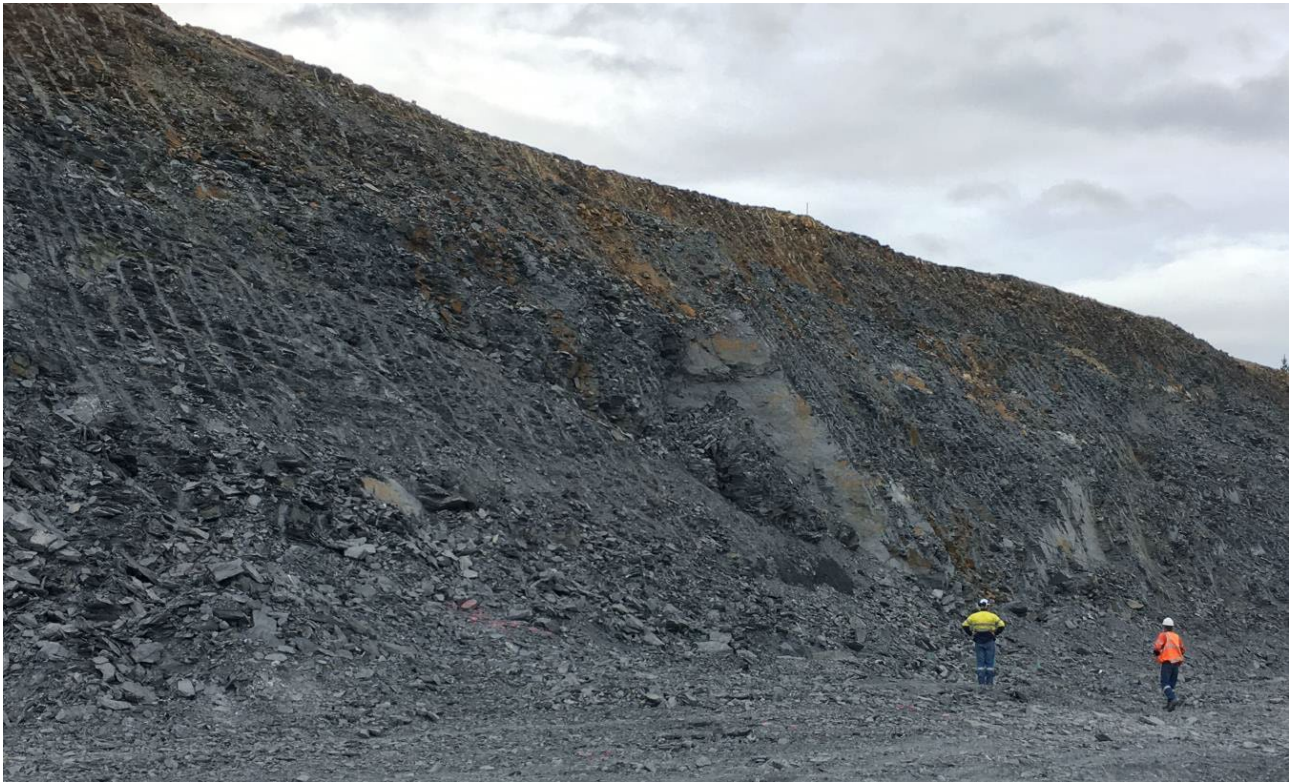
Photo 6: East wall of Coronation Stage 5 pit. The floor is 675 mRL.
