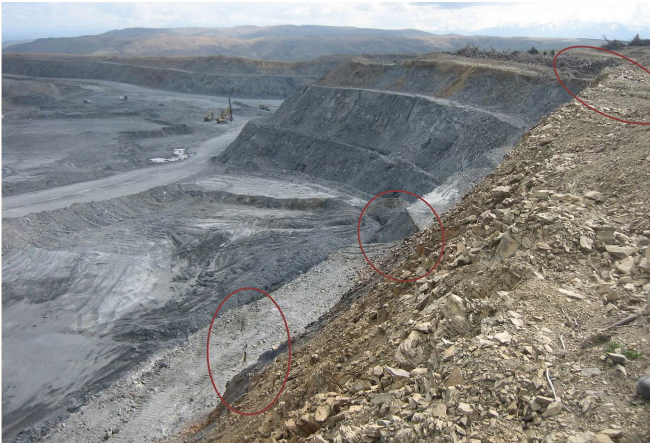
Photo 3: South-eastern wall of Coronation Pit Stage 1. Wedge failures and cracking have formed along north-south trending, westerly dipping faults, 2015.
