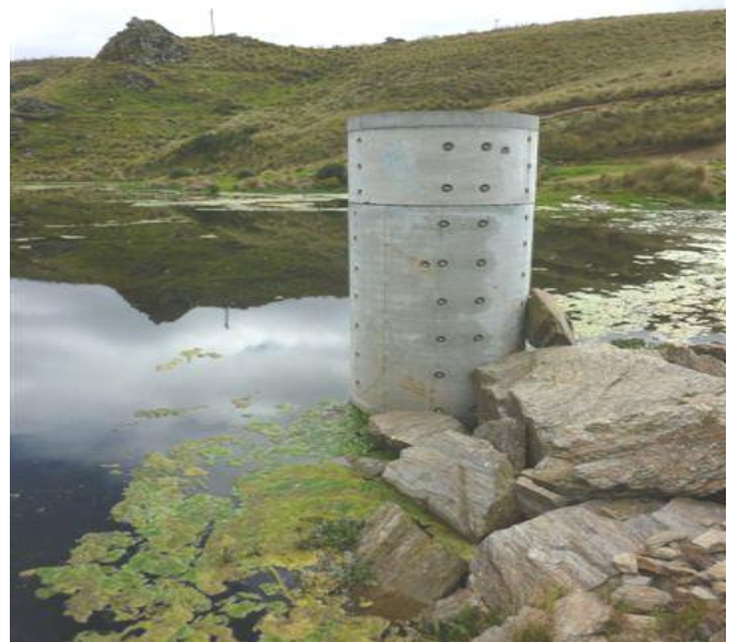
Plate 6. Typical Silt Pond Decant Structure
