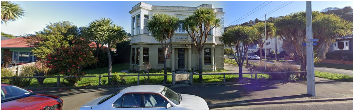
Figure 2: Photograph of the northeastern elevation from Beach Street (Source - Google Maps Sept 2023)
