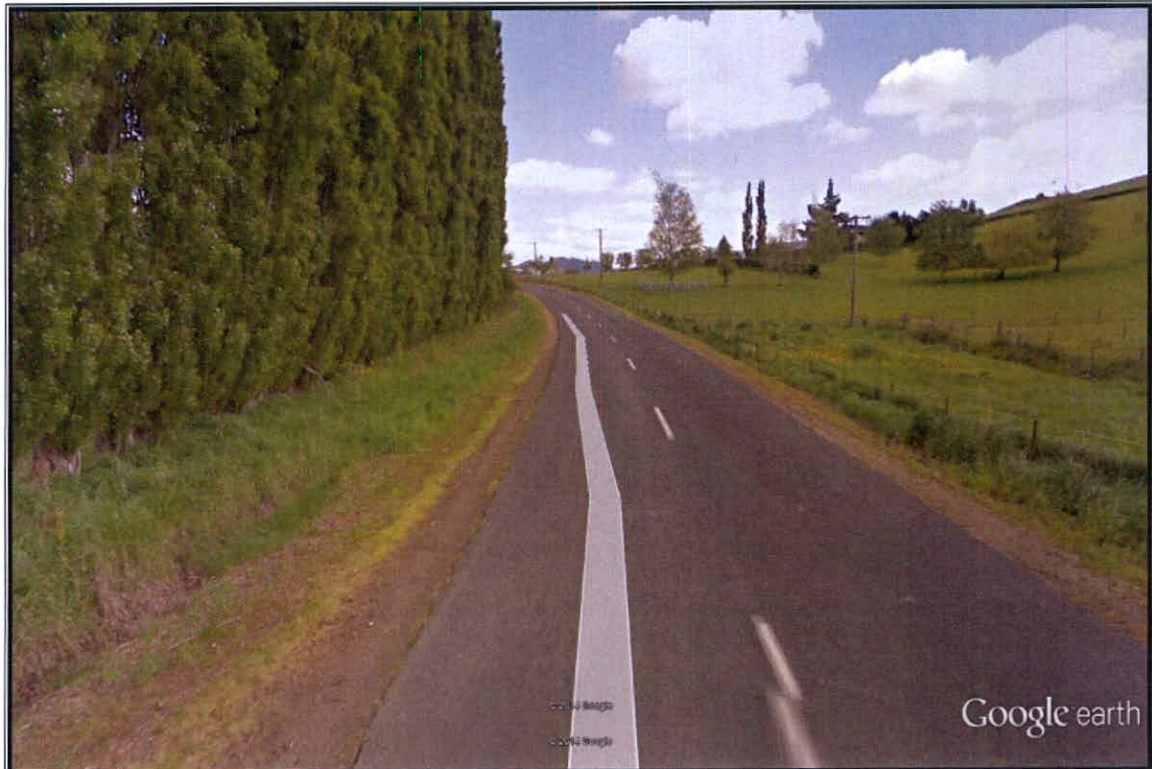
This photo shows the view from the entrance to Lot 2 to the north along Puddle Alley towards the Factory Road intersection – the sight distance here is about 150 metres to the end of the visible part of the curve. (Image date: November 2012)
