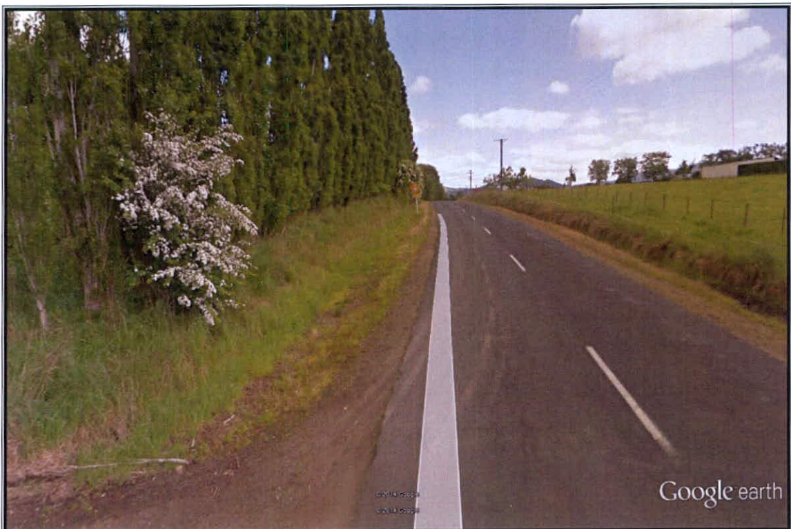
This photo shows the view to the north along Puddle Alley towards the Factory Road intersection – the sight distance here is about 150 metres to the crest of the rise. (Image date: November 2012)
