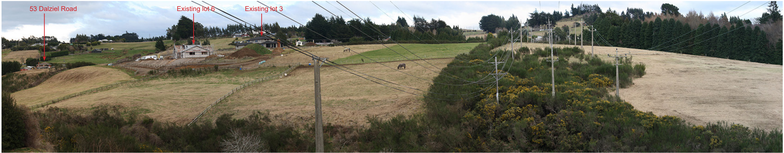
Figure 2 : View of the site from 161 Ashmore Street, Halfway Bush
