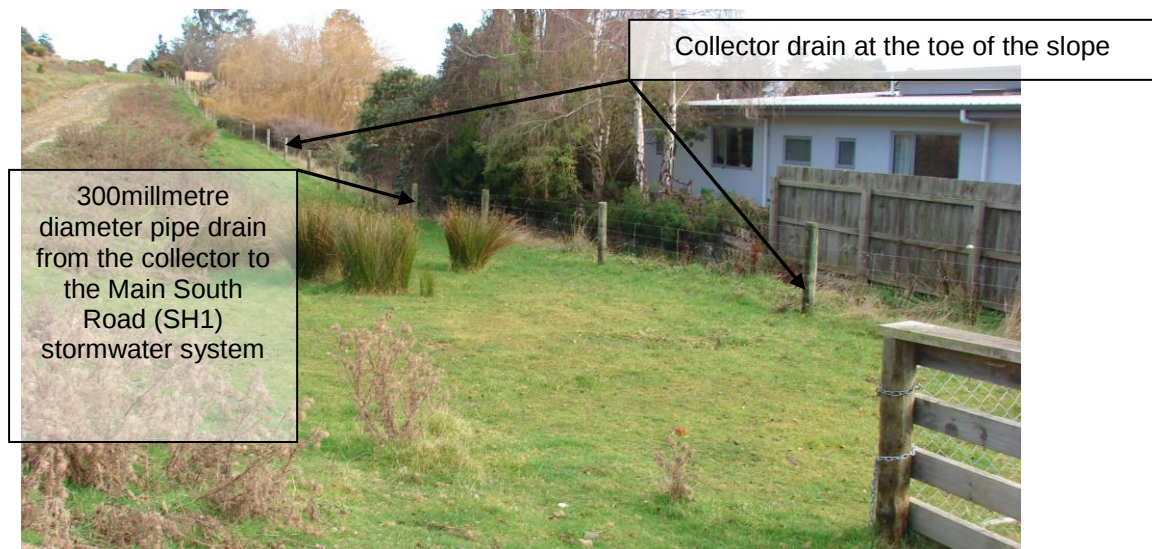
Figure 3: Depression and stormwater discharge locality - northern boundary of Lot 2
