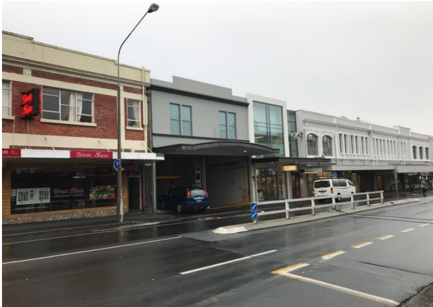
Photograph 1 – Wall Street Mall carpark entrance off St Andrews Street.
