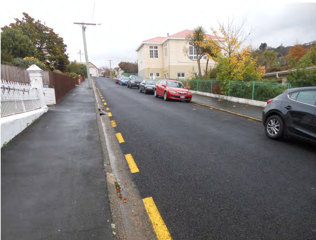
Photograph 2-11: Lomond St – view west
