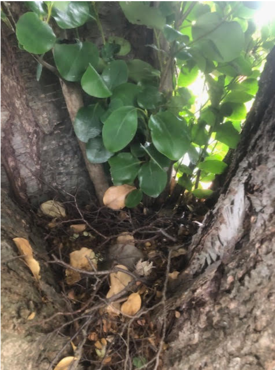
Figure 6 showing the main union where the codominant stems form with debris and a small coprosma growing from the debris
