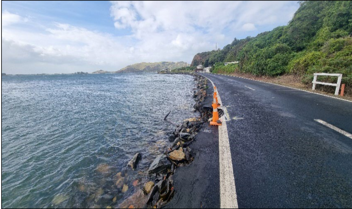
Figure 2 – Ōtākou Wharf section of Harington Point Road is narrow, being undermined and vulnerable to high tides and sea level rise that will shut off the marae and important businesses unless dealt with as a matter of urgency.
