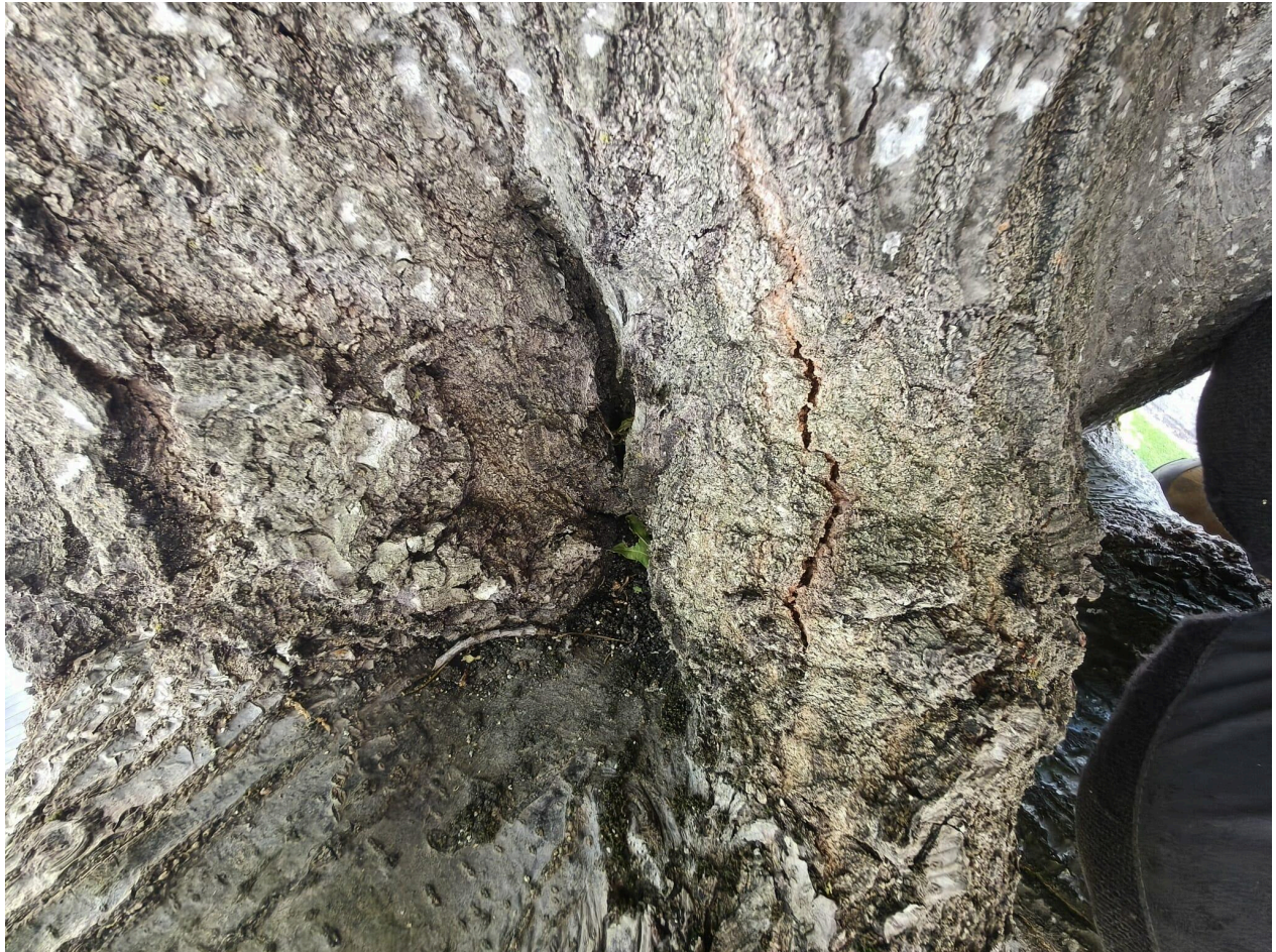
Figure 11.7. A small crack has formed above a limb.
