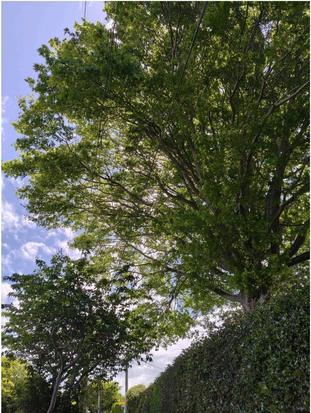
Figure 3. The tree's canopy extends above the power lines, footpath, and road. Although not in this picture the footpath is in between the cherry tree and holly hedge with the road running next to the cherry tree on the western side.
