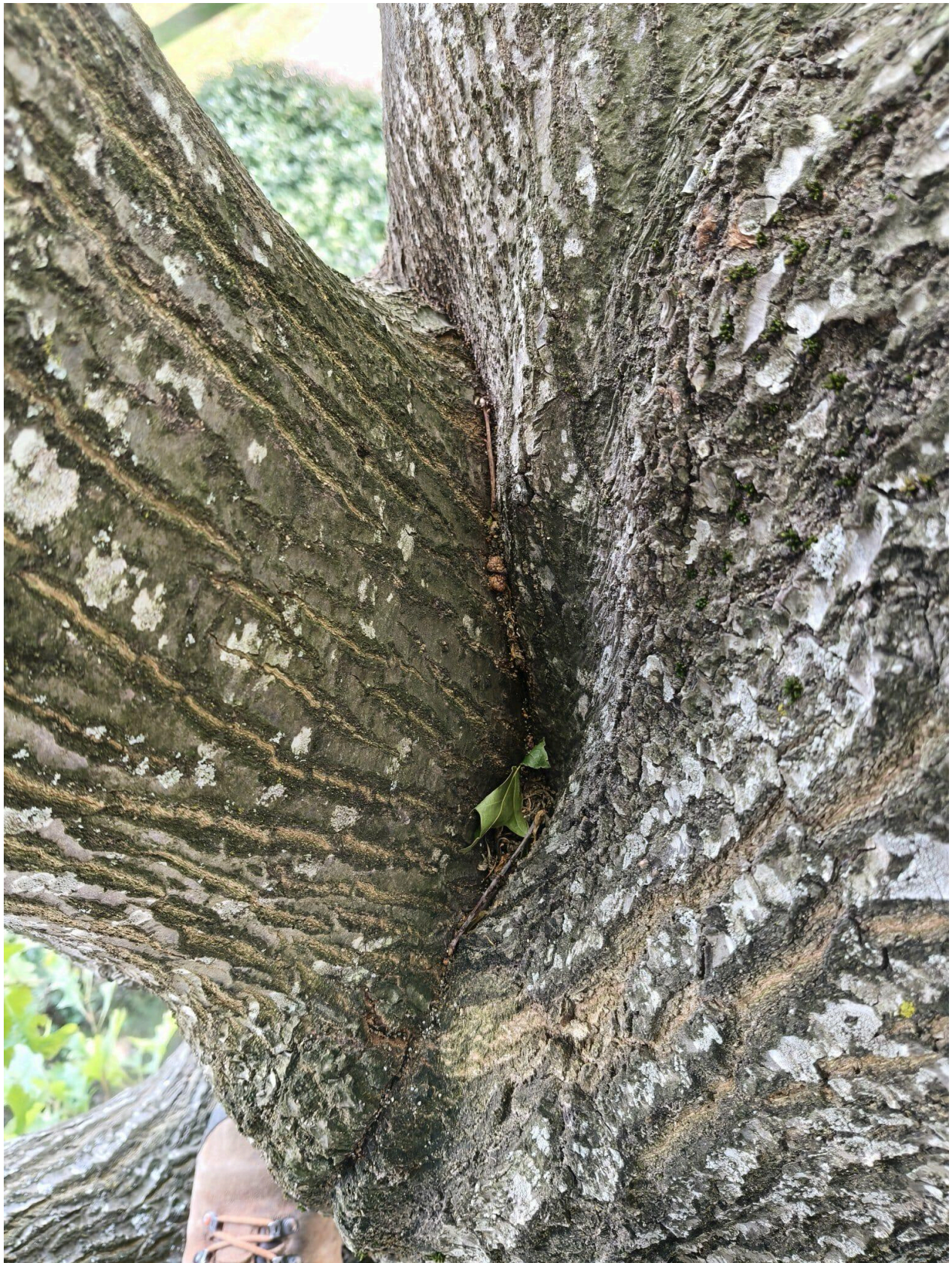
Figure 11.1. Included bark on the limb growing above powerlines.
