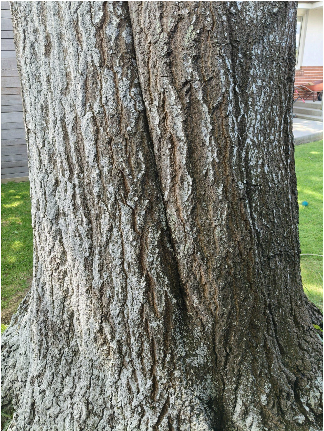
Figure 7. The bottom of the torsional crack.
