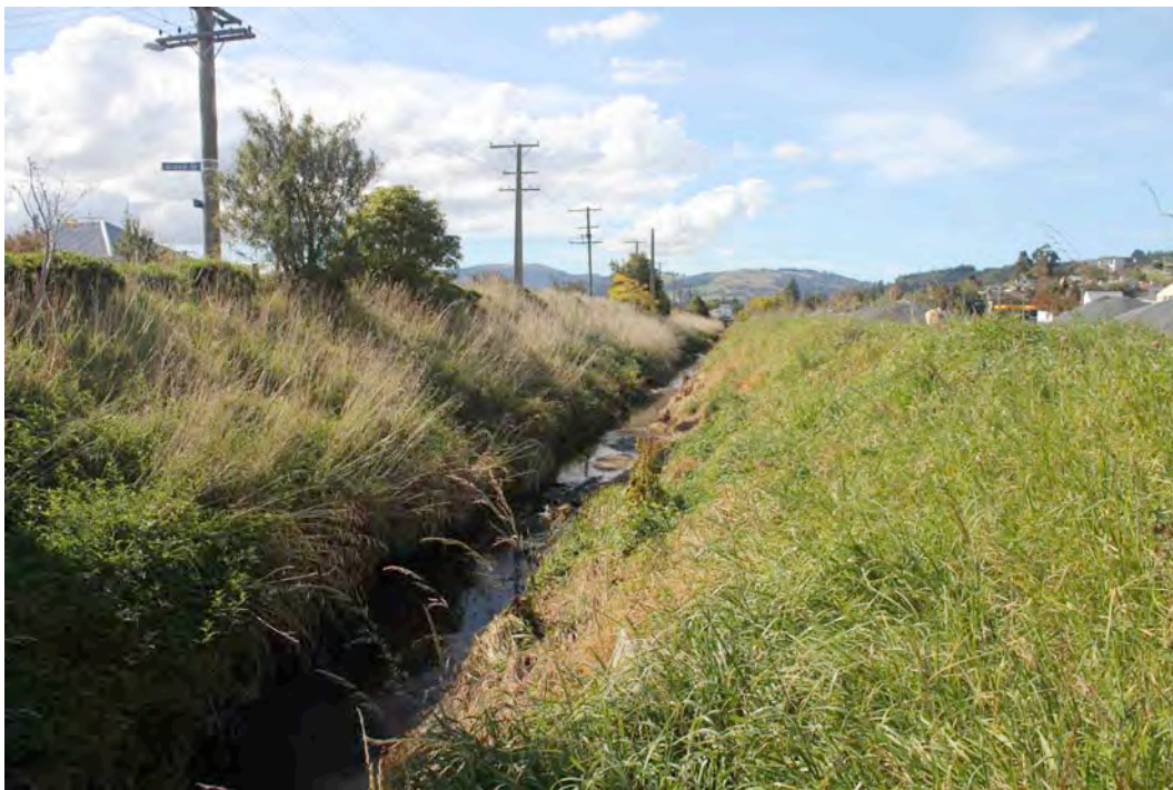
Figure 20 Owhiro Stream at Burns Street, looking upstream.
