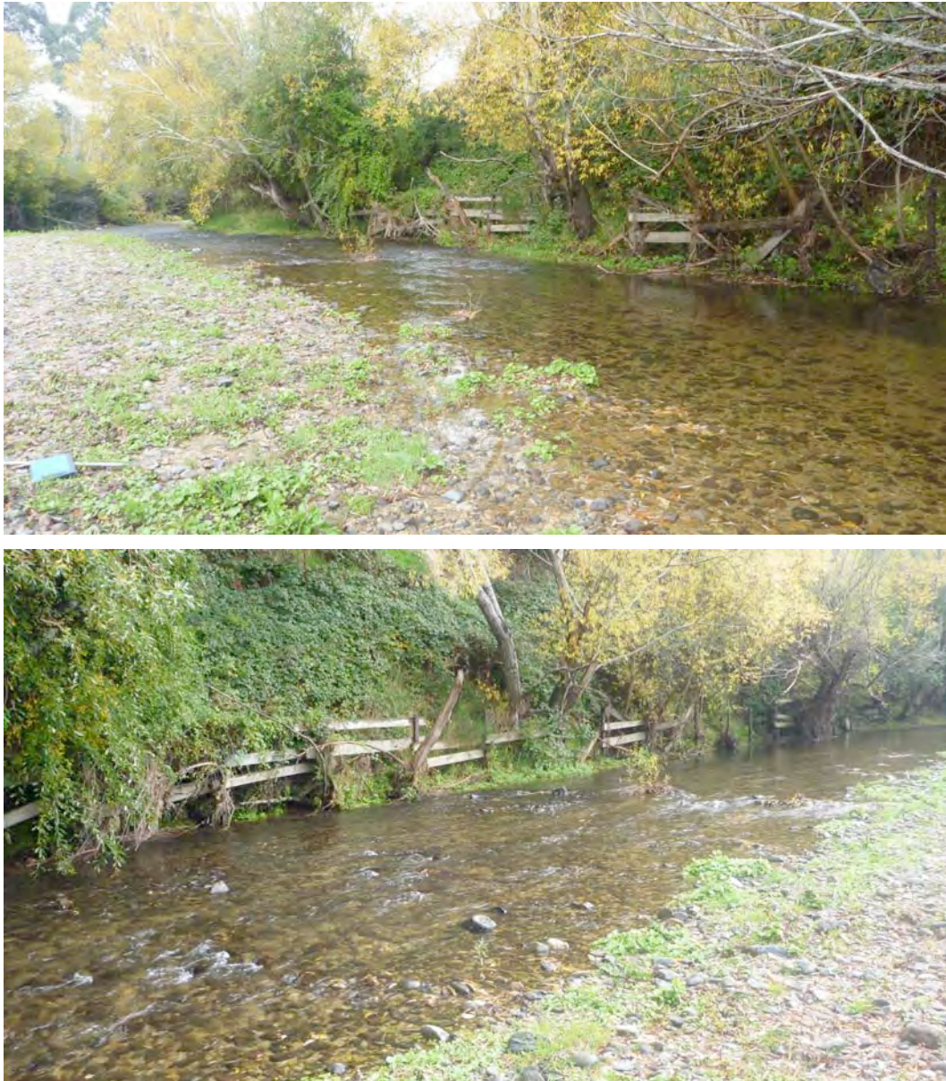
Figure 6 Silver Stream at Puddle Alley. Top: Assessment site, looking downstream. Bottom: Bank reinforcing along the true right bank.
