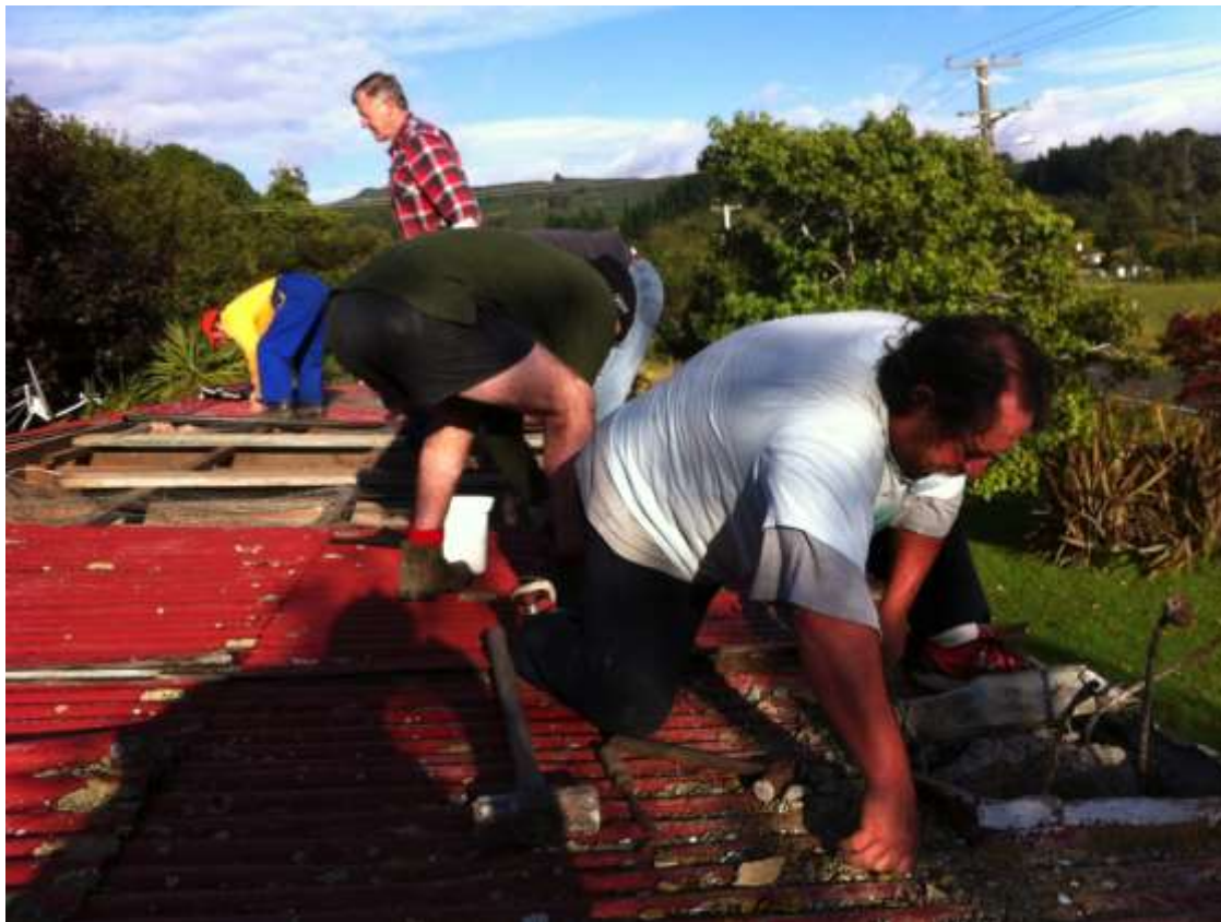
Community Support: 2014 ‘Flash Mob’ to retrofit ceiling insulation in a cold home with high energy costs. Photo: BRCT.
