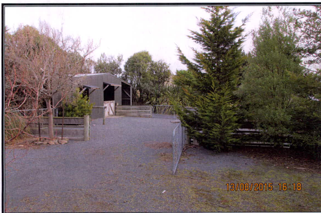
This photo was taken from inside the site's car park area with the large barn/shed in view in the back ground. Cleghorn Street carriageway is behind this view. (Photo taken: August 2015)
