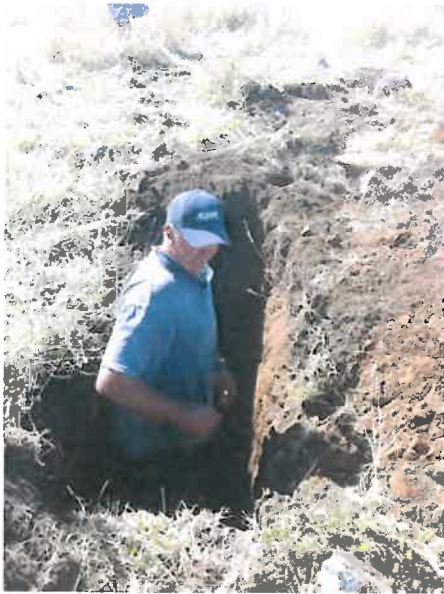
Figure 6: Photograph of test pit dug for testing tower foundation
