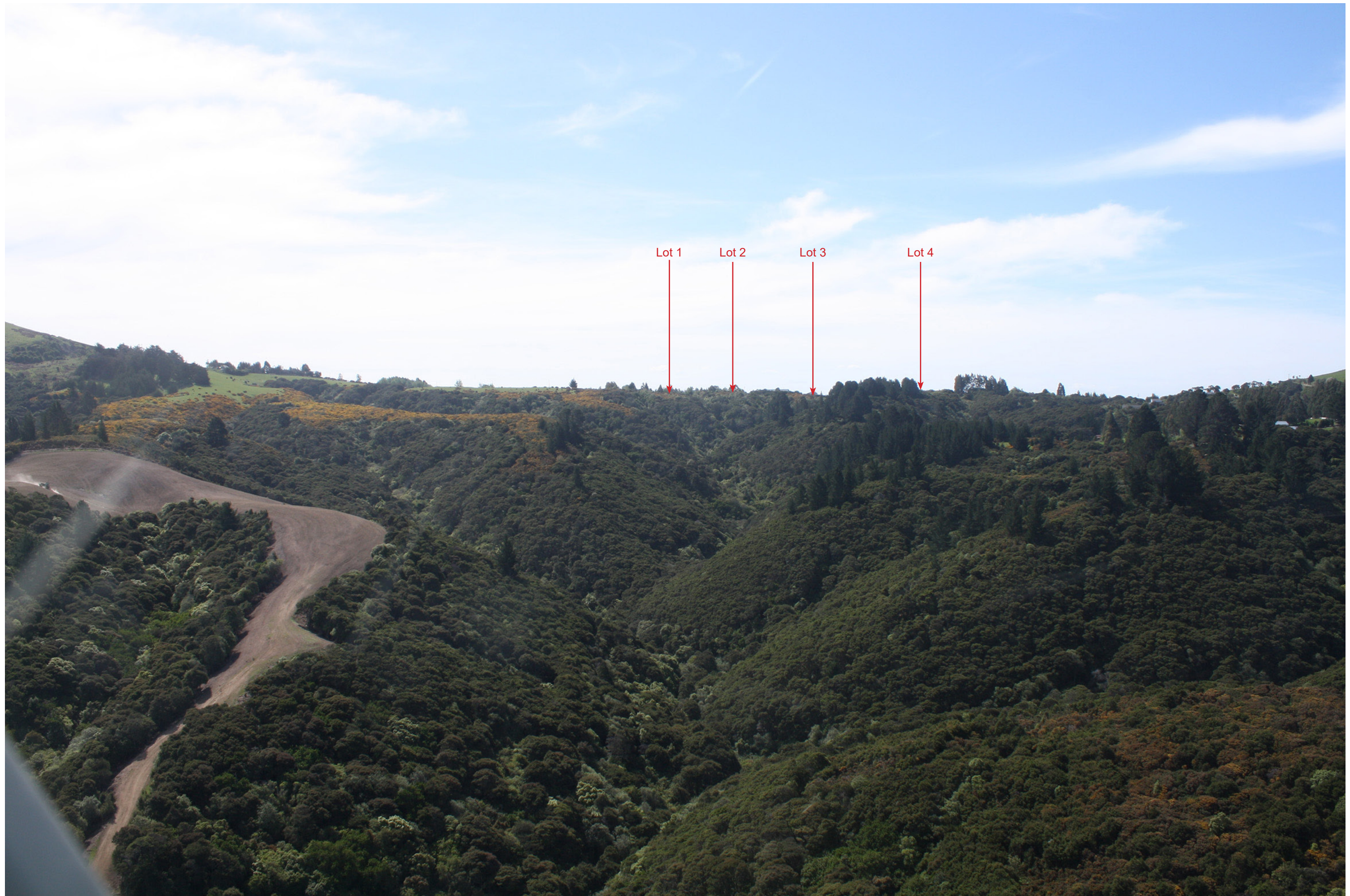
Figure 2 : Oblique Aerial view over 505 Saddle Hill Road
