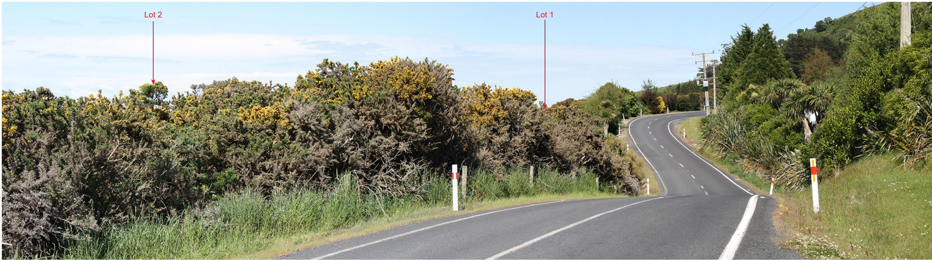
Figure 3 : View westward along Saddle Hill Road from its intersection with Sproull Drive
