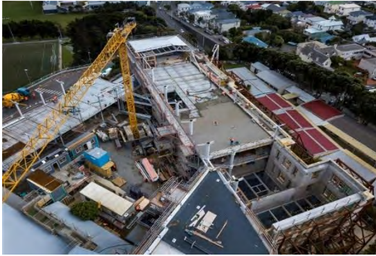
Figure 31: Aerial view showing the construction proceeding.
