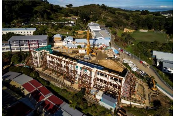
Figure 26: External view of the temporary propping.
