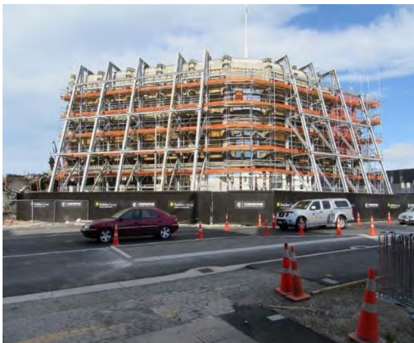
Figure 1: External view of temporary propping to façade.
