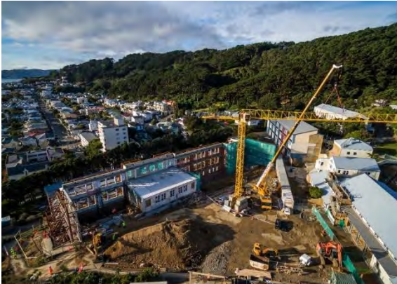
Figure 25: Aerial view of the temporary support.
