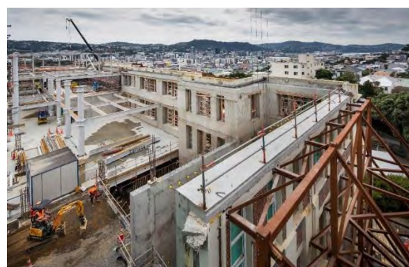
Figure 30: Internal view of the building progressing.
