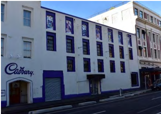
Figure 15: Cumberland Street façade of Block 1.
