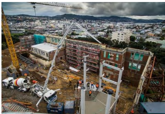
Figure 27: Internal view showing the start of the strengthening works required.
