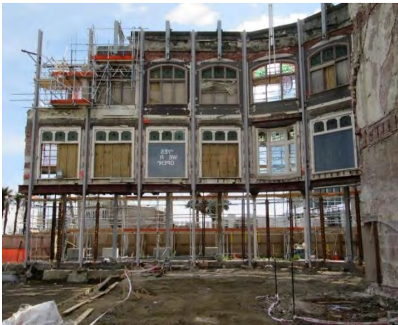
Figure 33: Inside view of the temporary support for the Mackenzie and Willis façade Christchurch.
