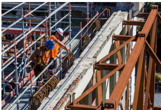
Figure 29: Internal concrete beams to reinforce and support the brickwork.
