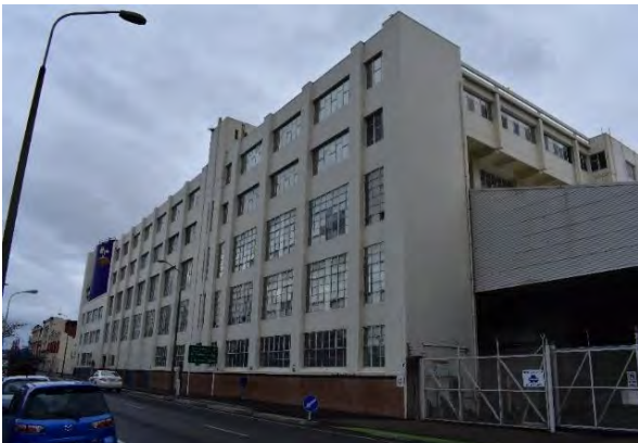
Figure 24: Castle Street elevation of Block 5.
