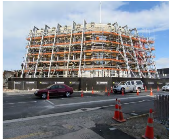
Figure 34: External view of the temporary propping.
