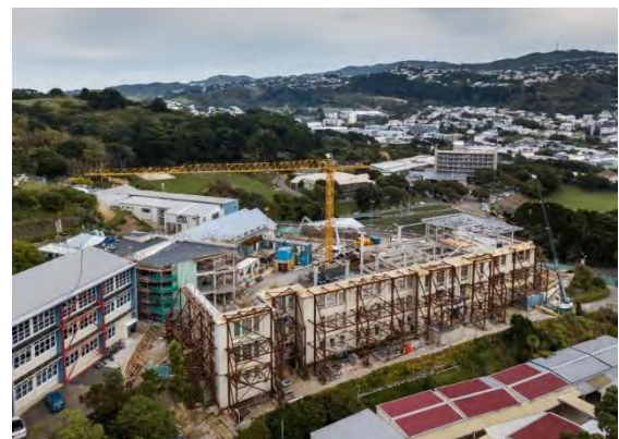
Figure 28: view showing the extent of the temporary propping.
