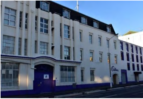
Figure 18: External view of the block 2 façade looking South.
