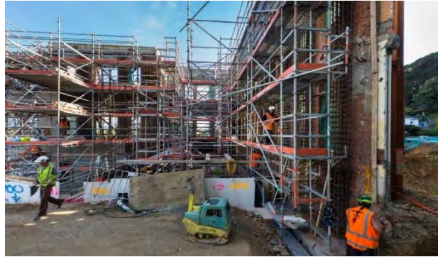
Figure 32: Extent of the strengthening work inside.
