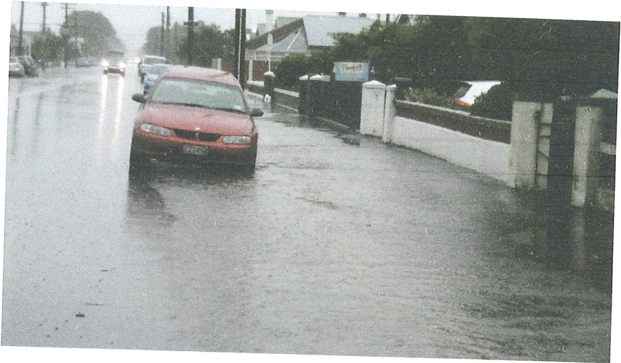
February 2020 Surface Flooding (NOT fixed)
