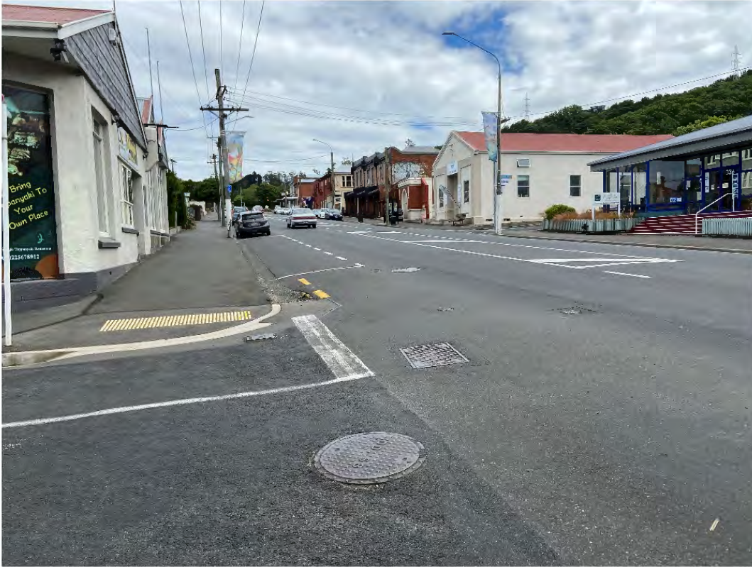
Photograph 2-3: South Rd — view west from College St
