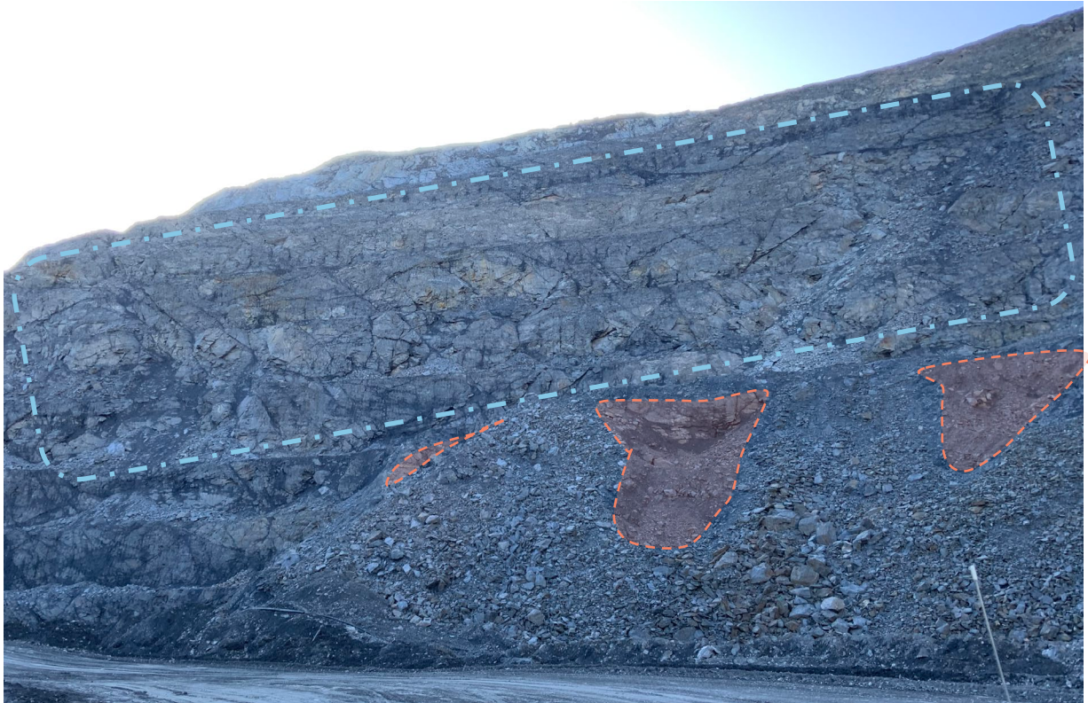
Photo 8: Fraser 6/FRIM north wall - Surface caving expression of near surface stopes highlighted in orange. Dilated structures associated with rock mass relation visible through the zone in blue.
