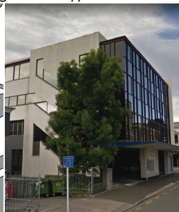
■ Partial curtain wall
