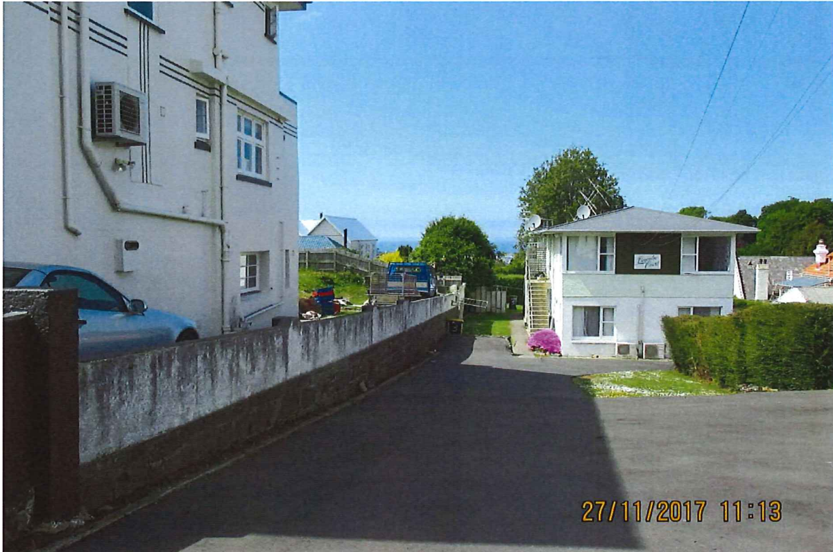
Photo 5: The photo has been taken from the footpath of High Street, looking towards the back yard of 403 High Street. The house on the left is that of 403 High Street, and the building on the right is the flats of 409 High Street. The bluestone wall can be seen on the lower half of the wall (the portion acting as a retaining wall).
