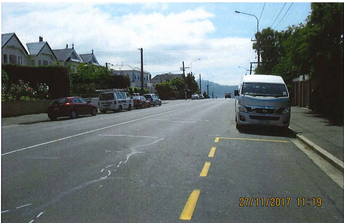
Photo 16: High Street, looking northeast from the driveway of 403 High Street.
