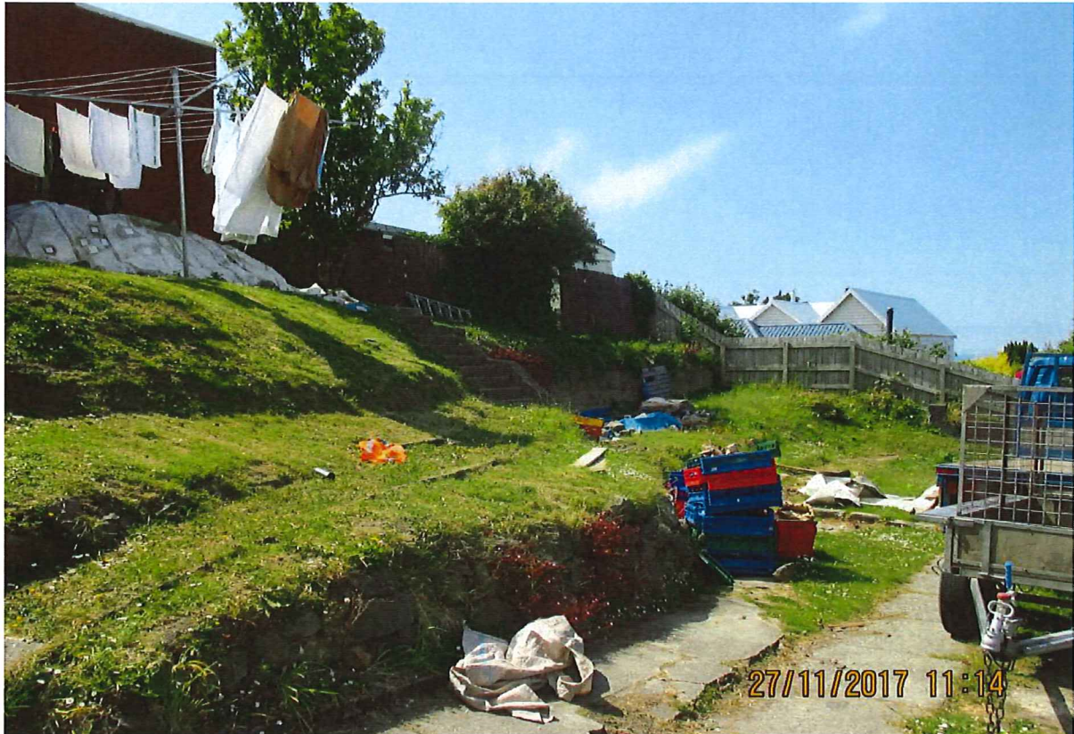
Photo 7: The back yard of 403 High Street with the existing terracing. The dark fence is on the boundary of 401 High Street. The light fence is on the boundary of 167 Maitland Street.
