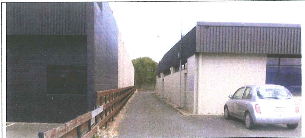
Above: Boundary wall of the neighbouring property at 547 Andersons Bay Road.
