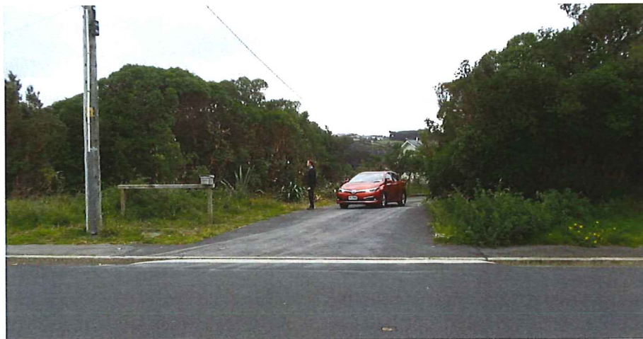
Figure L: The formed and sealed vehicle crossing onto Tomahawk Road.
