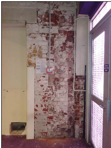
Figure C-34. Detail photograph of interior wall of Cadbury World building that would have originally form the north exterior wall of the pre-1900 kiln showing a possible ground floor partition wall and joist insertion point for the original mezzanine level.
