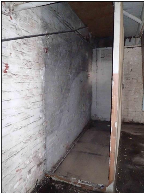
Figure C-45. Photograph showing former stairwell in the 1901 southern extension looking southwest in the most easterly room of the same building (right)
