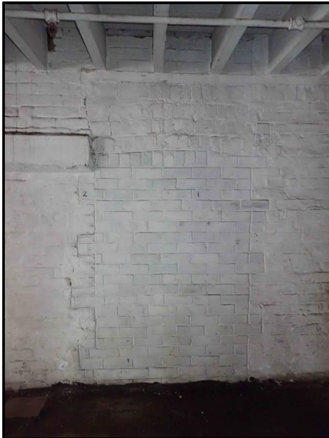
Figure C-37. Blocked in doorway in the former kiln building looking east.
