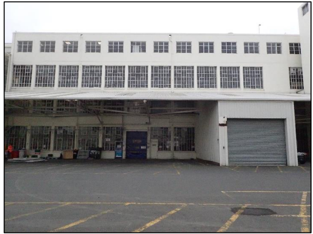
Figure C-75. Photograph looking north at the southern elevation of the chocolate and biscuit factory.
