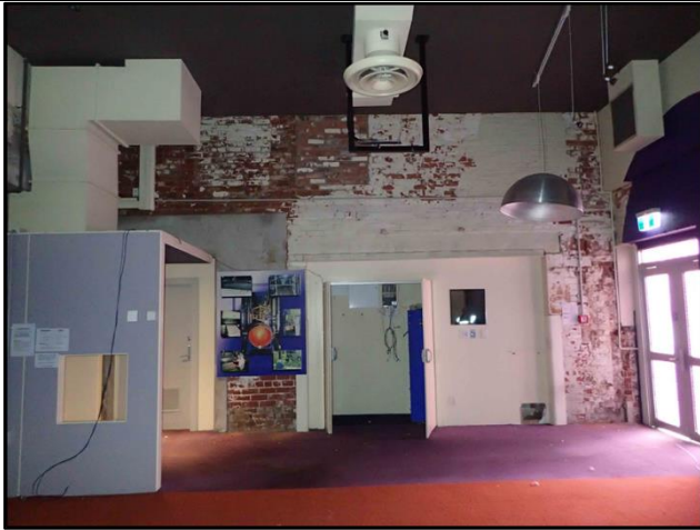
Figure C-32. Photograph of interior wall of Cadbury World building that would have originally form the north exterior wall of the pre-1900 kiln. Note the bricked in windows of what was once the mezzanine level.
