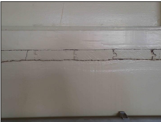
Figure C-90. Photograph looking east at tongue and groove of mezzanine above basement in engineering workshop, labs and office building.
