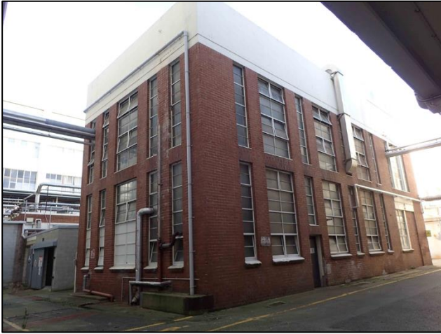
Figure C-113. Photograph looking southeast at central boiler house constructed in the 1940s (Block 4B).
