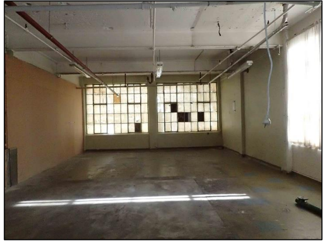
Figure C-72. Photograph looking north at chocolate factory and garage building on the first floor.
