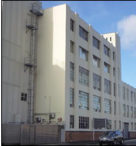
Figure C-98. Photograph looking southeast at the Cumberland Street façade of the biscuit and dispatch building.
