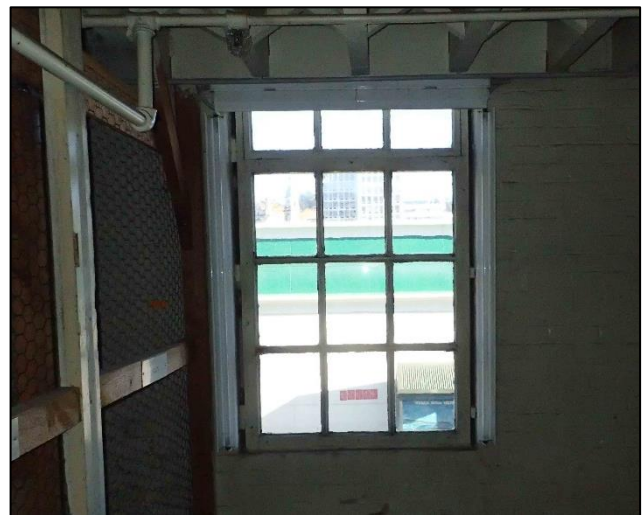
Figure C-46. Photograph looking west at multi-pane fixed window on the first floor of Cadbury World.
