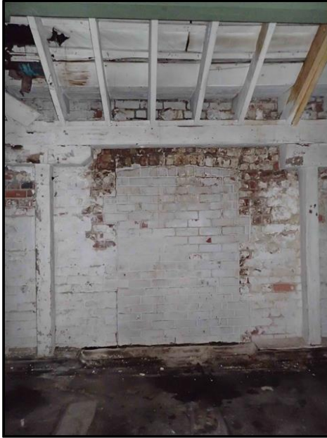
Figure C-51. Photograph looking east at a blocked in doorway in the second floor of the Cadbury World building, the most easterly room of the former kiln building.
