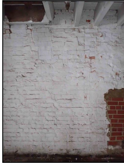
Figure C-36. Blocked in doorway in the former kiln building looking east.
