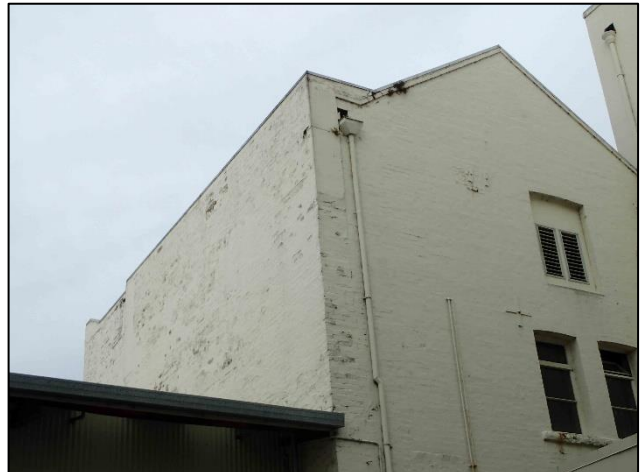
Figure C-25. Photograph looking southwest at the eastern and northern wall of former smutters and kiln building. The upper floor was added sometime between 1892 and 1901, while the southern extension of 1901 is visible at the rear. There is one blocked in window on the eastern wall and another on the northern wall.
