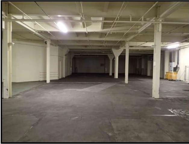
Figure C-71. Photograph looking west at the former garage on the ground floor.
