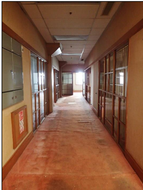
Figure C-63. Photograph looking south at office portion of the office building on the first floor.
