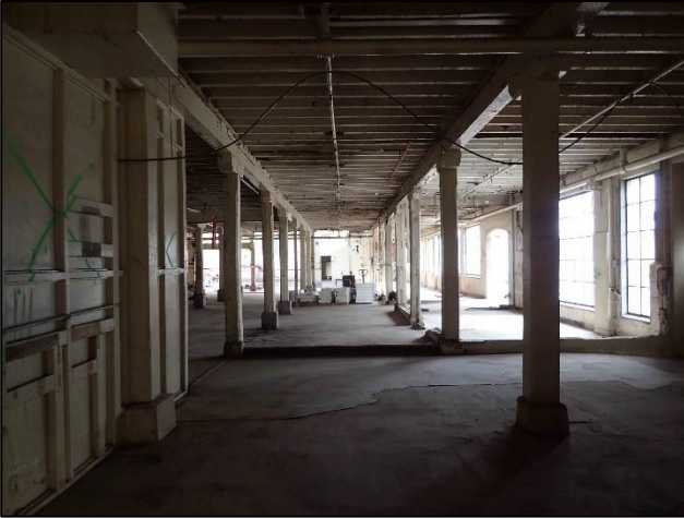
Figure C-18. Photograph looking west at the ground floor of dairy and machine house building.
