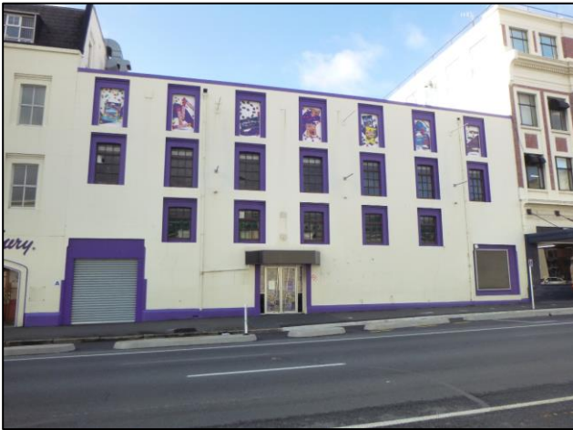
Figure C-24. Photograph looking east at the Cumberland Street façade of Cadbury World.
