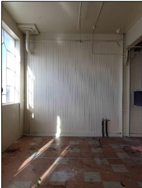
Figure C-83. Photograph looking south at tongue and groove wall lining on the second floor of Building 3 (Block C).
