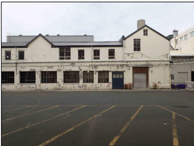
Figure C-3. Photograph looking south at the eastern elevation showing two distinct portions: the central dairy and the western machine house.
