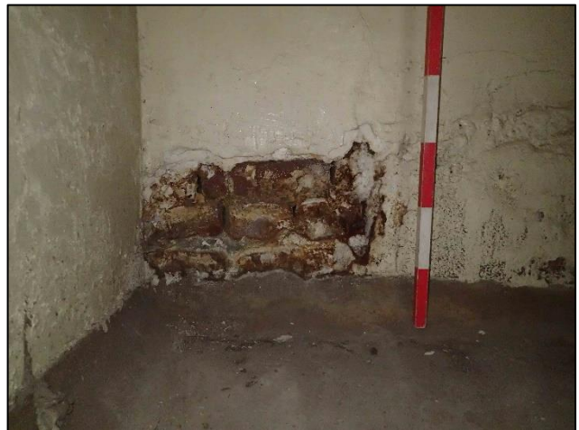
Figure C-23. Photograph looking west at the plastered brick wall of ground floor in the machine house portion of dairy and machine house building.
