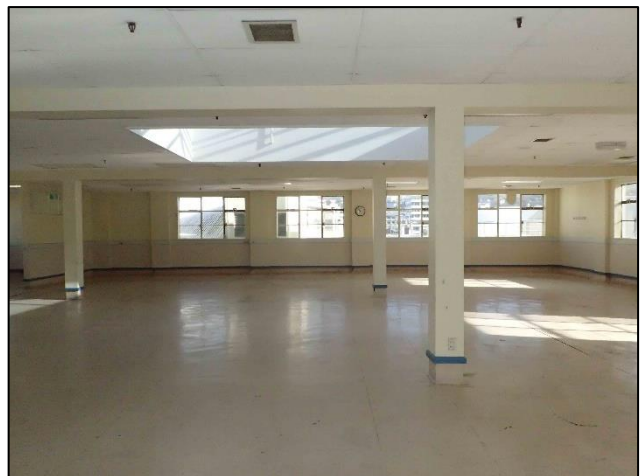
Figure C-79. Photograph looking west at third floor cafeteria of chocolate and biscuit factory building.
