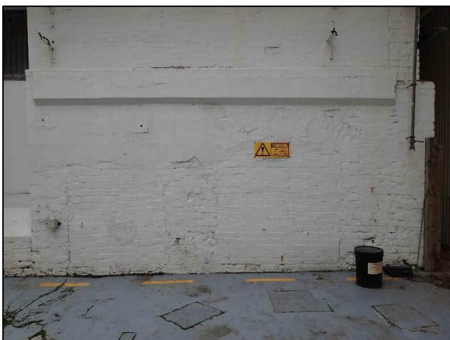
Figure C-5. A close-up photograph looking east at the western wall of the machine house showing the blocked-in windows.
