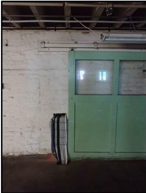
Figure C-41. Photograph looking east at two blocked in doorways (top) either side of current doorway (bottom) to the eastern room of the former kiln and smutters room.
