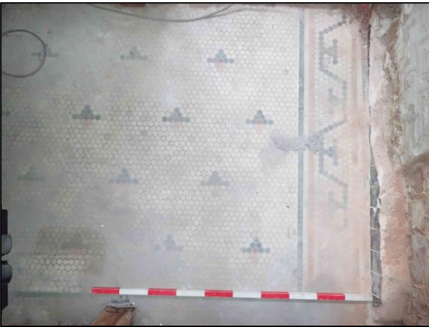
Figure C-20. Photograph showing penny tiling in the office portion of the dairy and machine house building.
