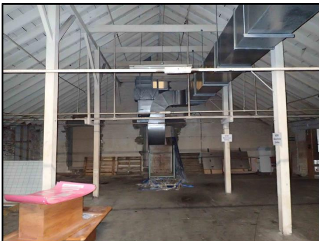
Figure C-49. Photograph looking north at the roof framing and the windows of the second-floor north wall of the Cadbury World building associated with the 1901-1915 storey addition. Prior to the 1915-1922 raising of the offices and shop building this would have been an exterior wall.
