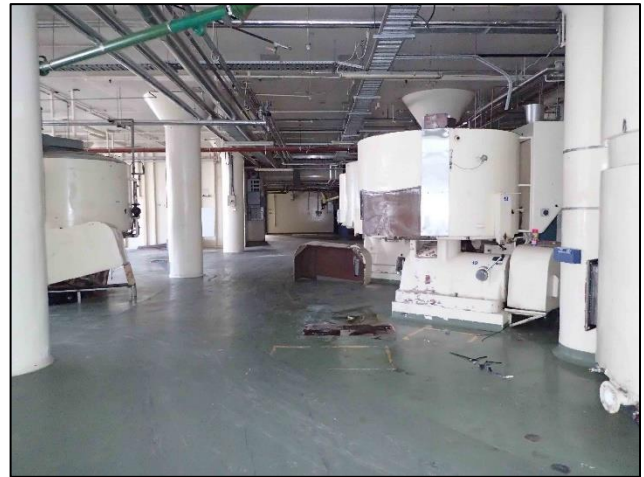
Figure C-104. Photograph looking north at the biscuit and dispatch building (Block 5A) on the first floor.
