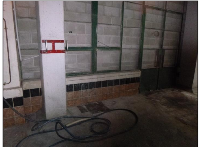
Figure C-118. Photograph looking north east at covered in area (Block 4B) to the rear of the dispatch building, possibly once the exterior as features the same brown tiling as seen on Building 4 façades.
