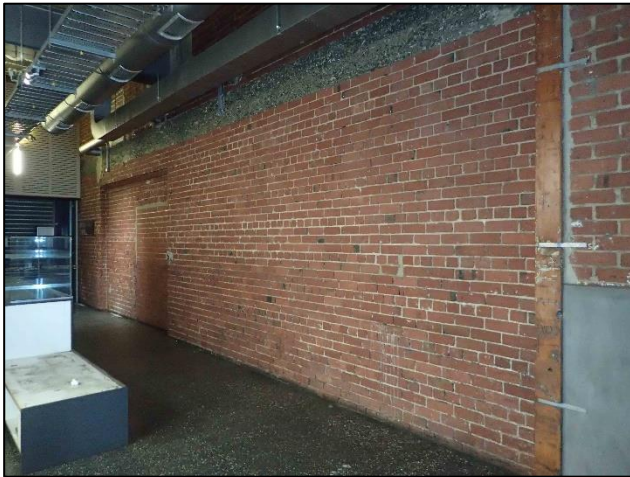
Figure C-28. Photographs looking northwest at southern internal partition wall on the ground floor of the Cadbury World café. The wall was likely present from 1922. Note the blocked-in doorway on the northern internal wall.
