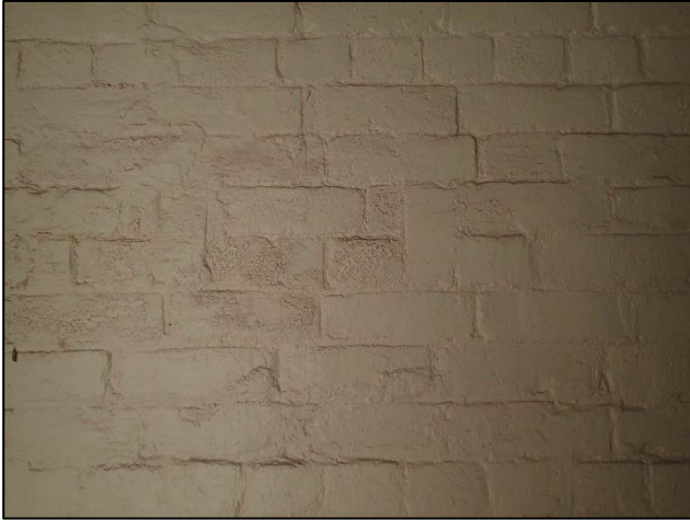
Figure C-14. Photograph looking south on ground floor of the dairy building at possible joist insertion points. These are at the same height as the first former staircase landing and possibly indicate there was a mezzanine floor at this height.
