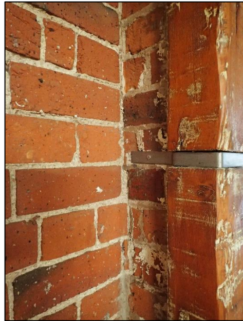
Figure C-29. Photographs looking northeast at the abutment of southern internal partition wall on the ground floor of the Cadbury World café to an earlier external wall to the west.
