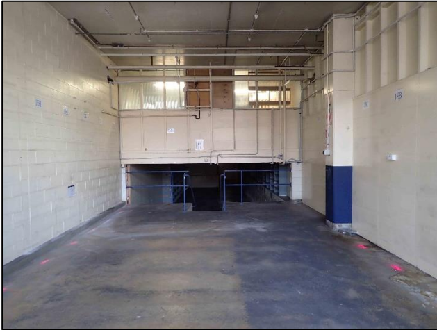
Figure C-88. Photograph looking east into basement and at mezzanine of engineering workshop, labs and office building from ground level.
