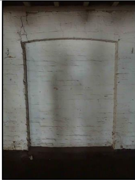
Figure C-40. Photograph looking east at blocked in doorway to the eastern room of the former kiln and smutters room.
