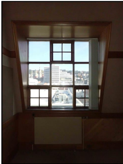
Figure C-67. Photograph of window on third floor looking west facing out from the mansard roof (right).
