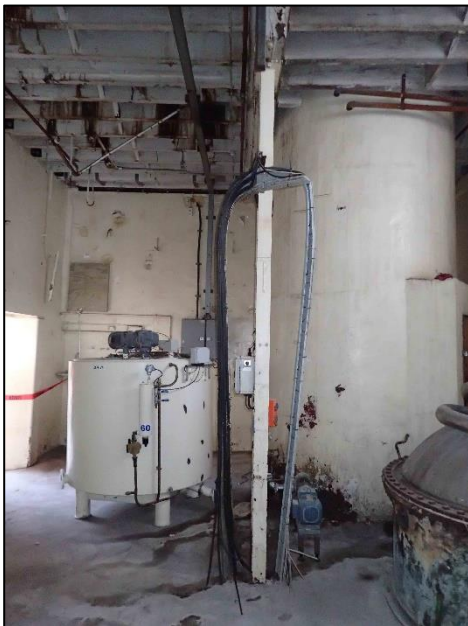
Figure C-22. Photograph looking south machine house portion of the dairy and machine house building. The larger cylindrical item to the right is the base of the once 90 ft. concrete chimney
