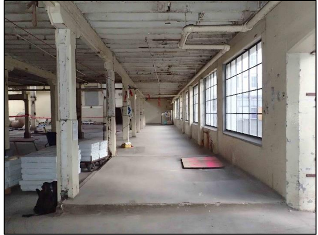
Figure C-19. Photograph looking west at the north side of the central dairy portion of the dairy and machine house building.
