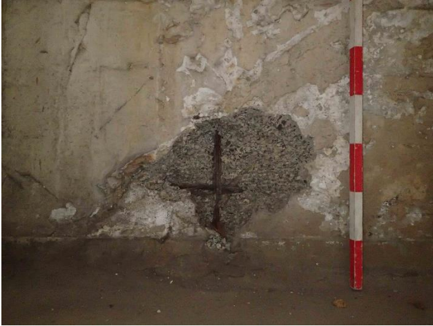
Figure C-117. Photograph looking west at ground floor wall in central boiler house (Block 4B). Note the concrete and steel construction.
