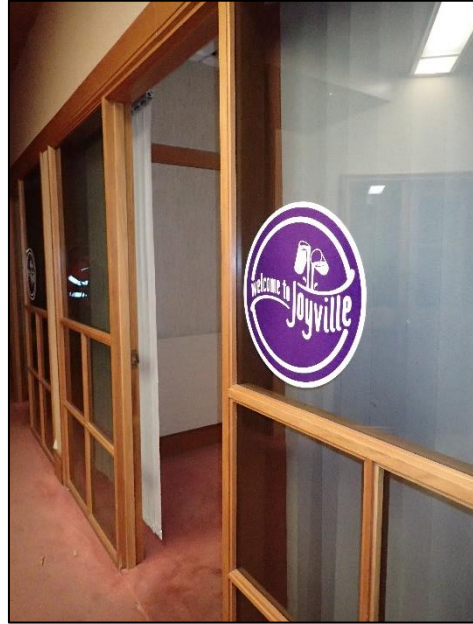
Figure C-62. Photograph looking northwest at office portion of the office building on the first floor showing Cadbury Joyville sign
