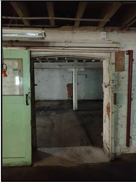
Figure C-39. Photograph looking east at blocked in doorway to the eastern room of the former kiln and smutters room.
