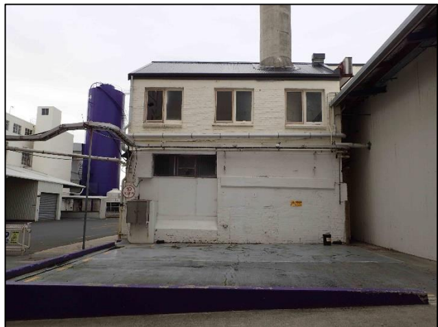
Figure C-4. Photograph looking east at the western wall of the machine house showing blocked-in windows.
