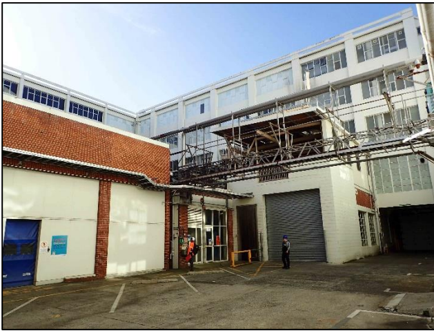
Figure C-100. Photograph looking northeast at the rear of the biscuit and dispatch building.
