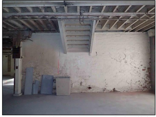
Figure C-9. Photograph looking north at partition wall with two blocked windows and the bottom of the stairwell leading from the partitioned area to the first floor.
