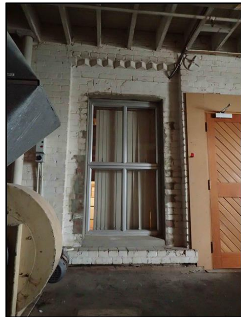
Figure C-60. Photograph looking north at a former exterior window of the office building (Block 2A) associated with the 1915-1922 third storey addition to the building. This photograph is taken from the later 1922-1927 addition at the rear of the Cadbury World building on the first floor
