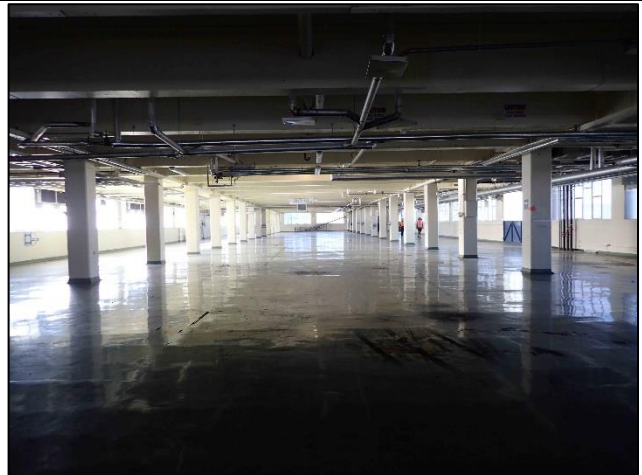
Figure C-108. Photograph looking east at the biscuit and dispatch building (Block 5B-C) on the third floor.
