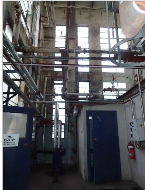
Figure C-116. Photograph looking north at ground floor in central boiler house (Block 4B).
