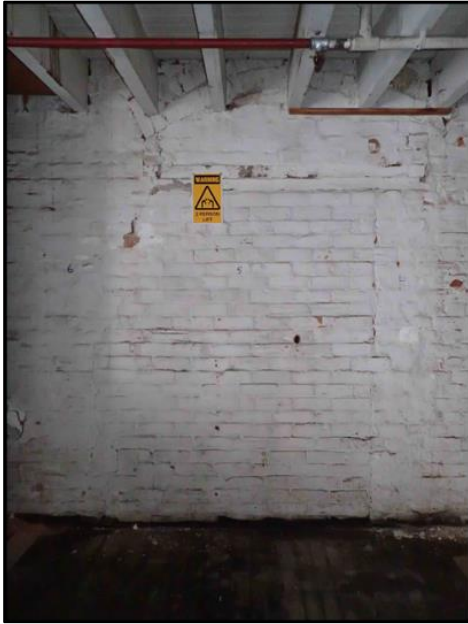
Figure C-35. Blocked in doorway in the former kiln building looking east.
