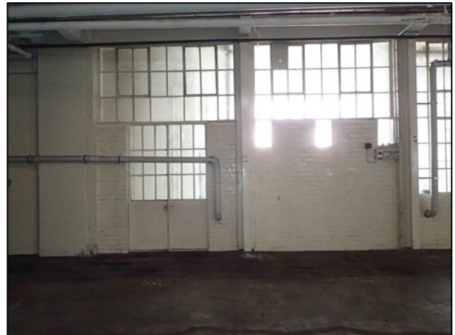
Figure C-82. Photograph looking south at bricked in wall section in Block B-C of Building 3 on the ground floor
