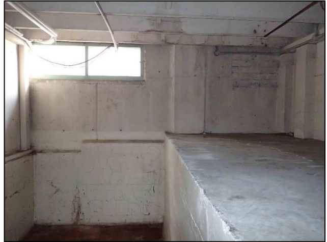
Figure C-89. Photograph looking east at basement wall of Building 4 (Block 4A). Note the brick infill and the open window running up into the mezzanine level above.
