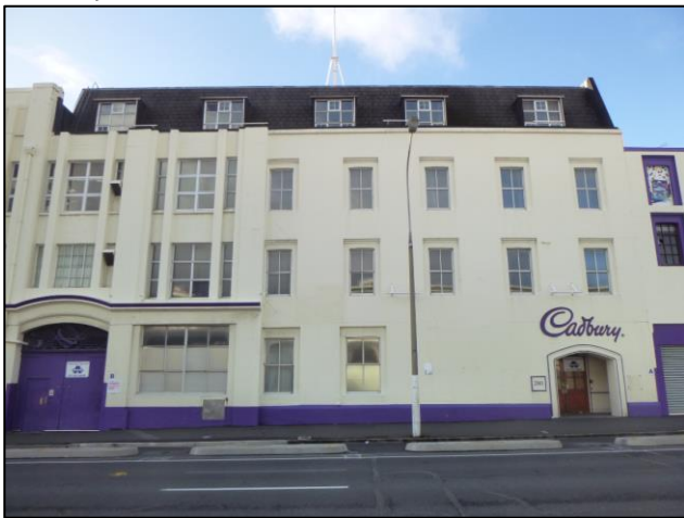
Figure C-57. Photograph looking east at the Cumberland Street façade of Office Building.
