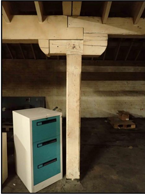
Figure C-47. Photograph looking south at column on second Floor 2 of the Cadbury World building with the 1901 southern extension behind.
