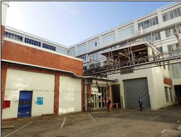
Figure C-115. Photograph looking northeast at central boiler house extensions in the 1950s and 1960s (Block 4B).
