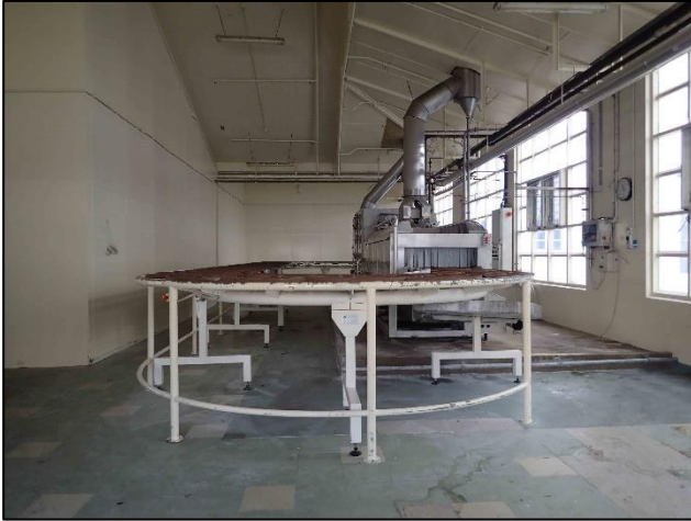
Figure C-94. Photograph looking west at engineering workshop, labs and office building showing tin wash on second floor.
