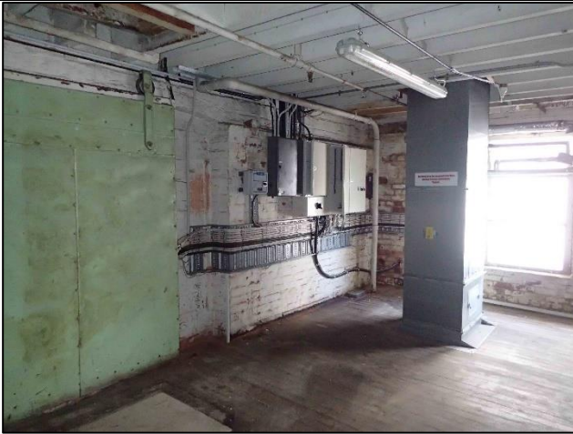
Figure C-43. Photograph looking northwest at blocked in doorway and stepped out portion of the wall into the eastern room of the former kiln building.
