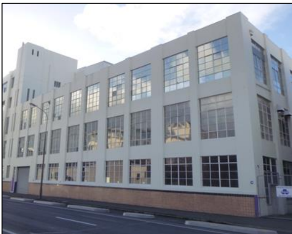
Figure C-86. Photograph looking northeast at the Cumberland Street façade of engineering workshop, labs and office building.
