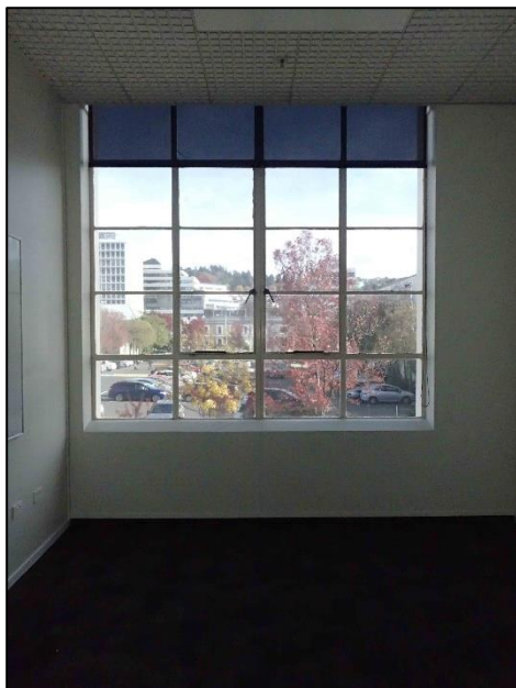
Figure C-96. Photograph looking west window of engineering workshop, labs and office building on the first floor.
