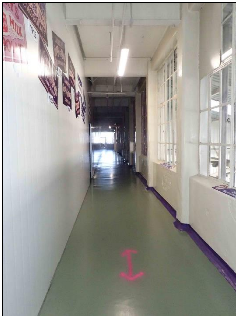
Figure C-73. Photograph looking north at corridor along chocolate factory and garage building on the first floor.
