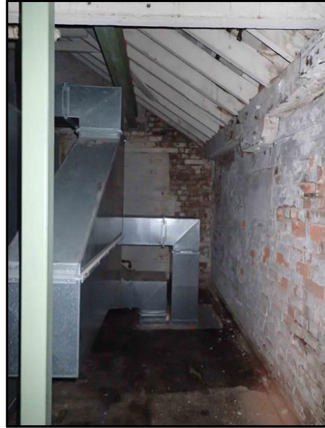
Figure C-52. Photograph looking north (left) at a blocked in window in the second floor of the Cadbury World building, the most easterly room of the former kiln building.
