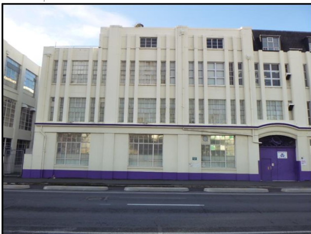
Figure C-70. Photograph looking east at the Cumberland Street façade of the chocolate factory and garage building
