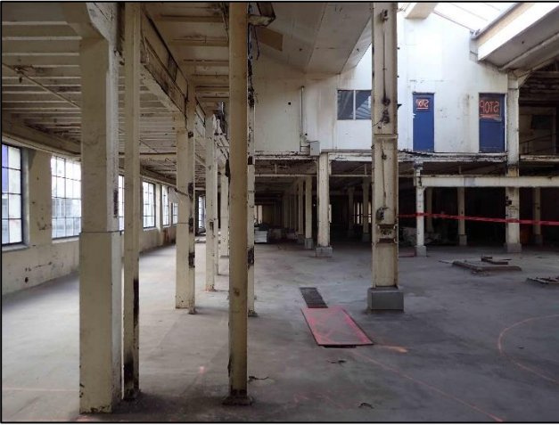
Figure C-8. Photograph looking east at second floor of the dairy and machine house building.
