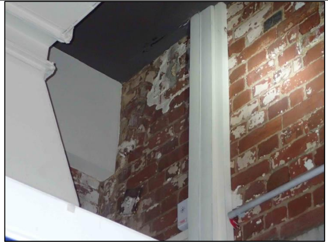
Figure C-33. Detail photograph of interior wall of Cadbury World building looking northwest that would have originally formed the north exterior wall of the pre-1900 kiln showing an arch above a blocked-in window.
