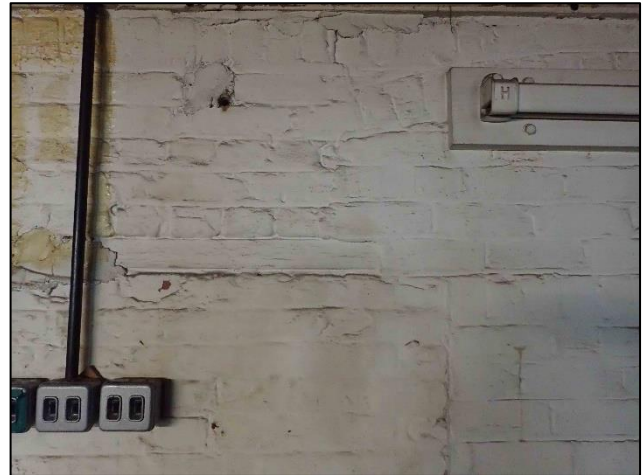
Figure C-42. Photograph looking south at detail of blocked in doorway of the former kiln building. Note the wood to the left of the doorway
