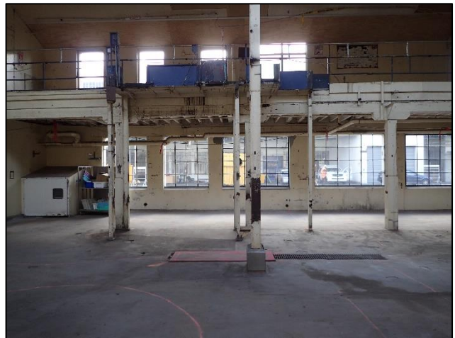
Figure C-17. Photograph looking north at multi-pane windows of the dairy central portion of dairy and machine house building.
