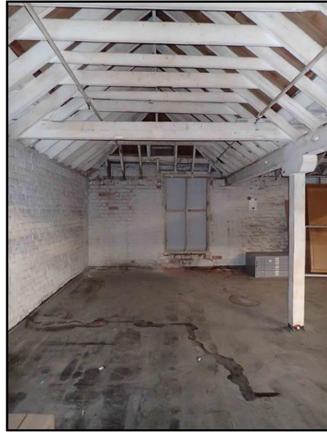
Figure C-48. Photograph looking west at roof structure of the southern extension.
