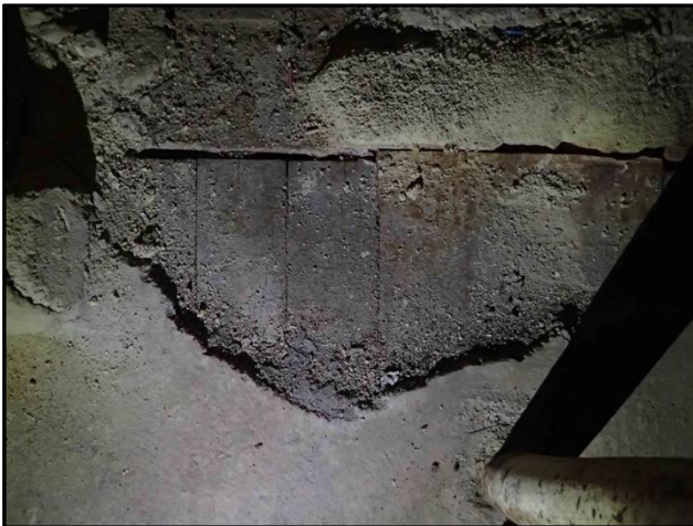
Figure C-53. Photograph of tongue and groove timber underneath concrete of the floor in the 2nd floor of the Cadbury World building.
