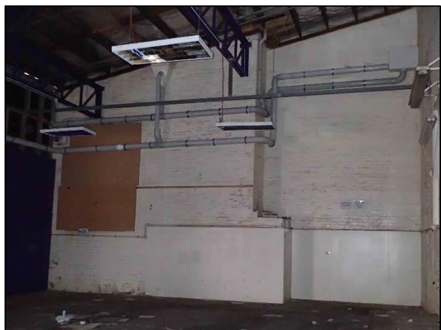
Figure C-6. Distinct dog-legged wall of the former shared wall between what was once the cellar (presently referred to as the dairy building) and the mill.
