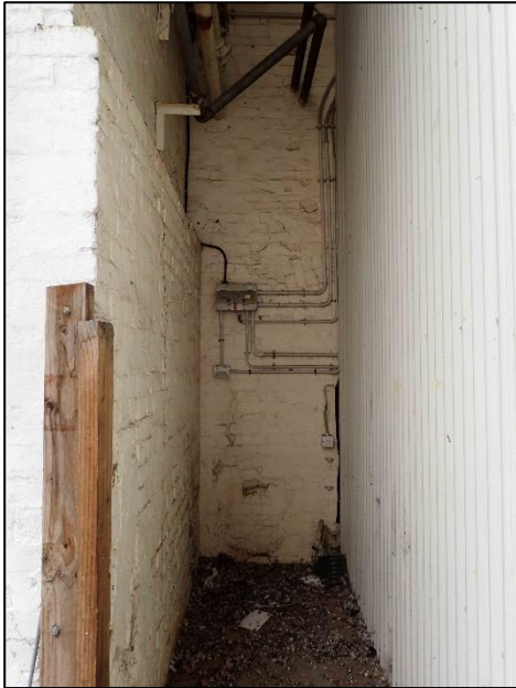
Figure C-7. Photograph looking east at the former doorway or window arch located on the shared wall between what was once the cellar (presently referred to as the dairy building) and mill.
