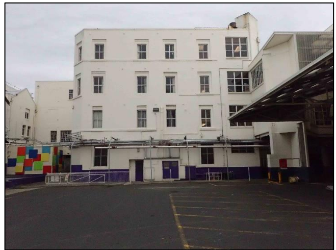
Figure C-58. Photograph looking west at the rear of the office building and 1920s addition to the rear of Cadbury building
