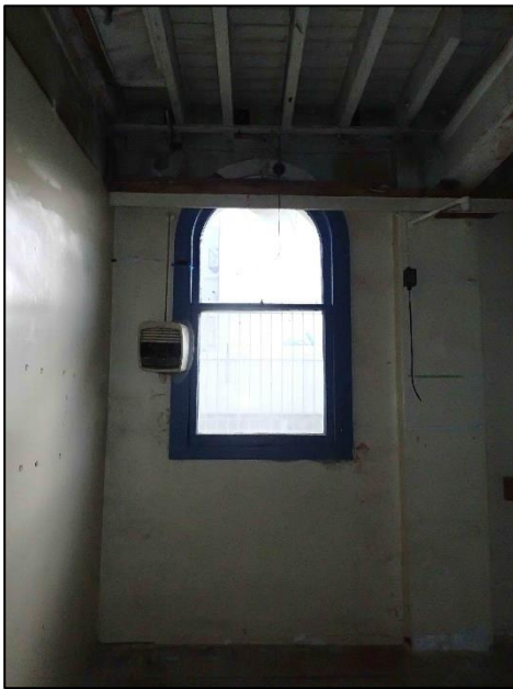
Figure C-16. Photograph looking north at single hung sash window in the office portion of the dairy and machine house building.
