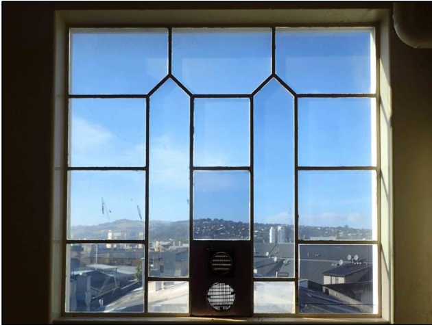
Figure C-84. Photograph looking east at decorative window in Building 3 Building 3B-C on the second floor.
