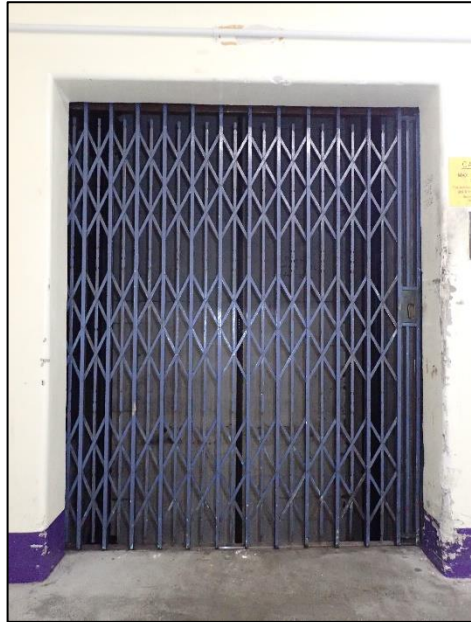
Figure C-81. Photograph looking west at third floor lift shaft.
