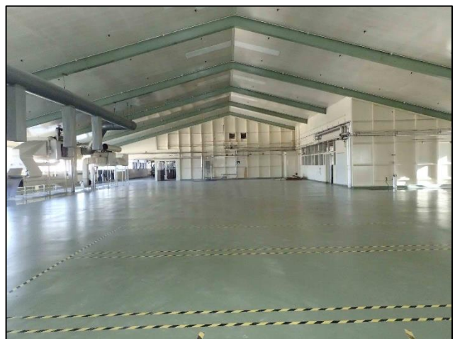
Figure C-110. Photograph looking west at fourth floor of the biscuit and dispatch building (Block 5C).
