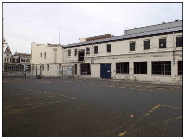
Figure C-2. Photograph looking southeast at the eastern elevation showing two distinct portions: the eastern offices and the central dairy.
