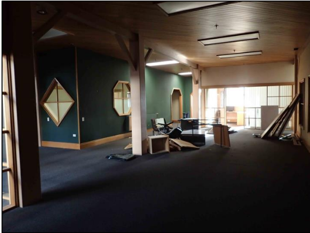
Figure C-65. Photograph looking northeast at office space on the third floor.
