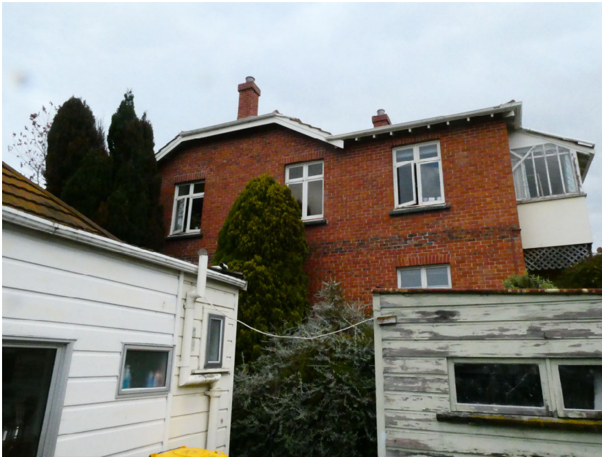
Figure 1: Eastern facade of 45 Cargill Street (as view from subject site)
