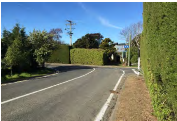
Figure 5-2: On Hill Road looking south towards curve 2
