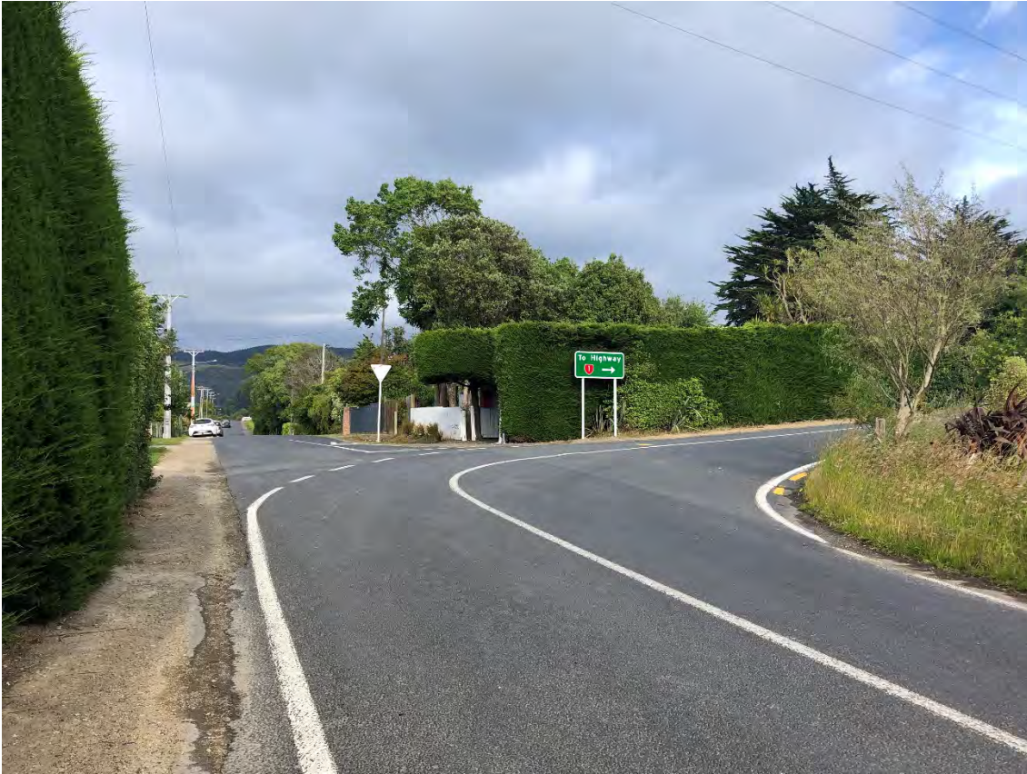
Photograph 6: BAY Road / Hill Road Intersection
