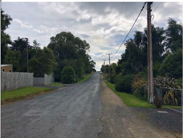
Image 8: View looking east along Bay Road from the driveway of the site.
