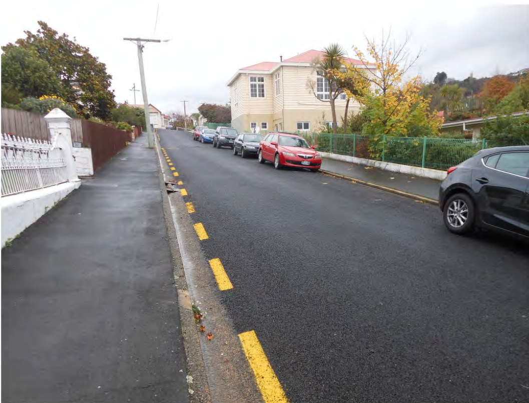
Photograph 2-11: Lomond St – view west
