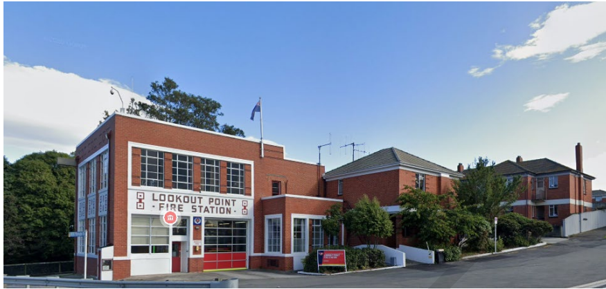
Figure 1. Lookout Point Fire Station in 2020. 1
