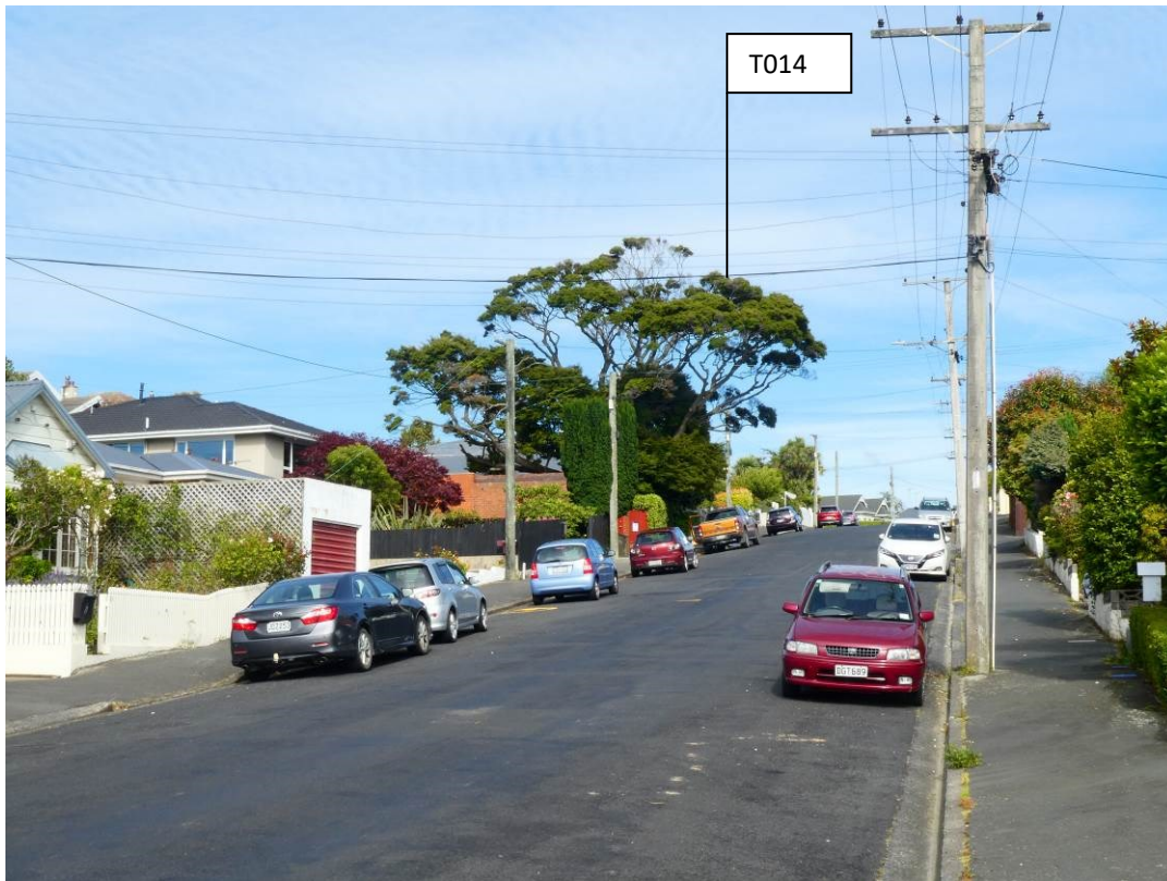
Figure 1. View towards T014 from the east on Preston Crescent.
