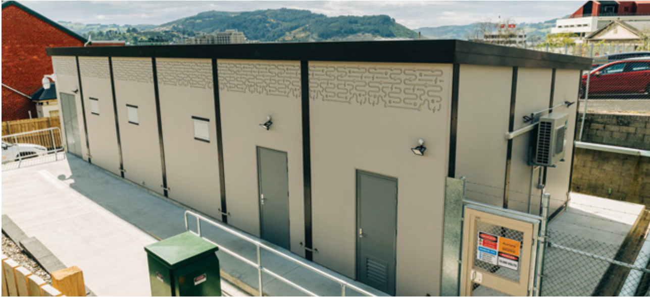
Smith St: The Smith Street Zone Substation Upgrade strengthened electricity supply and created greater network resilience and back-up supply options for customers in central Dunedin and Roslyn.
