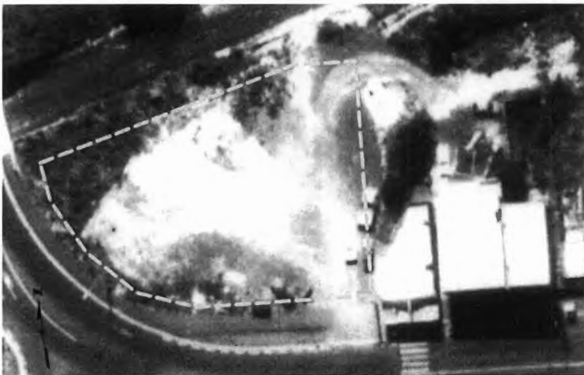
Figure 10: The site in 1990 showing that the site has been cleared of the Sydney Street rail overbridge and the small utility building that had been fronting Sydney Street. It appears that the site was also being filled at the time of the photograph (Source DCC)
