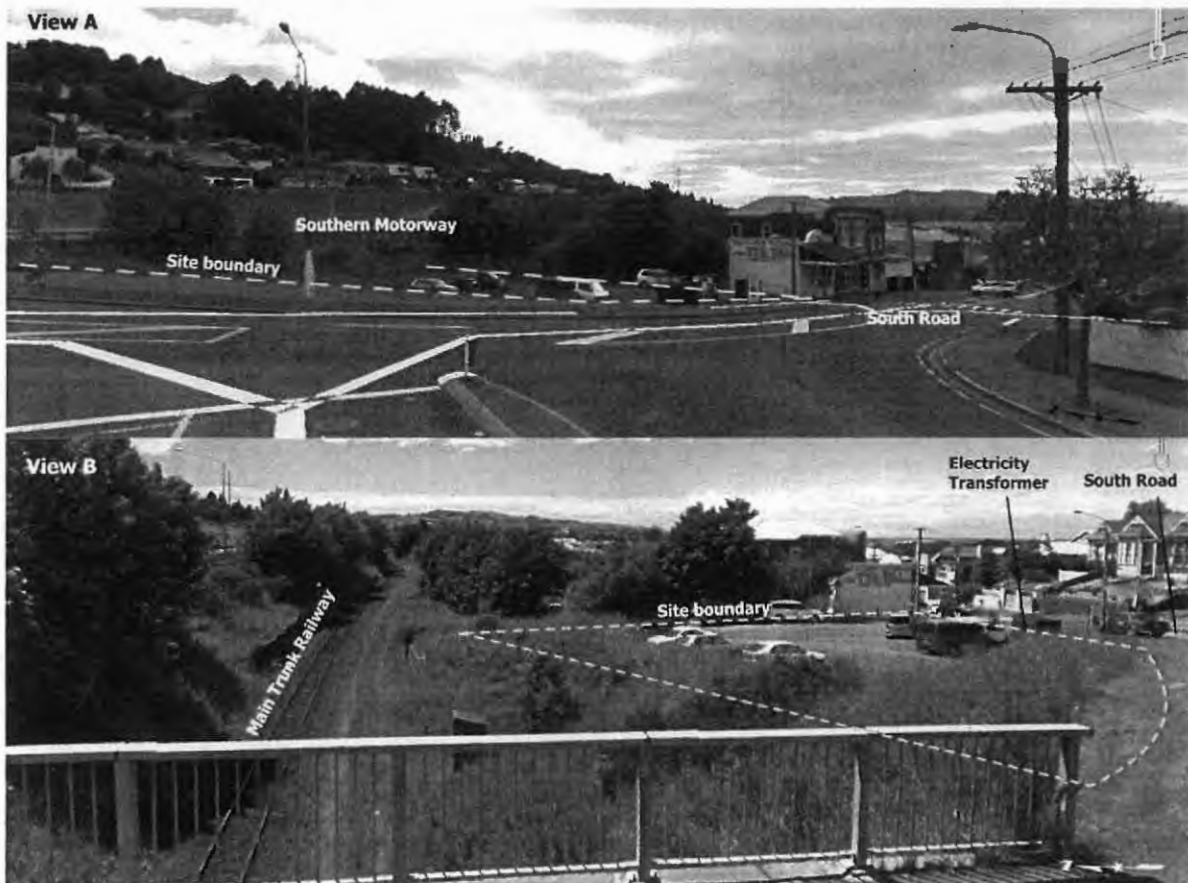
Figure 14: Photos of site boundaries from 2014 (Google Earth); Photo A is from the intersection of South Road and the Caversham SH1 on-ramp. Photo B is from the SH1 on-ramp rail over-bridge showing the relationship between the site and the railway and motorway and adjoining shops and residential area of Caversham.
