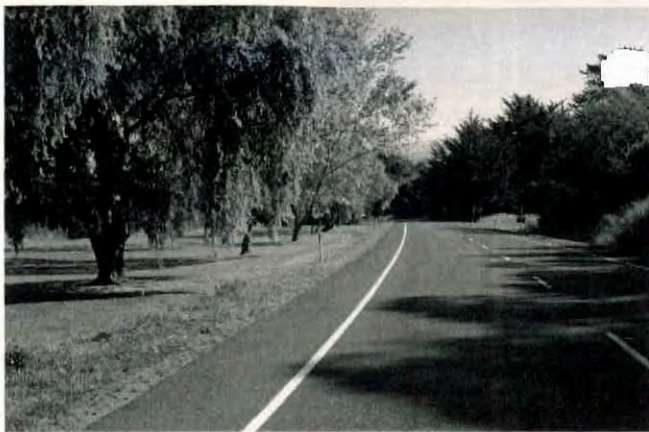
Vpt.3 - North-east approach to Outram past the site on Mountfort Street
