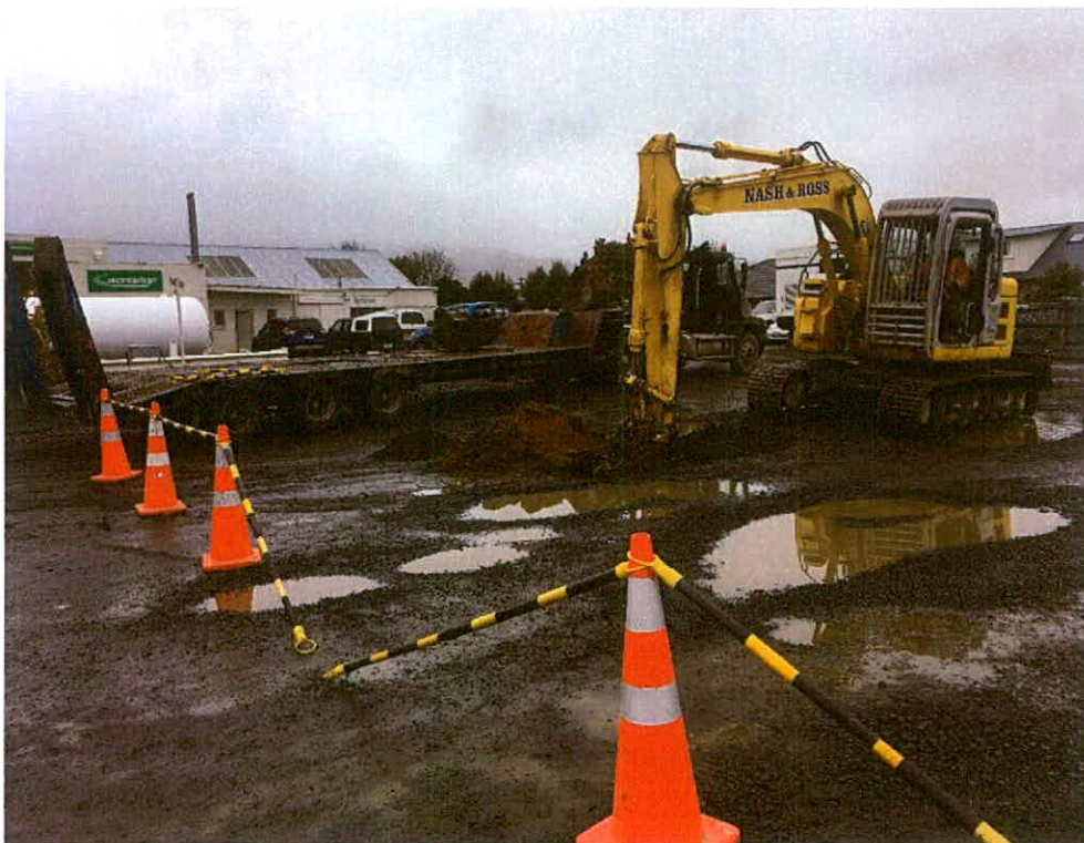
Site Photograph 6: Nash & Ross digging first test pit at location TP004 (taken 01/06/2017).
