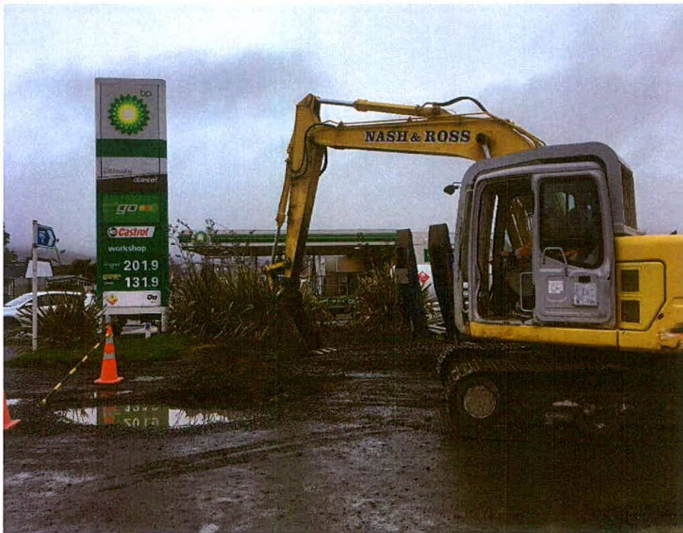
Site Photograph 5: Nash & Ross clearing for underground services prior to McMillan Drilling Group's cone penetrometer rig at location CPT003 (taken 01/06/2017).
