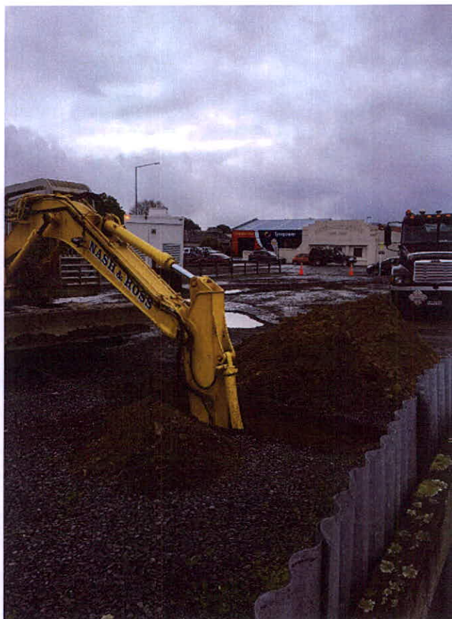
Site Photograph 7: Nash & Ross digging second test pit at location TP005 (taken 01/06/2017).
