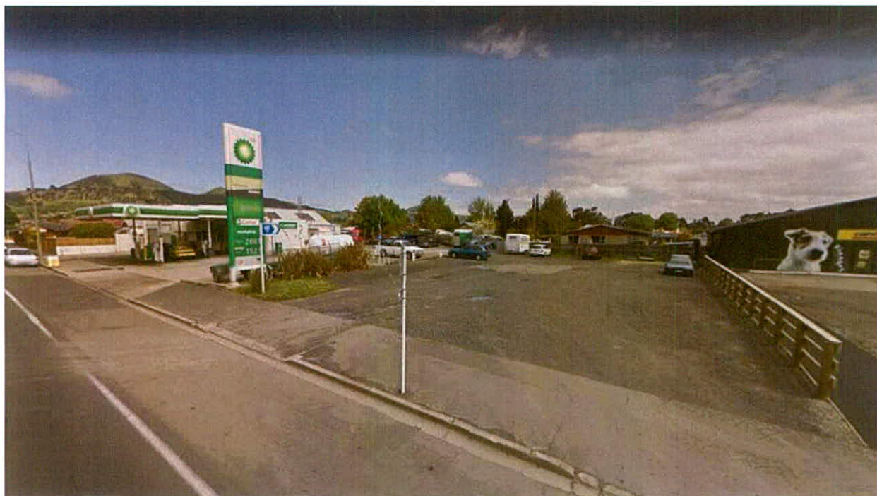
Site Photograph 1: BP Mosgiel from Gordon Road facing southwest (Source: Google Maps 2017, captured June 2017).
