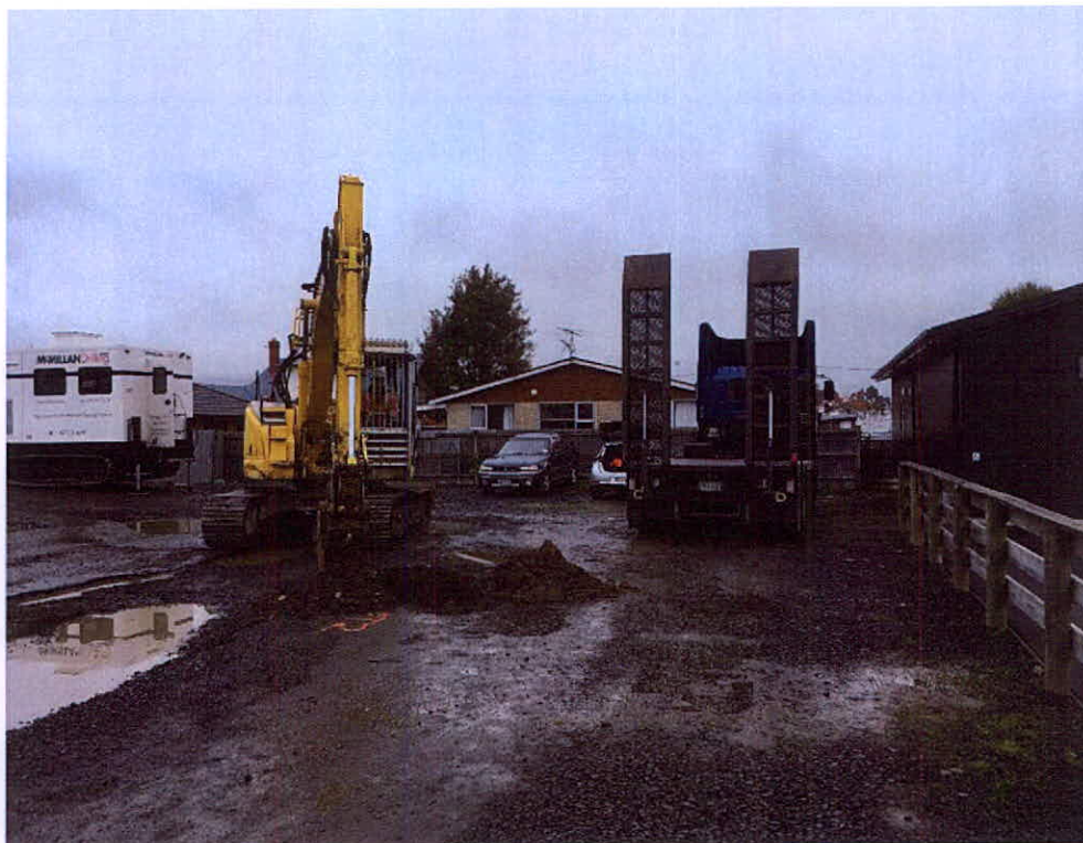
Site Photograph 3: Nash & Ross clearing for underground services prior to McMillan Drilling Group's cone penetrometer rig at location CPT002 (taken 01/06/2017).
