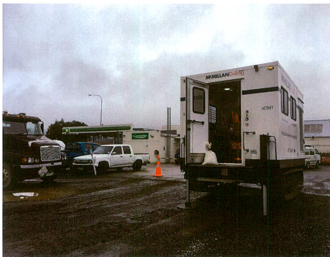
Site Photograph 2: McMillan Drilling Group cone penetrometer rig at location CPT001.
