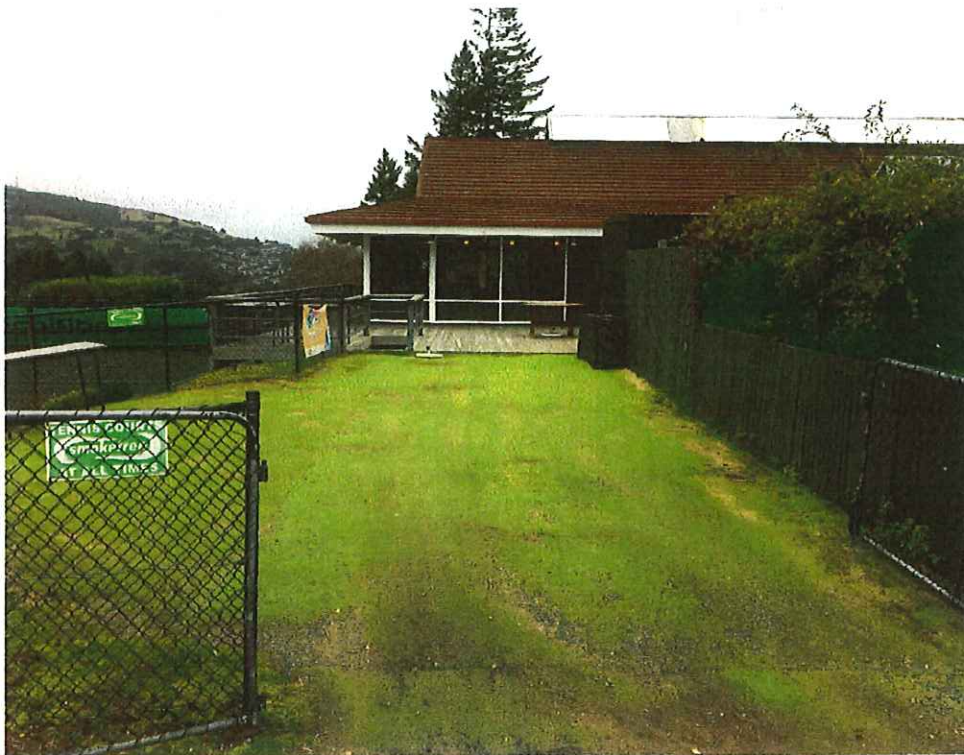
Above: Mobility entrance to building from tennis court area
