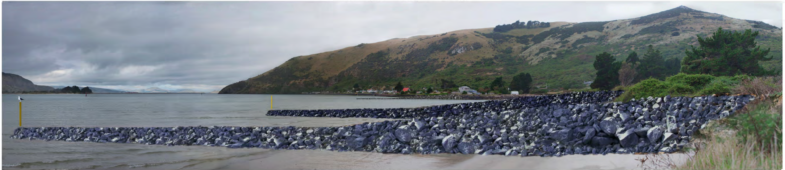
View A (Low tide) with groynes.
