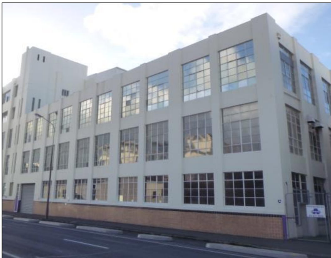
Figure 7-55 Cumberland Street (left) and Castle Street (right) façades of the biscuit and dispatch building.
