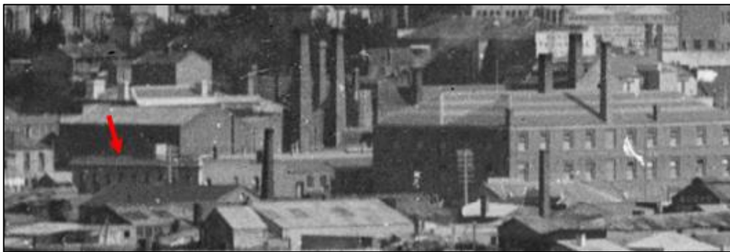
Figure 5-43. Top: 1902 photograph of the cellar building with the office alterations at the front along Castle Street (red arrow) (Muir and Moodie Studio, 1902).
