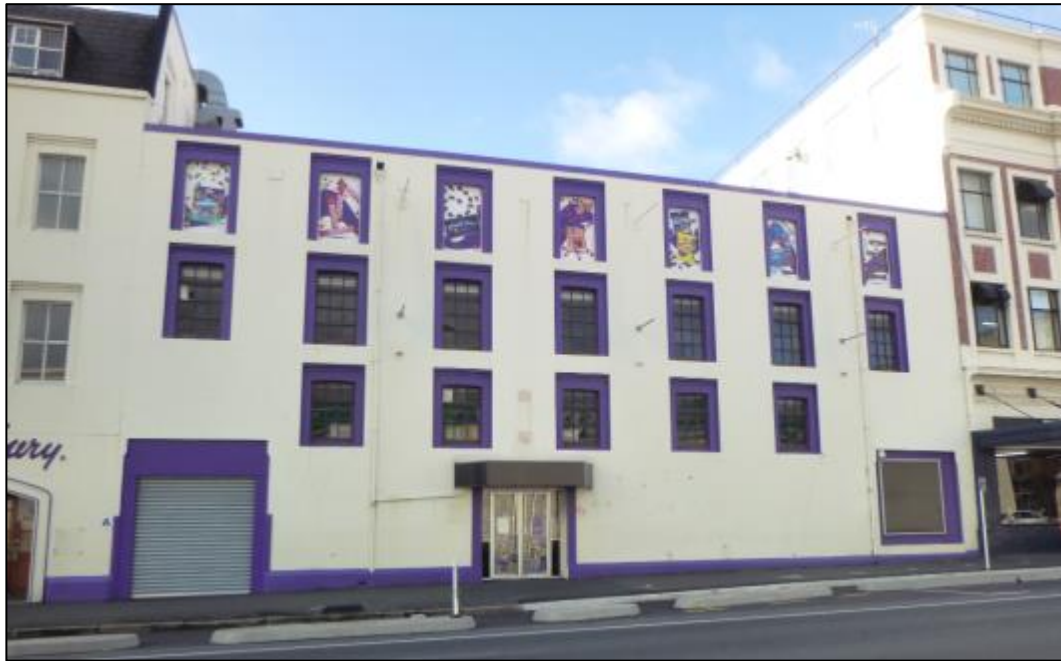
Figure 7-15 Photograph looking east at the Cumberland Street façade of Cadbury World.
