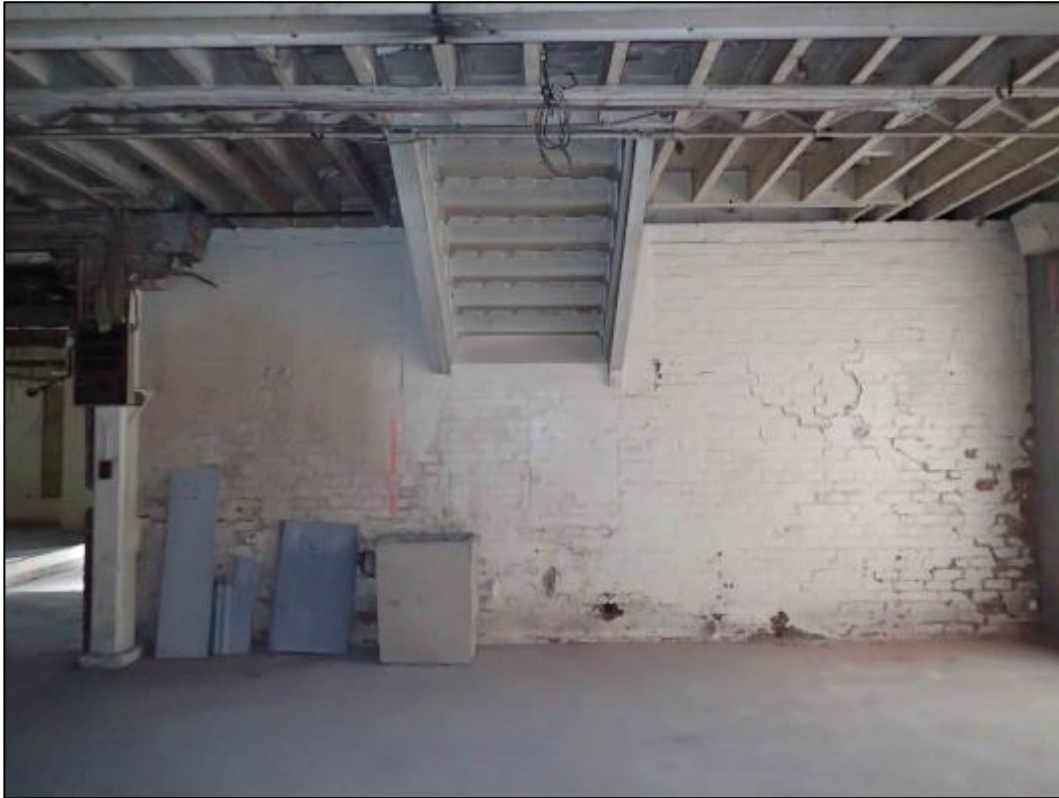
Figure 7-9. Photograph looking north at partition wall with two blocked in windows and the bottom of the stairwell leading from the partitioned area to the first floor.
