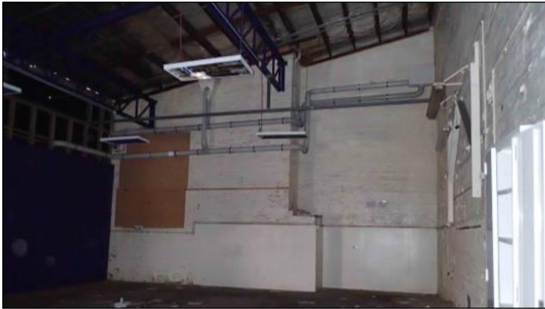
Figure 7-6 Distinct dog-legged wall of the former shared wall between the cellar and the mill (today the Dairy and Machine House Building and covered loading bay).
