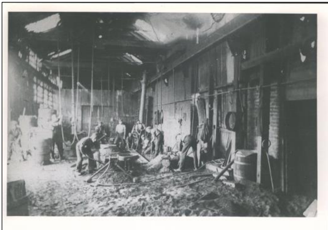
Figure 5-22. Photograph looking east of the iron moulding structure (Anon., n.d.-c).
