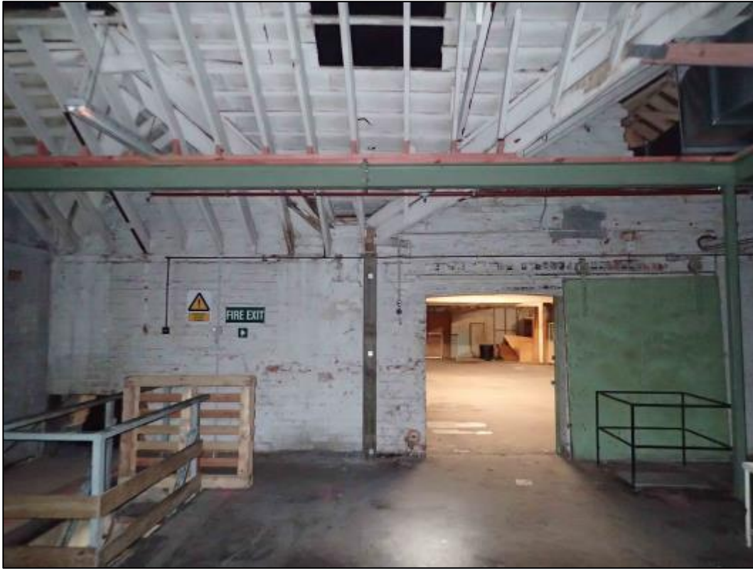
Figure 7-33 Photograph looking north at interior of Cadbury World building showing steel framing added to roof structure and steel columns. Note earlier skylights have been covered.
