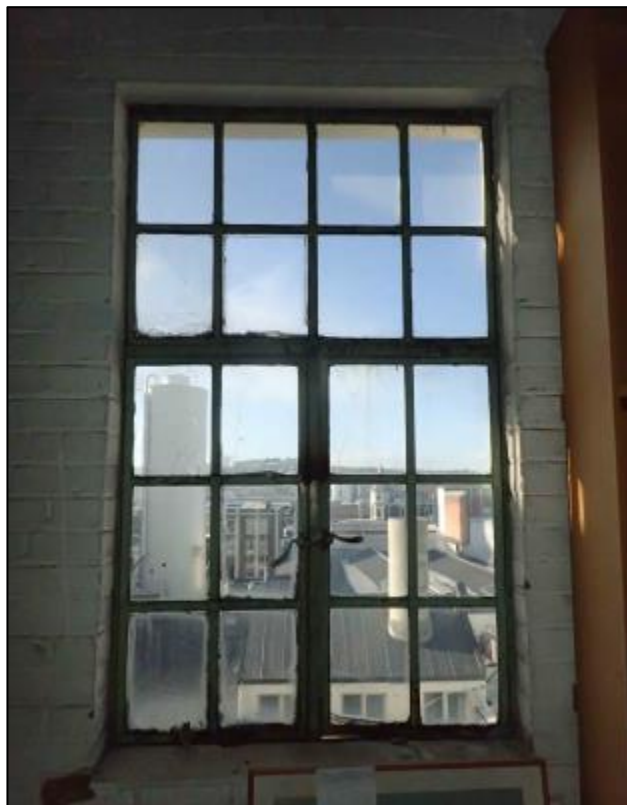
Figure 7-36 Photograph of windows on third floor looking east from the confectionery factory towards the rear of Cadbury World.
