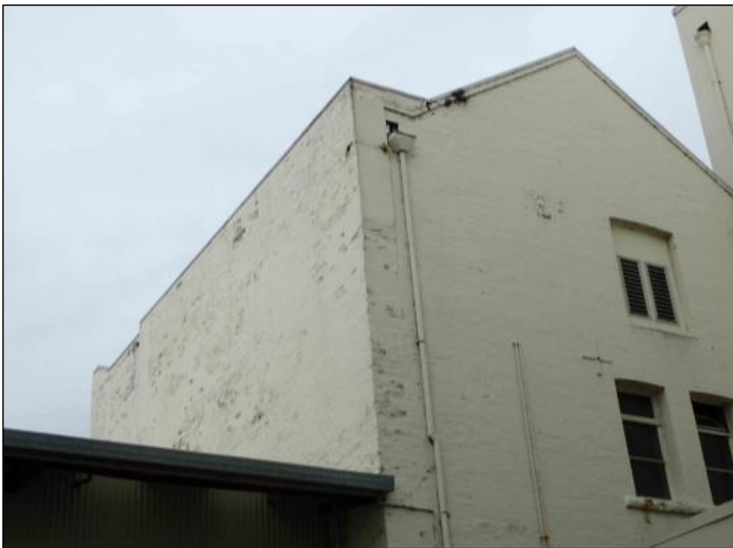
Figure 7-17 Photograph looking southwest at the eastern and northern wall of former smutters and kiln building. The upper floor was added sometime between 1892 and 1901, while the southern extension of 1901 is visible at the rear. There is one blocked in window on the eastern wall and another on the northern wall.
