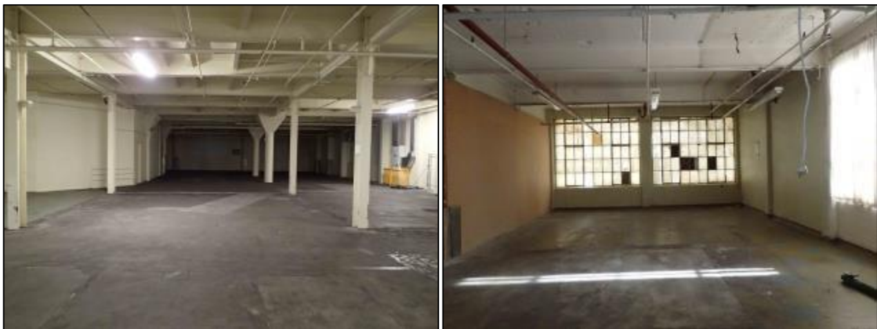
Figure 7-48 Photograph of the Chocolate Factory and Garage Building looking west at the former garage on the ground floor (left), and looking north at the former factory on the first floor (right).
