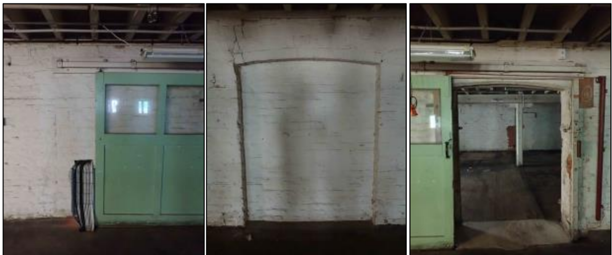
Figure 7-25 Photographs looking east at two blocked in doorways (top) either side of current doorway (bottom) to the eastern room of the former kiln and smutters room.
