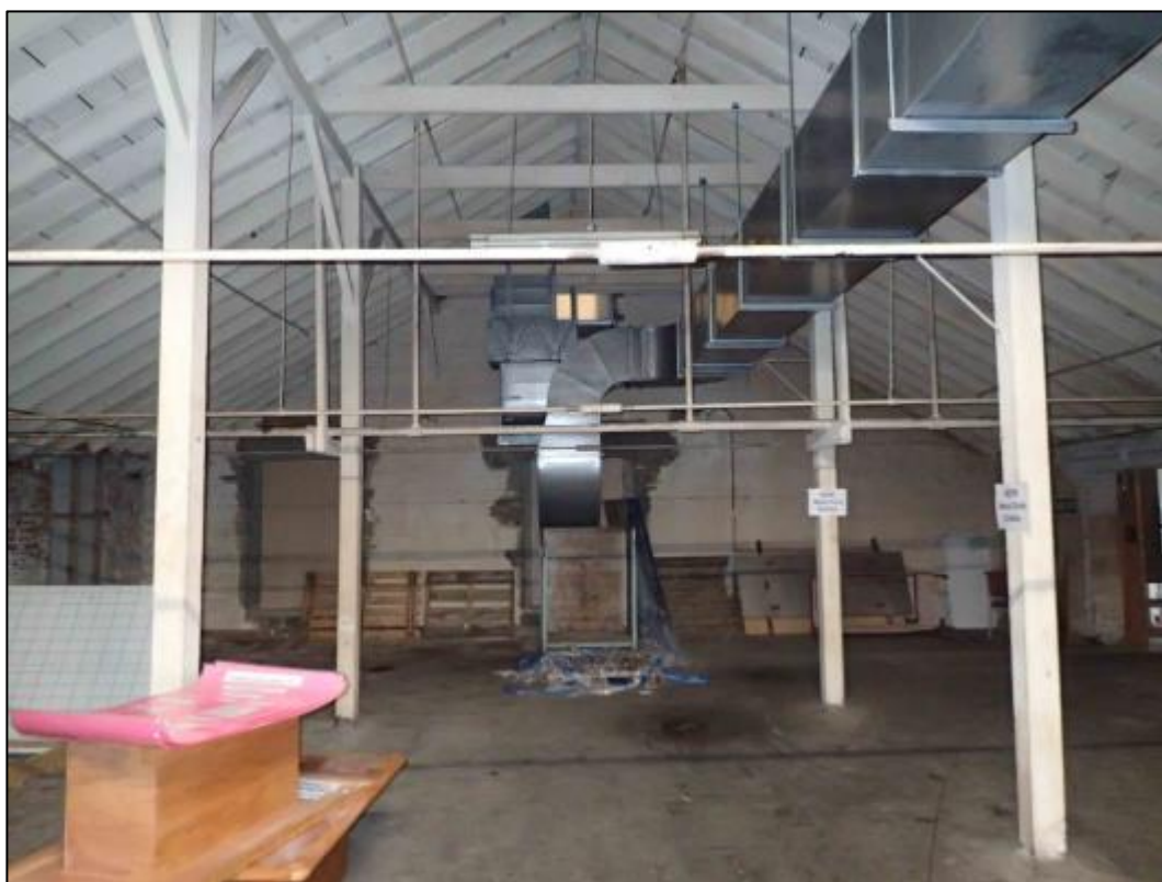
Figure 7-32 Photograph looking north at the roof framing and the windows of the second floor north wall of the Cadbury World building associated with the 1901-1915 storey addition. Prior to the 1915-1922 raising of the offices and shop building this would have been an exterior wall.
