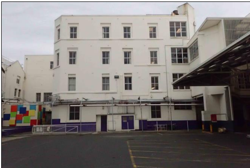
Figure 7-39. Photograph looking west at the rear of the Office Building (Block 2A).
