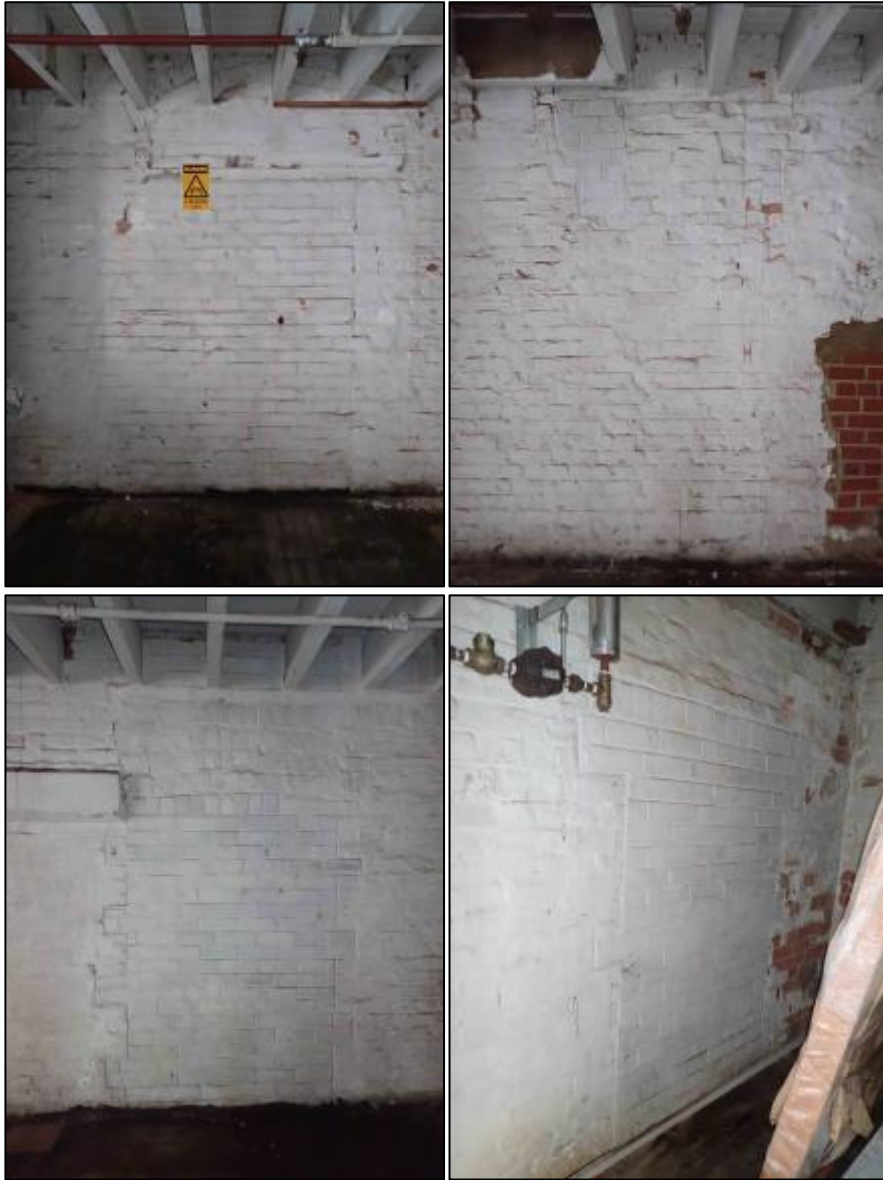
Figure 7-24 Blocked in doorways and windows in the former kiln building looking east (top right and left and bottom left) and northeast (bottom right).
