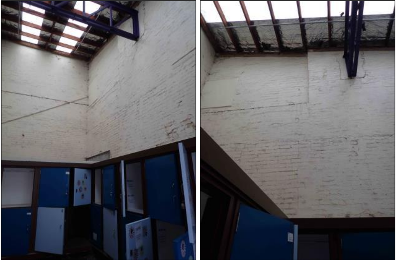
Figure 7-16. Photograph looking southwest (left) and west (right) at the eastern wall of the former kiln and northern wall of the former mill building. Note the jut into the wall is on the second storey. This may be associated with pre-1900 lean-to at the rear of the kiln and mill buildings
