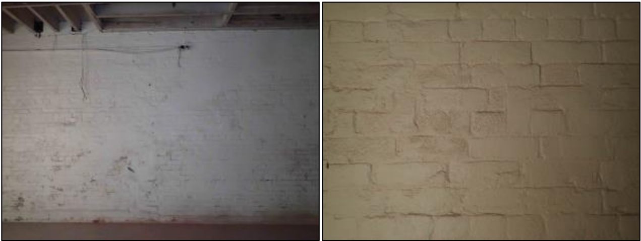
Figure 7-10 On the left is photograph looking south on ground floor of the Dairy and Machine House Building at location of first former staircase. A landing is visible half-way up. On the right is a photograph looking south on ground floor of the Dairy and Machine House Building at possible joist insertion points. These are at the same height as the first former staircase landing and possibly indicate there was a mezzanine floor at this height.
