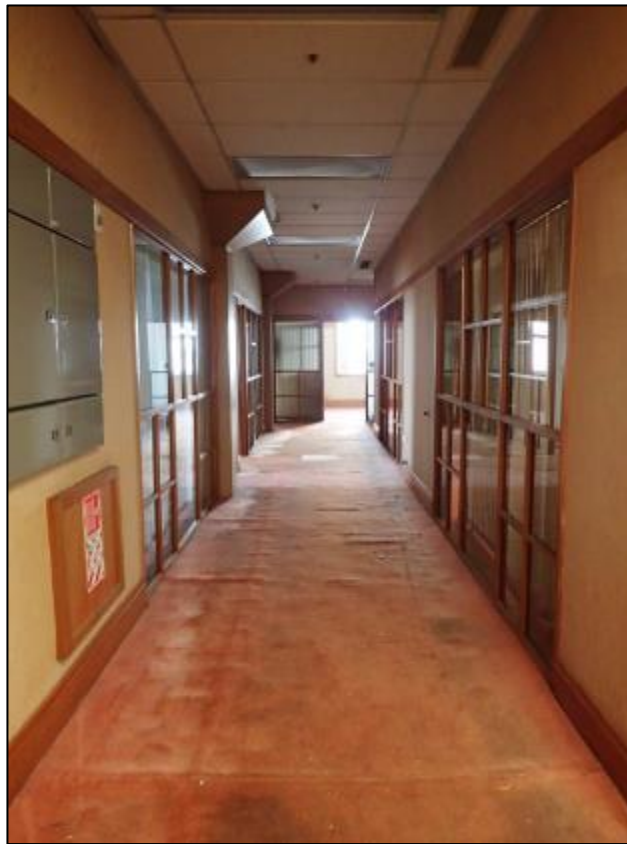
Figure 7-43 Photograph looking south at office portion of the Dairy and Machine House Building.
