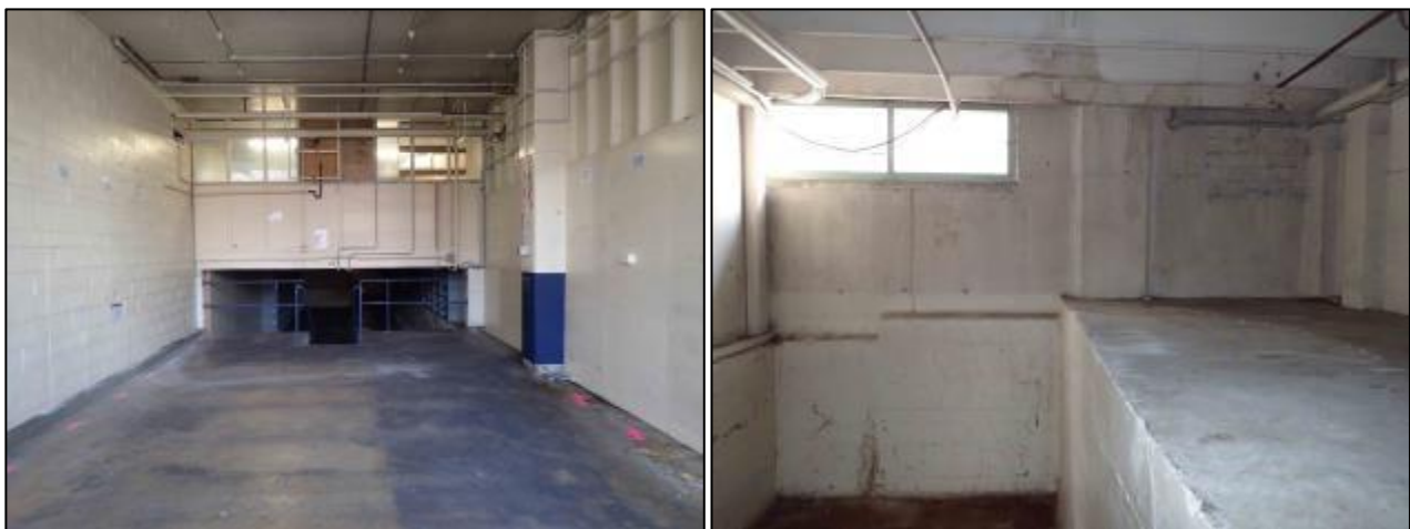
Figure 7-57 Photograph looking east into basement and Mezzanine from ground level (left) and at basement wall (right). Note the brick infill and the open window running up into the mezzanine level above.
