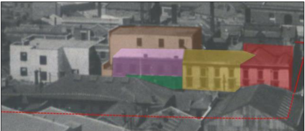
Figure 5-40 Circa 1922-1924 photograph showing buildings the alterations granary/malt floor and Kiln buildings (Frank Duncan and Co. c. 1922-1924). The original 1868 granary granary/malt floor and kiln buildings are not visible; however, subsequent alterations are highlighted red for Phase one (1901), yellow for Phase three (1901-1915), green for Phase four (1915), pink for Phase five (1915-1922), and brown for Phase six (1922).
