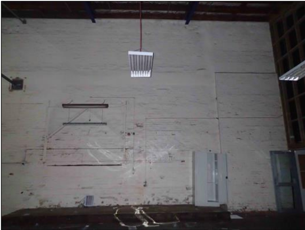
Figure 7-18 Photograph looking north at wall between Dairy and Machine House Building and the Cadbury World and Office Building. Note that the eastern end of the building has been raised.
