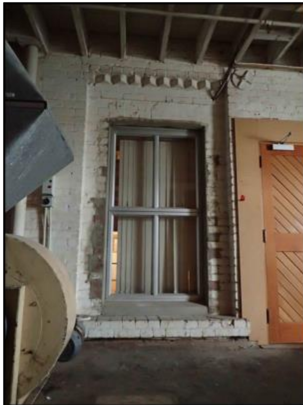
Figure 7-41. Photograph looking north at a former exterior window of the Office Building (Block 2A) associated with the 1915 western addition to the building. This photograph is taken from the later 1922-1927 addition at the rear of the Cadbury World building on the first floor.
