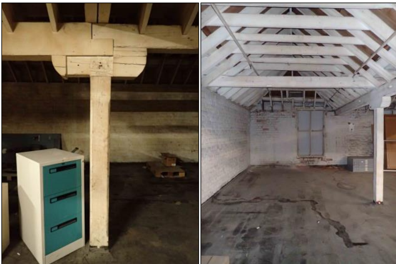
Figure 7-31 Photograph looking south (left) at column in the second floor of the Cadbury World building with the 1901 southern extension behind and photograph looking west (right) at roof structure of the southern extension.
