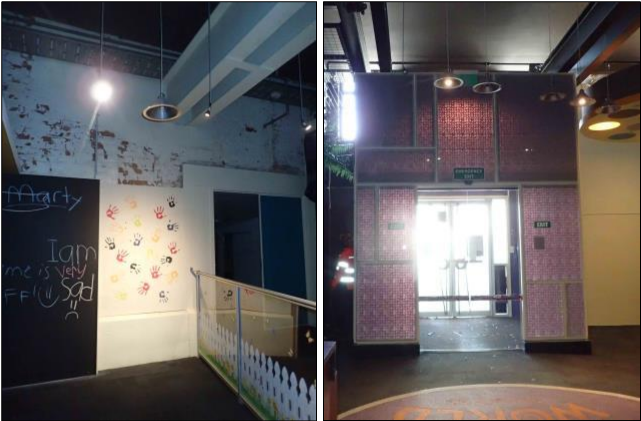
Figure 7-21. Photographs looking east (left) and west (right) on the ground floor of the Cadbury World building showing steel beams. Note the windows of the mezzanine floor above the door in the photograph on the left.
