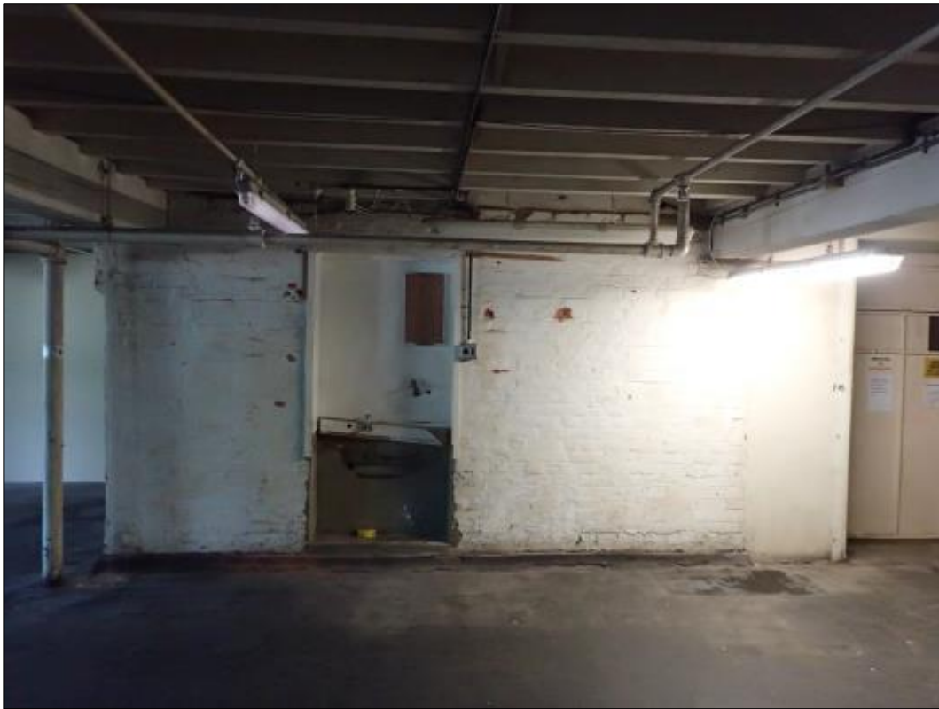
Figure 7-26. Photograph looking north at original kiln wall. There is a stone arch visible above the tap area to the east is a diagonal line rising up.
