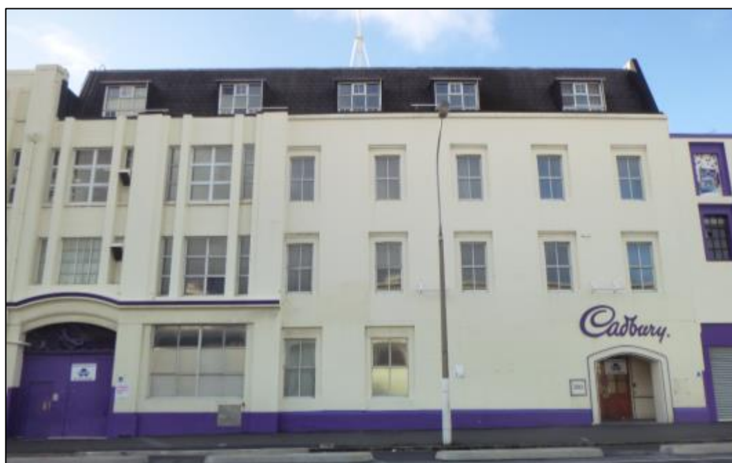
Figure 7-38. Photograph looking east at the Cumberland Street façade of the Office Building.
