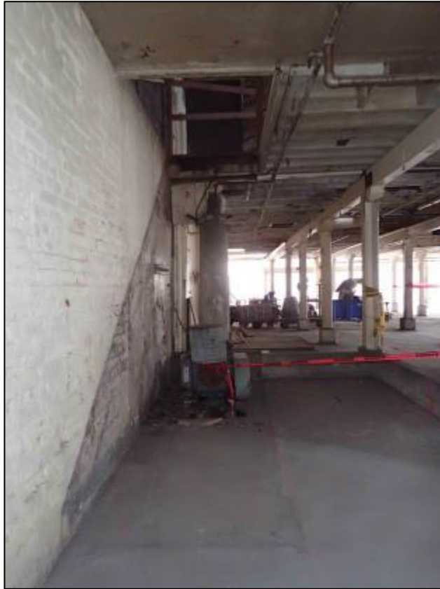
Figure 7-11 Photograph looking west on ground floor of the Dairy and Machine House Building at location of second former staircase visible in 1959 plans.
