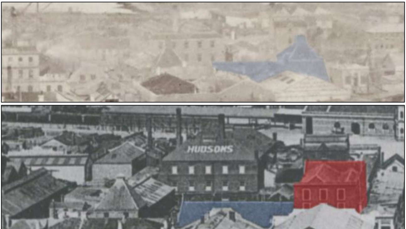
Figure 5-36. April 1901 photograph (top) showing the granary/malt floor building (highlighted blue) prior to the Phase one alterations (Muir and Moodie Studio, 1901). Part of a c. 1905 panoramic view (bottom) showing the 1901 Phase one southern and upper storey extension to the granary/malt floor and kiln buildings (highlighted red) (W Beattie & Co., n.d.). The 1868 central and northern extent of the granary/malt floor building is also visible to the north unaltered (blue). Note the biscuit factory in the background. The top photograph shows the 1901 factory, while the bottom photograph shows the almost identical 1902 building with “Hudsons” advertised on the roof.
