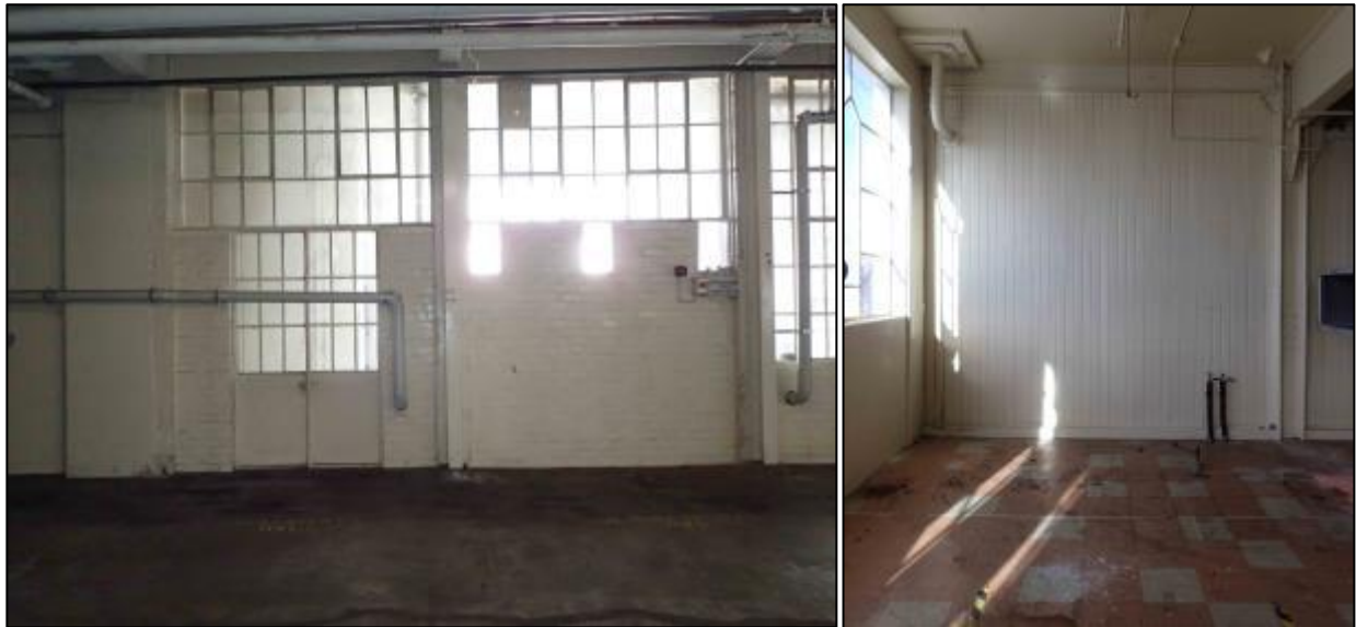
Figure 7-52 Photograph looking south at bricked in wall section in the Chocolate and Biscuit Factory (Block 3B-C) on the ground floor (left) and looking south at tongue and groove wall lining on the second floor.
