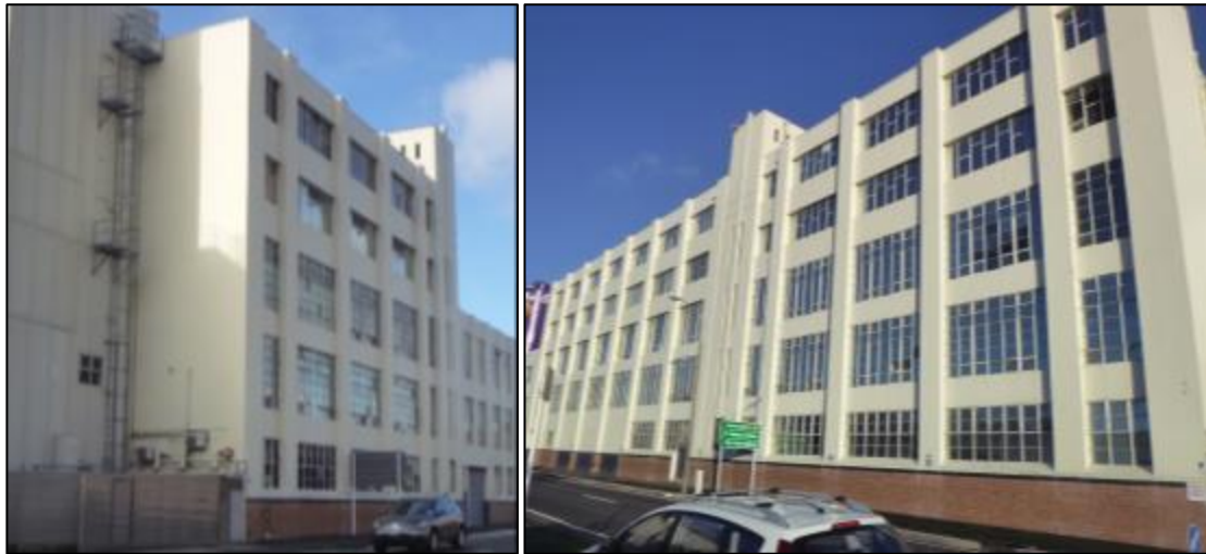
Figure 7-60 Cumberland Street (left) and Castle Street (right) façades of the biscuit and dispatch building.
