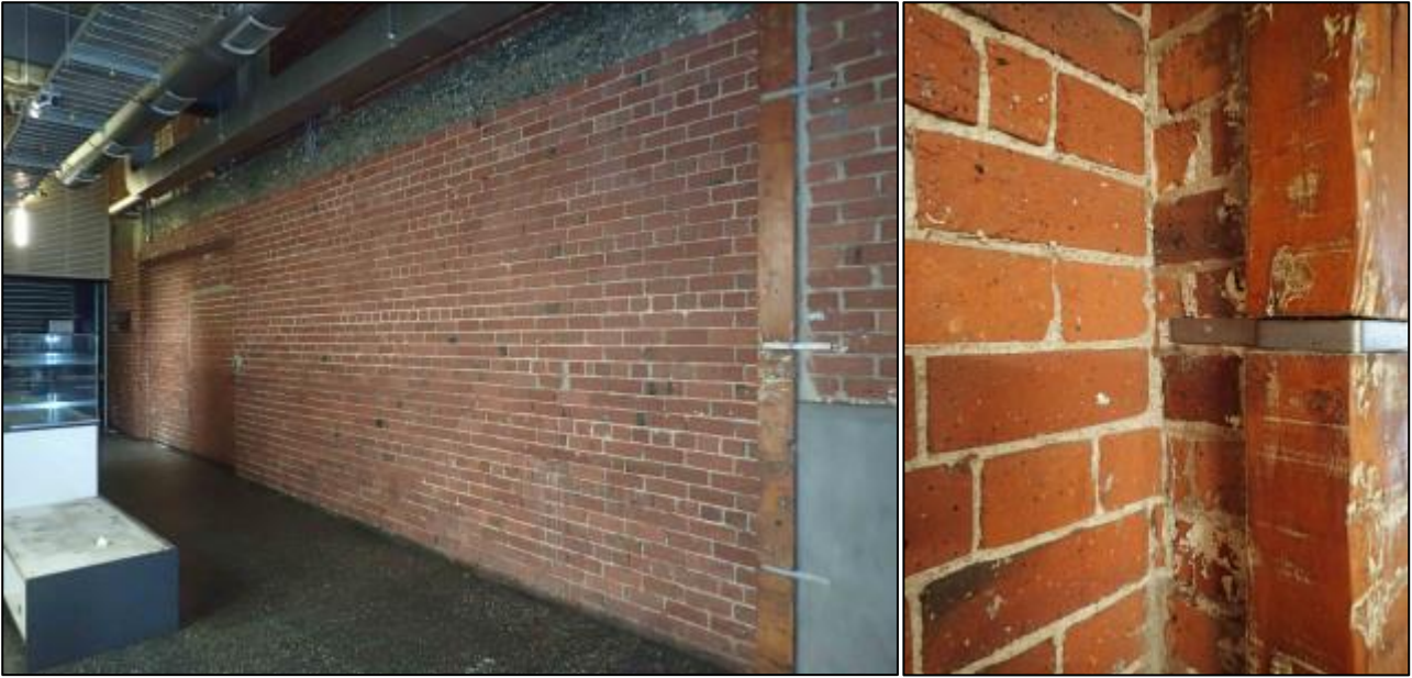
Figure 7-19. Photographs looking northwest (left) at southern internal partition wall on the ground floor of the Cadbury World Building and northeast (right) at the abutment of the same wall to an earlier external wall to the west. The wall was likely present from 1922. Note the blocked-in doorway on the northern internal wall.
