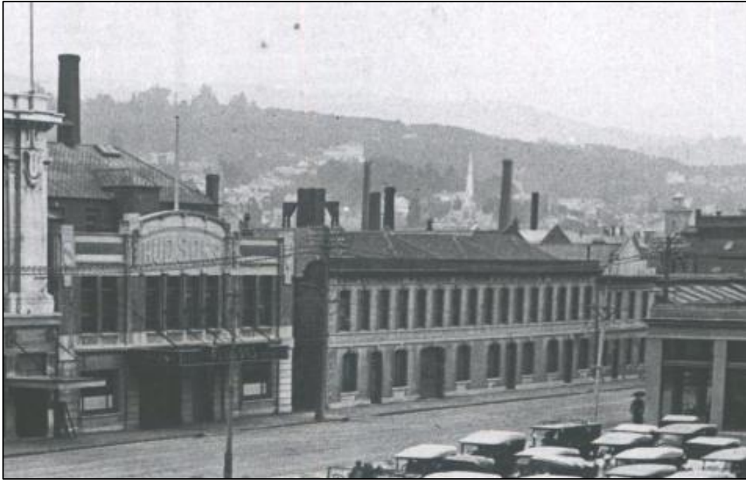
Figure 5-52. 1922 façade of the Dairy and Office Building and Biscuit factory in Town Section 72 and 73 abutting the earlier brick building in Section 71 (Anon., 1922).
