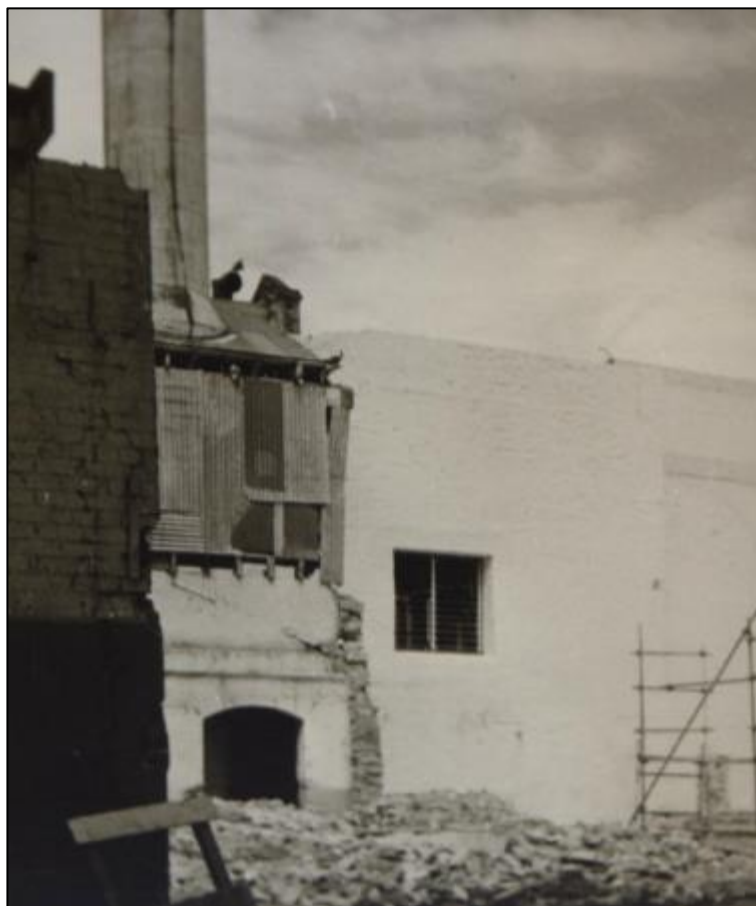
Figure 5-61. Likely early 1960s photo showing the demolition of the old boiler house. The rear wall of the machine or former engine house is visible to the left and the cellar building to the right (Figure 13 in Farminer, 2014). The north return wall of the mill or still room building is visible in the centre of the photo.
