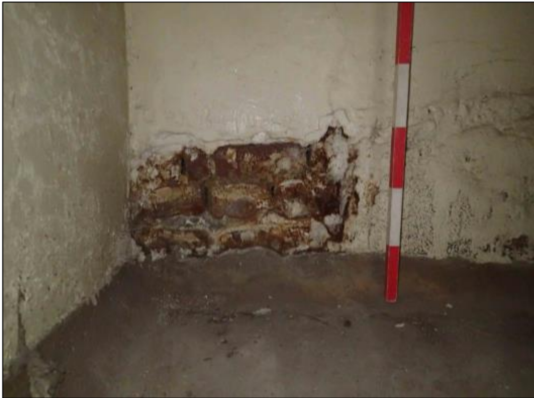
Figure 7-13 Photograph looking west at the plastered brick wall of ground floor in the machine house building.
