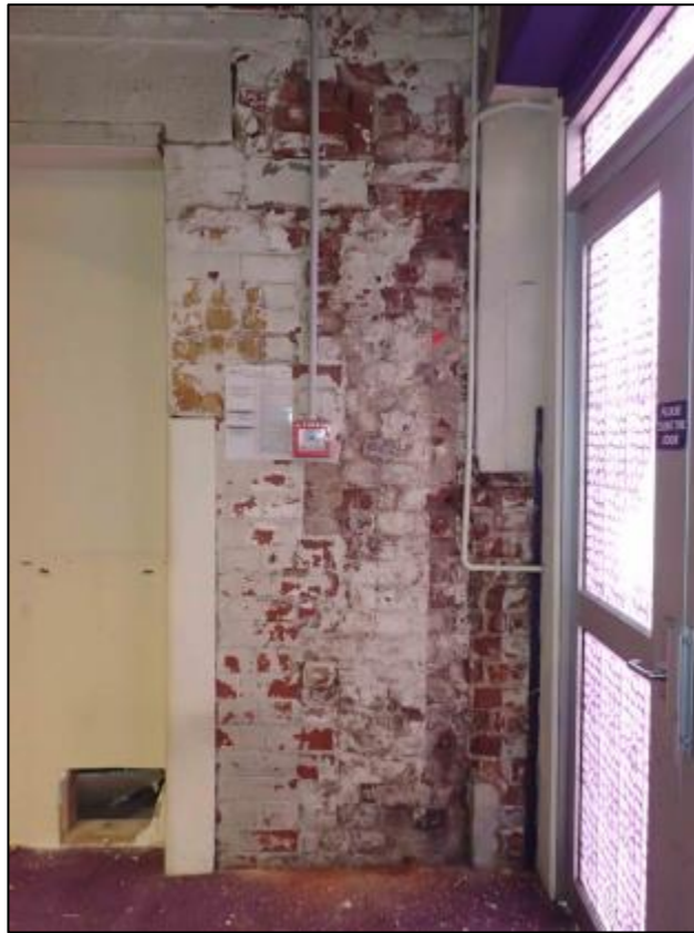
Figure 7-23. Detail photograph of interior wall of Cadbury World building that would have originally form the north exterior wall of the pre-1900 kiln showing a possible ground floor partition wall and joist insertion point for the original mezzanine level.
