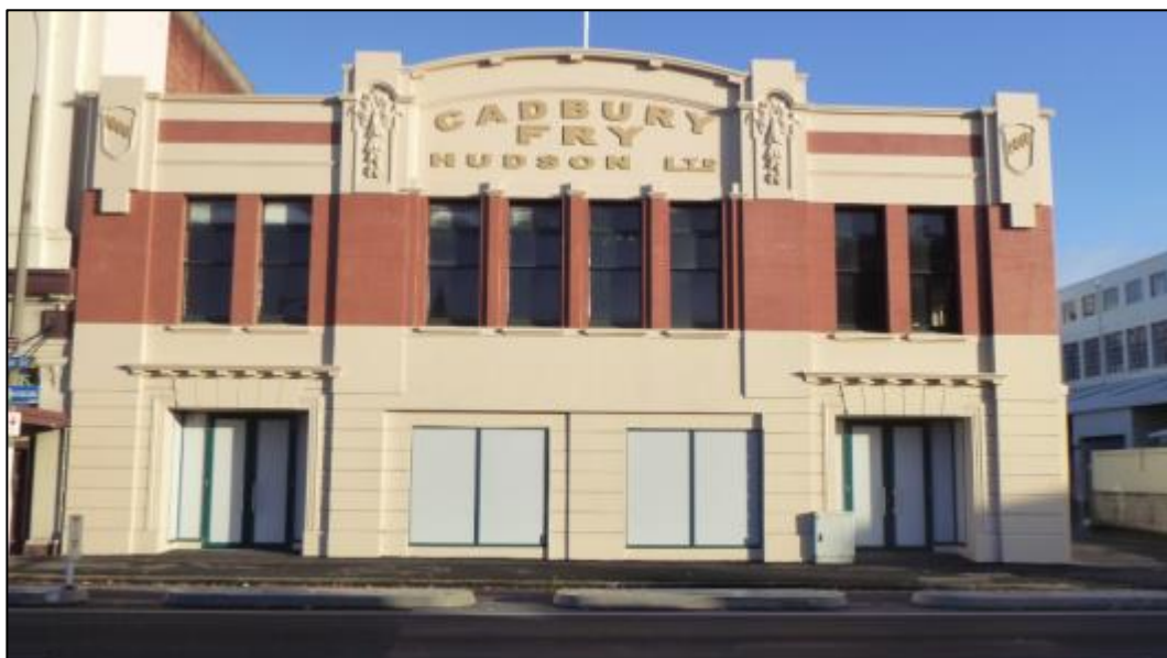
Figure 7-3 Photograph looking west at the Castle Street façade of the Dairy and Machine House Building.
