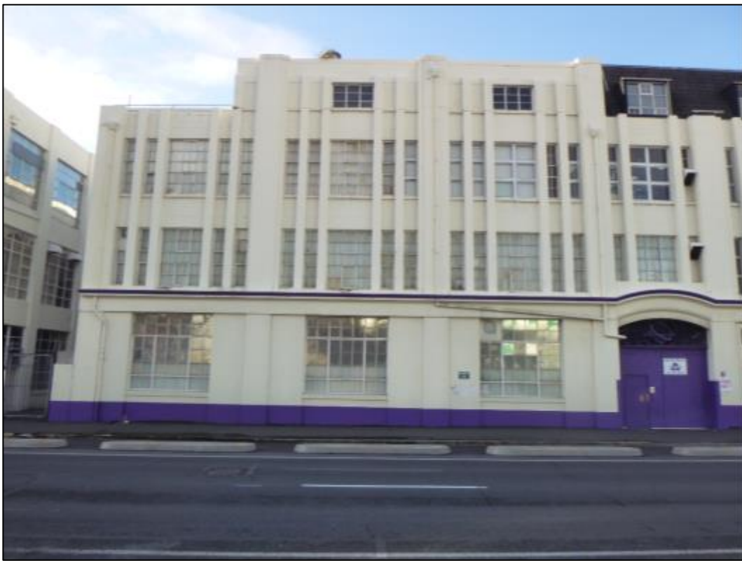
Figure 7-47 Photograph looking east at the Cumberland Street façade of the chocolate factory building.
