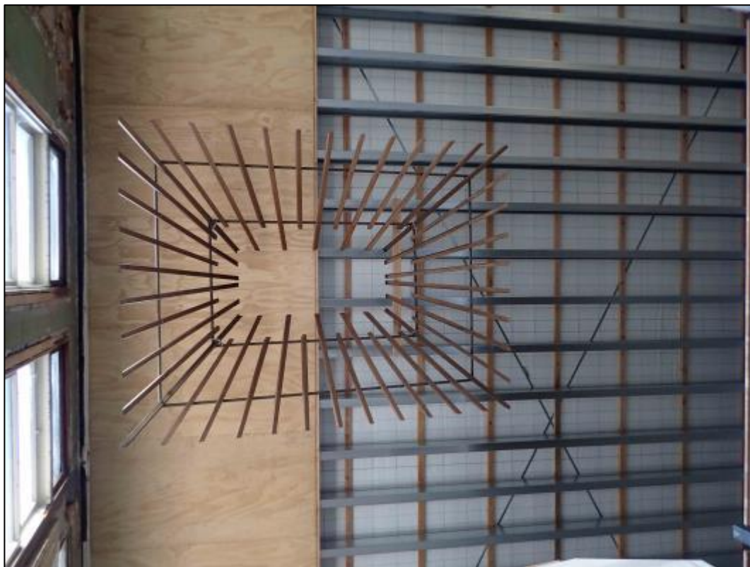
Figure 7-8. Suspended screen visible in the 1966 plans above the stairwell to the second floor.
