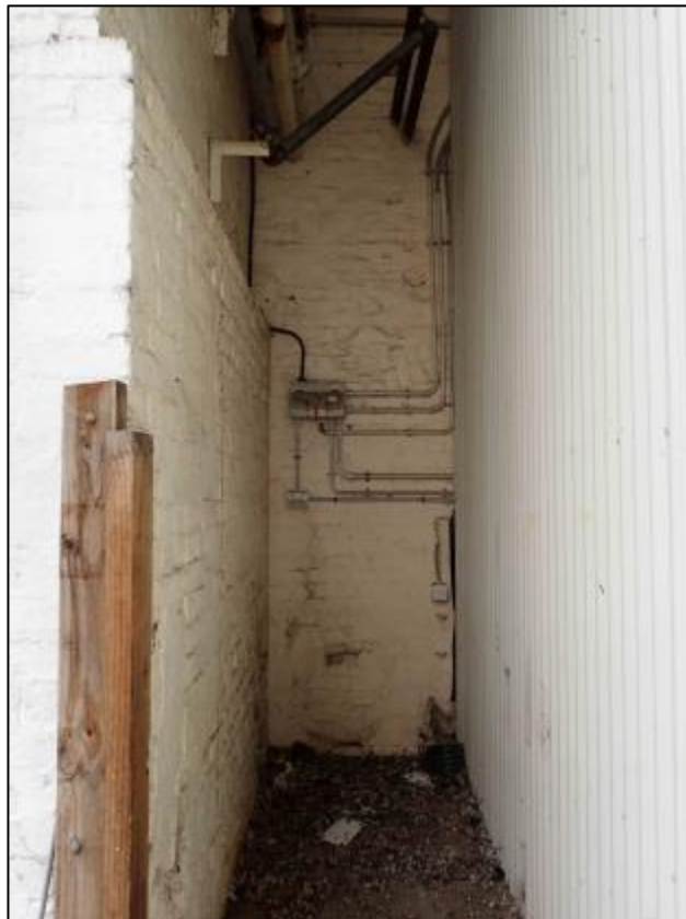
Figure 7-7 Photograph looking east at the former doorway or window arch located on the shared wall between what was once the cellar and mill
