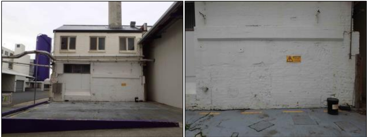
Figure 7-5. Photograph looking east at the western wall of the machine house showing the blocked-in windows. A close-up photograph is shown on the right.
