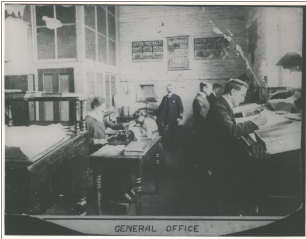
Figure 5-11 The interior of the general A & T Burt Offices in the late nineteenth or early twentieth century (Anon., n.d.-b)
