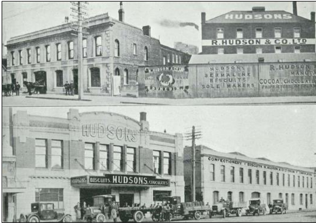
Figure 5-49. Top: 1900s photograph of the Biscuit factory in Town Sections 72 and 73 to the left of the offices in Town Section 74. Bottom: altered façade of the Hudson building in 1928 (Figure 12 in Brooks & Jacombs, 2010).
