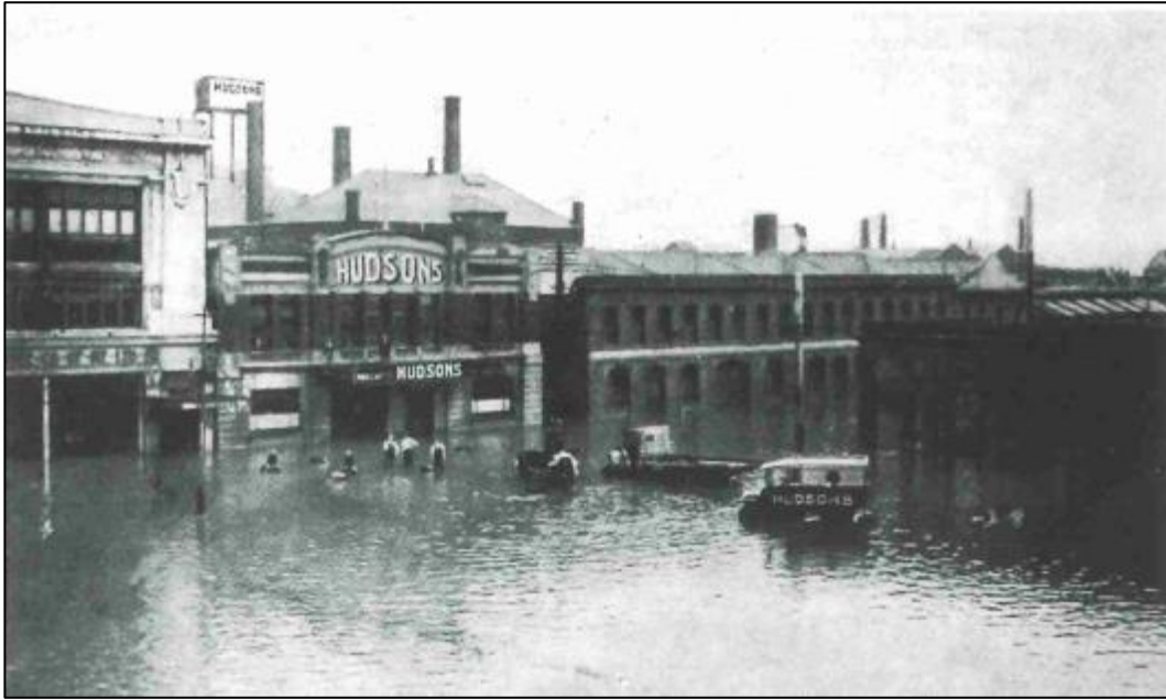
Figure 5-84 Photograph looking the Castle Street façade during the 1923 flood.
