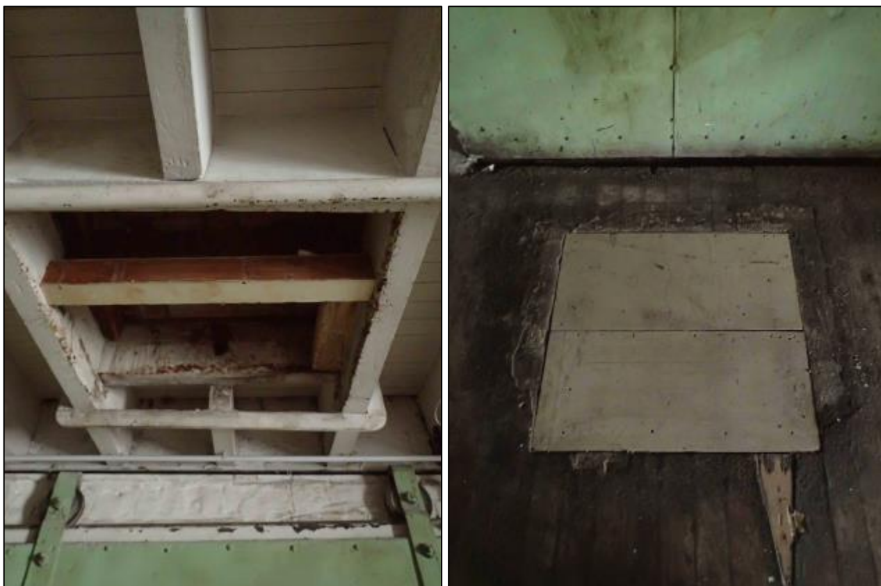
Figure 7-28 Photographs showing location of blocked in roof (left) and floor (right) of possible former chimney in former kiln building.
