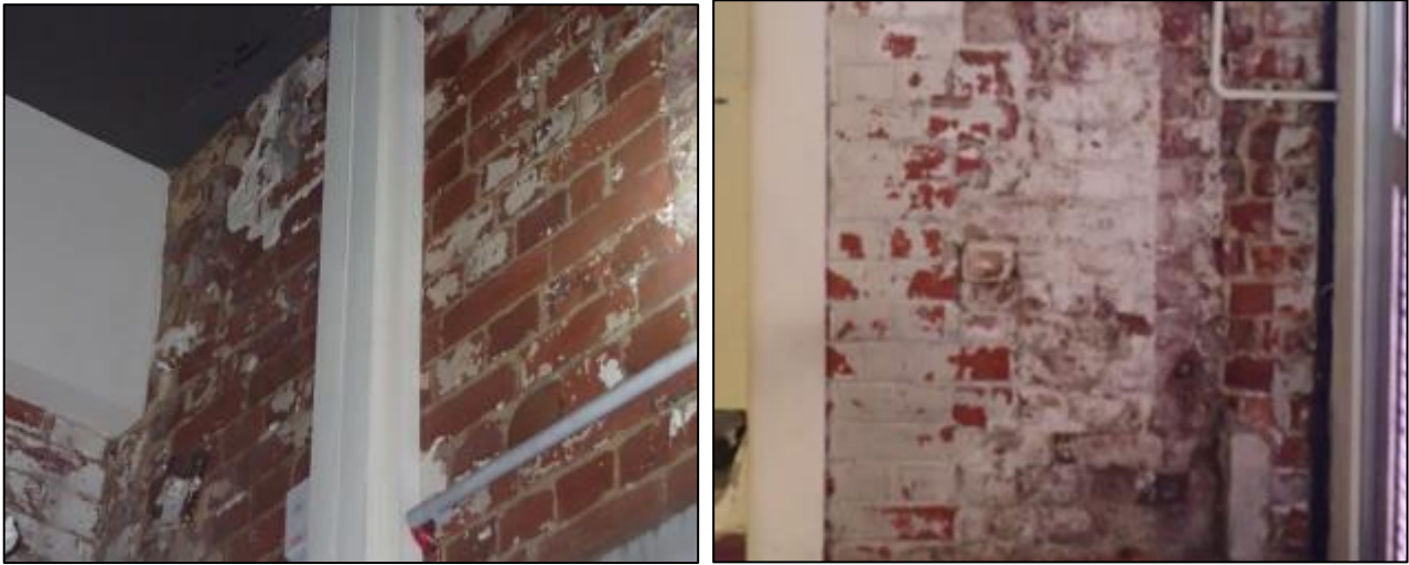
Figure 12-1 Examples of exposed and partially exposed brick from the Cadbury World building that might be salvaged and reused elsewhere in the hospital development.
