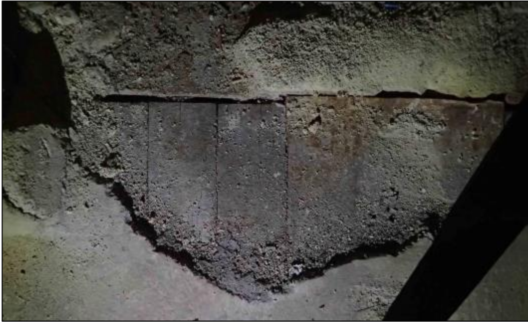
Figure 7-35 Photograph of tongue and grove timber underneath concrete of the floor in the second floor of the Cadbury World building.
