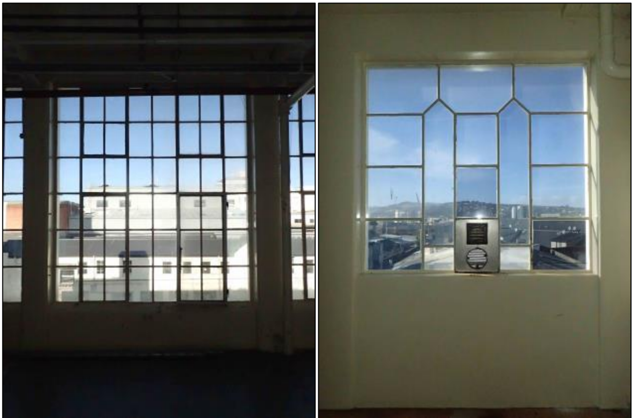
Figure 7-53 Photograph looking south (left) and east (right) at variant multi-pane window on the second floor of the Chocolate and Biscuit Factory building (Block 3B-C) second floor.
