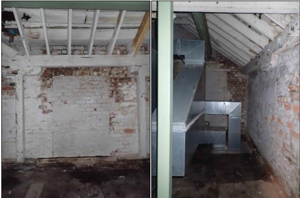
Figure 7-34 Photograph looking east (left) at a blocked in door way and north (right) at a blocked in window in the second floor of the Cadbury World building the most easterly room of the former kiln building.
