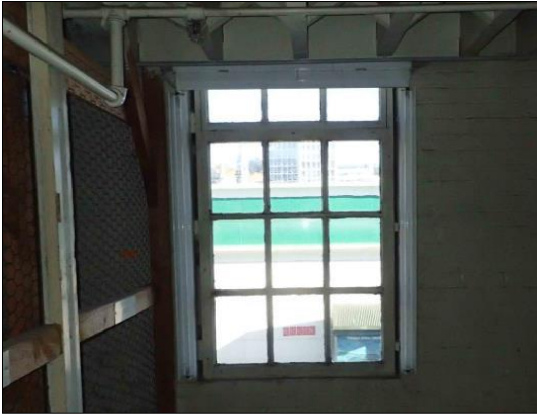
Figure 7-30 Photograph looking west at multiple fixed pane window on the first floor of Cadbury World. All windows along the western wall are the same suggesting they were added and older windows replaced to match the 1902 and 1915 windows when the central portion of the granary and malt floor was added or that the new windows were added to match the earlier 1889 to 1901 style of windows.
