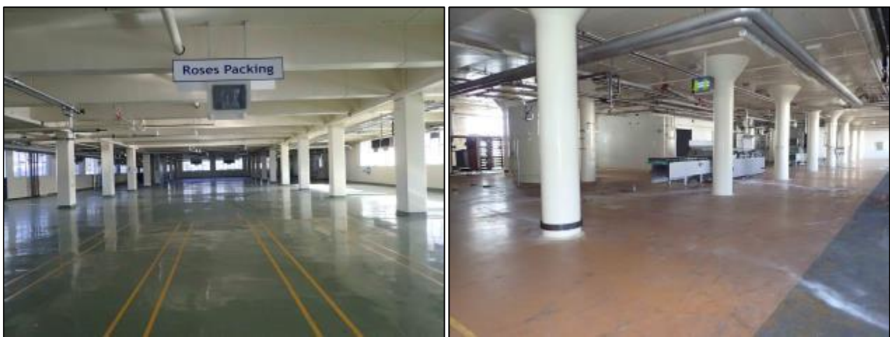
Figure 7-61 Photograph of the biscuit and dispatch building (Block 5C) on the third floor looking west (left) and on the first floor looking northwest (right).
