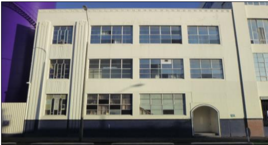
Figure 7-50 Photograph looking west at the Castle Street façade of the Chocolate and Biscuit Factory building.
