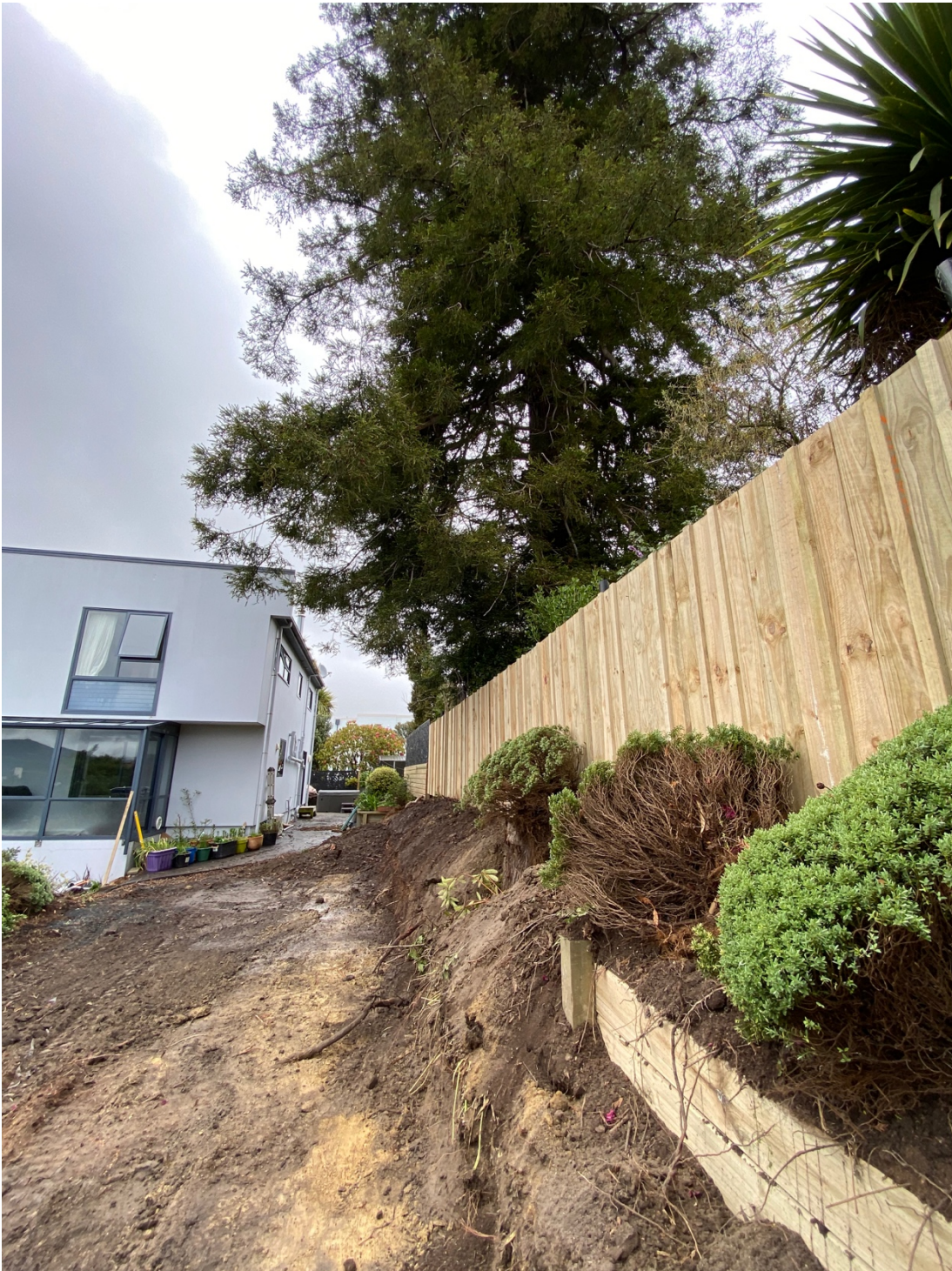
Image three: Image of T026 taken from inside 17C Melrose Street, showing the extent of the soil removal, proximity of the 'cut' to the boundary line, the clay-loam type soil and the complete absence of roots in the soil beyond the cut face.
