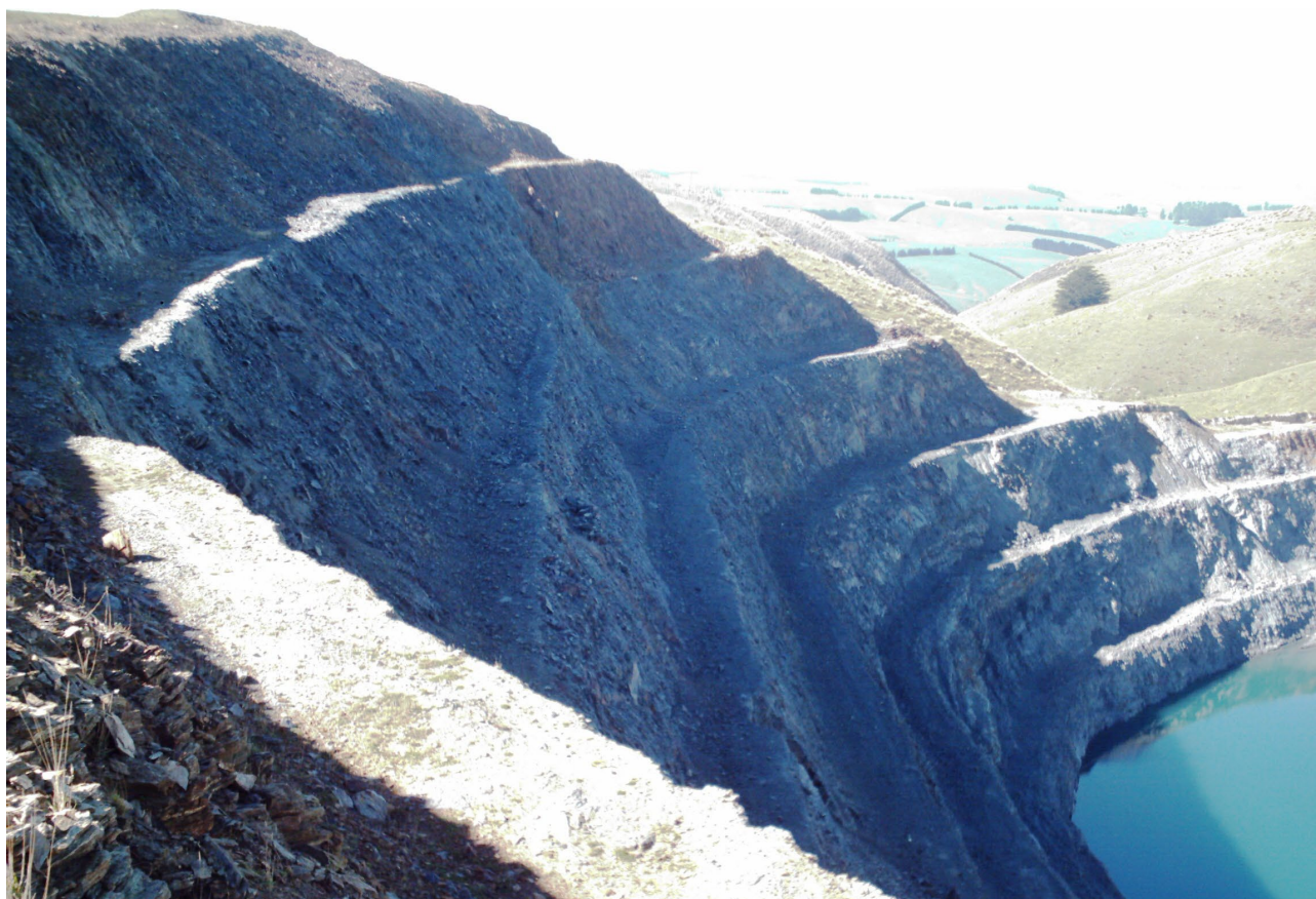
Photo 9: January 2009 - east wall taken from crest facing south. Berms are relatively clean.
