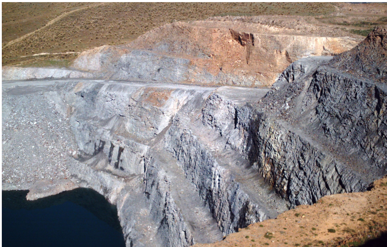
Photo 10: January 2009 – north wall. Photo taken from crest looking west. Pre-split 75° batters. Note joint bound wedges.
