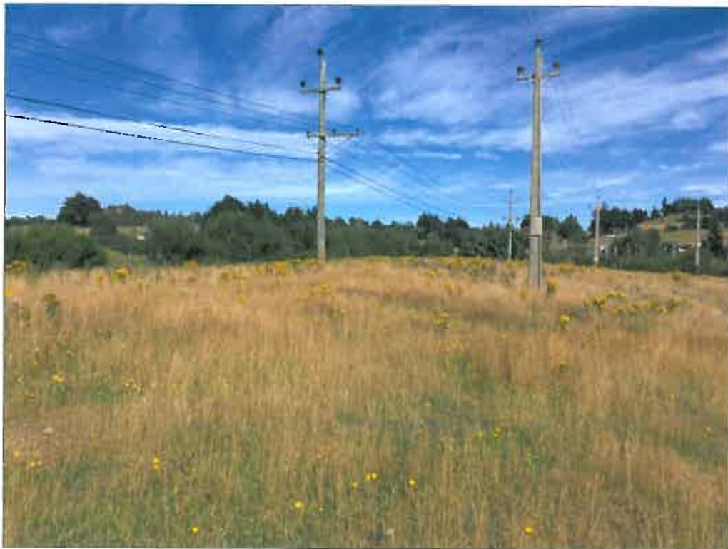
Photo U – Looking west from within the site (standing beneath the existing overhead transmission lines).
