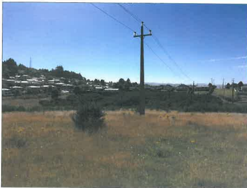
Photo Q – Looking east from within the site (standing beneath the existing overhead transmission lines).
