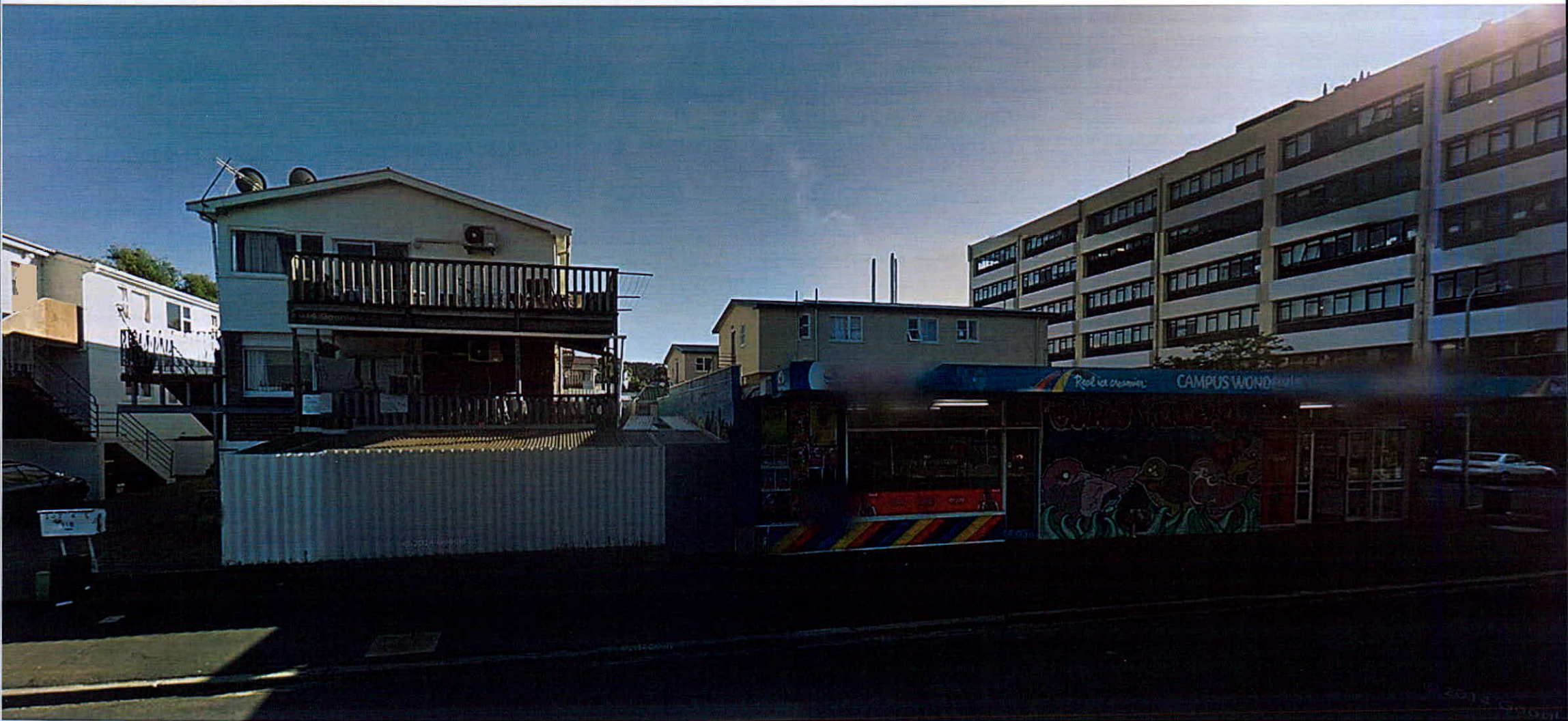
VIEW OF EXISTING BUILDINGS AT 118 and 138 UNION STREET EAST
