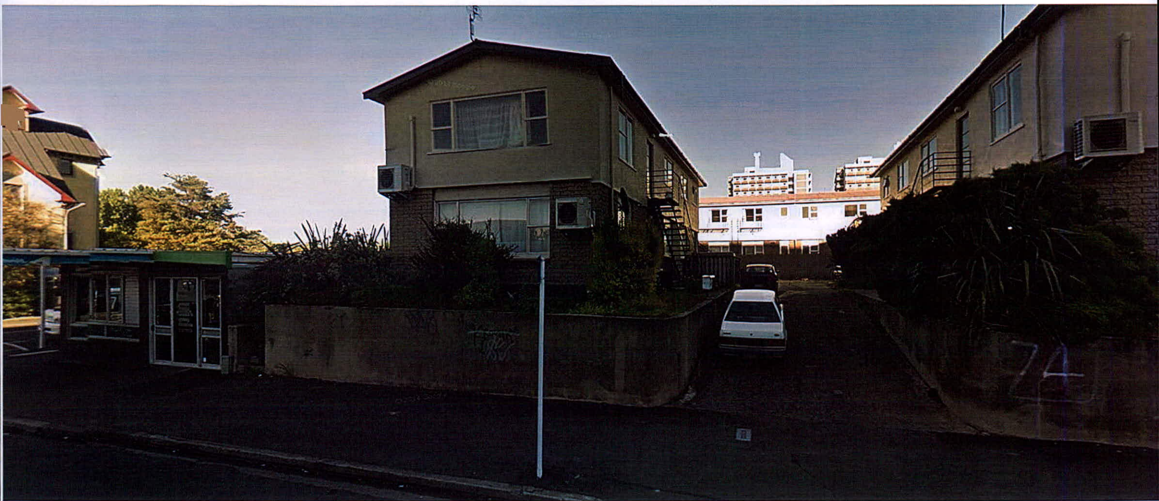
VIEW OF EXISTING BUILDINGS AT 74 FORTH STREET AND 138 UNION STREET EAST
