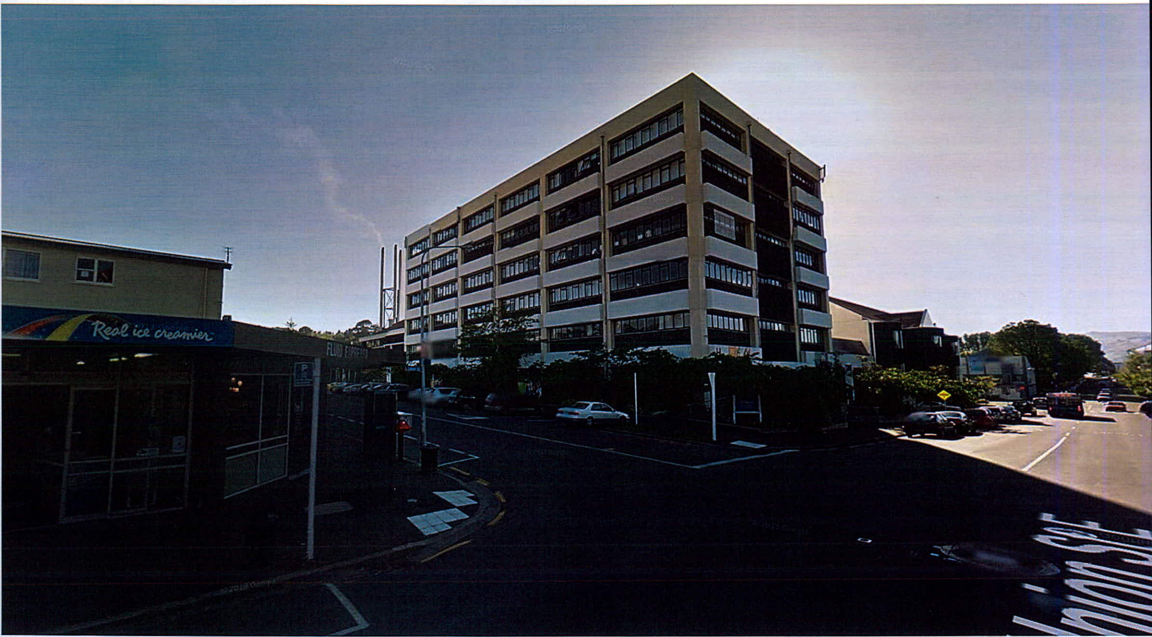
VIEW OF EXISTING BUILDINGS AT 138 UNION STREET EAST AND 95 FORTH STREET
