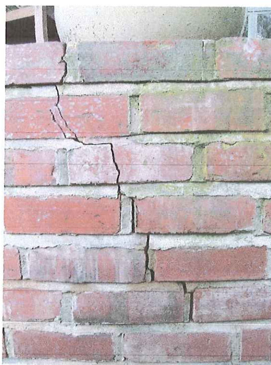
Photo 5A & 5B. Crack at location 4 in photo 1.
