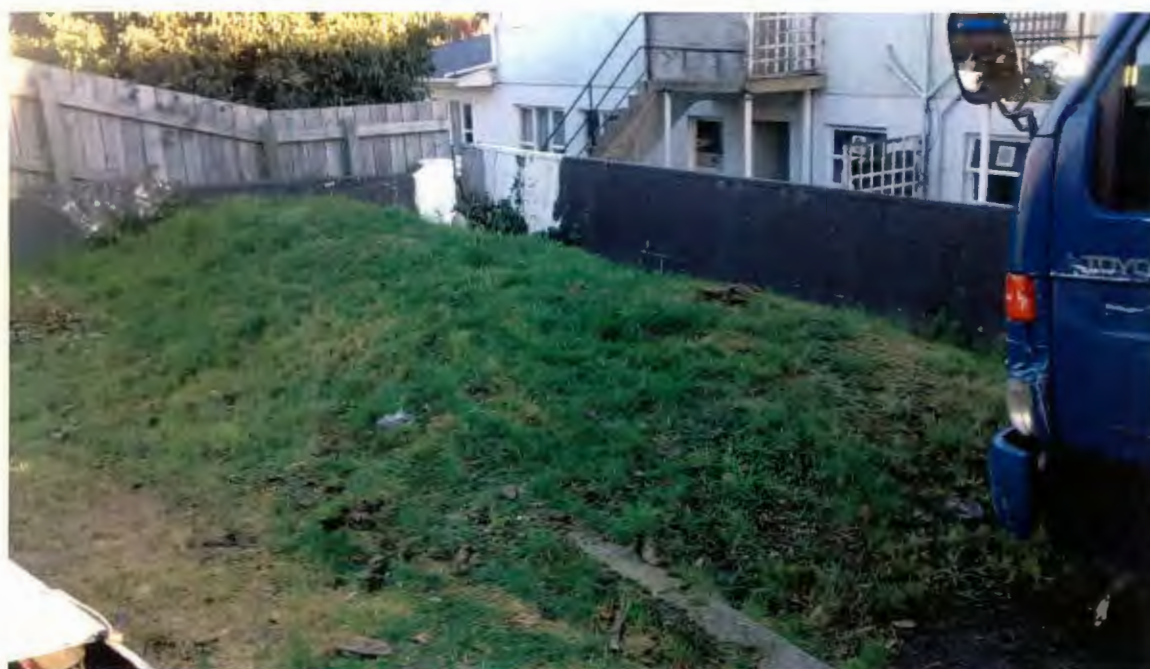
Figure 7. South-western boundary of the site, showing the drop to the west (9 June 2017).
