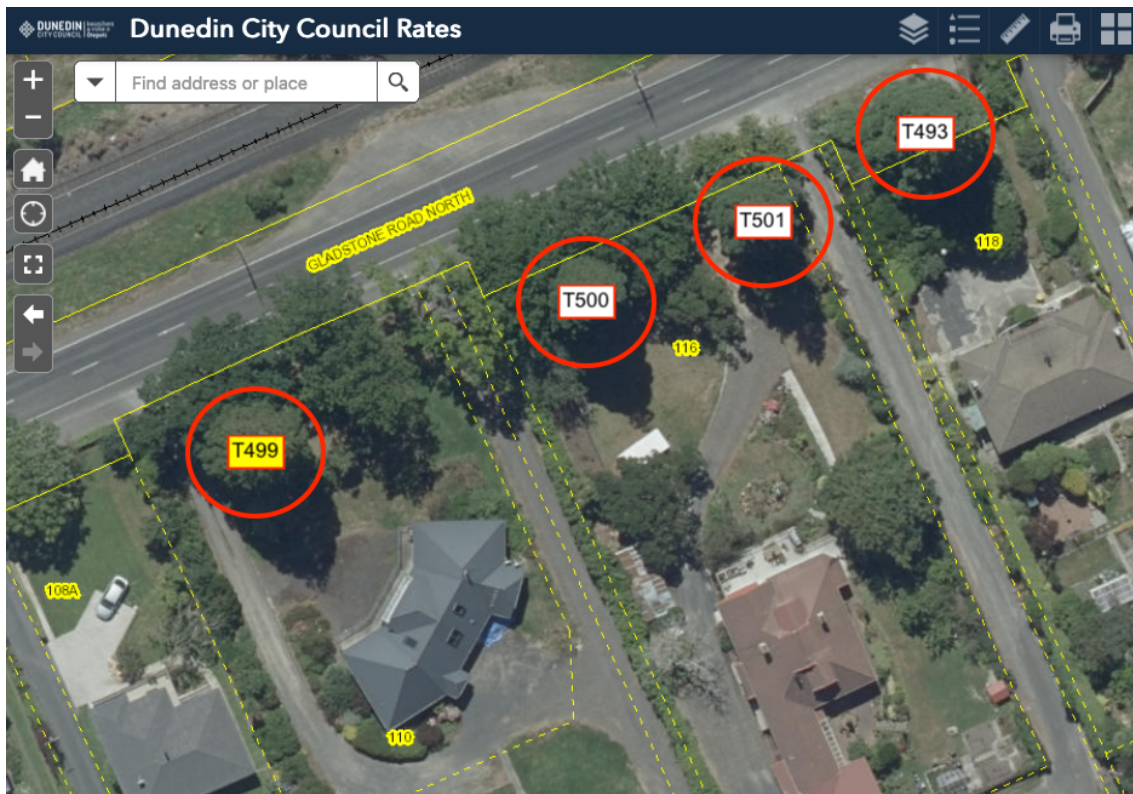
Image one: Image showing the row of 4 DCC Scheduled Wellingtonia trees on Gladstone Road North
